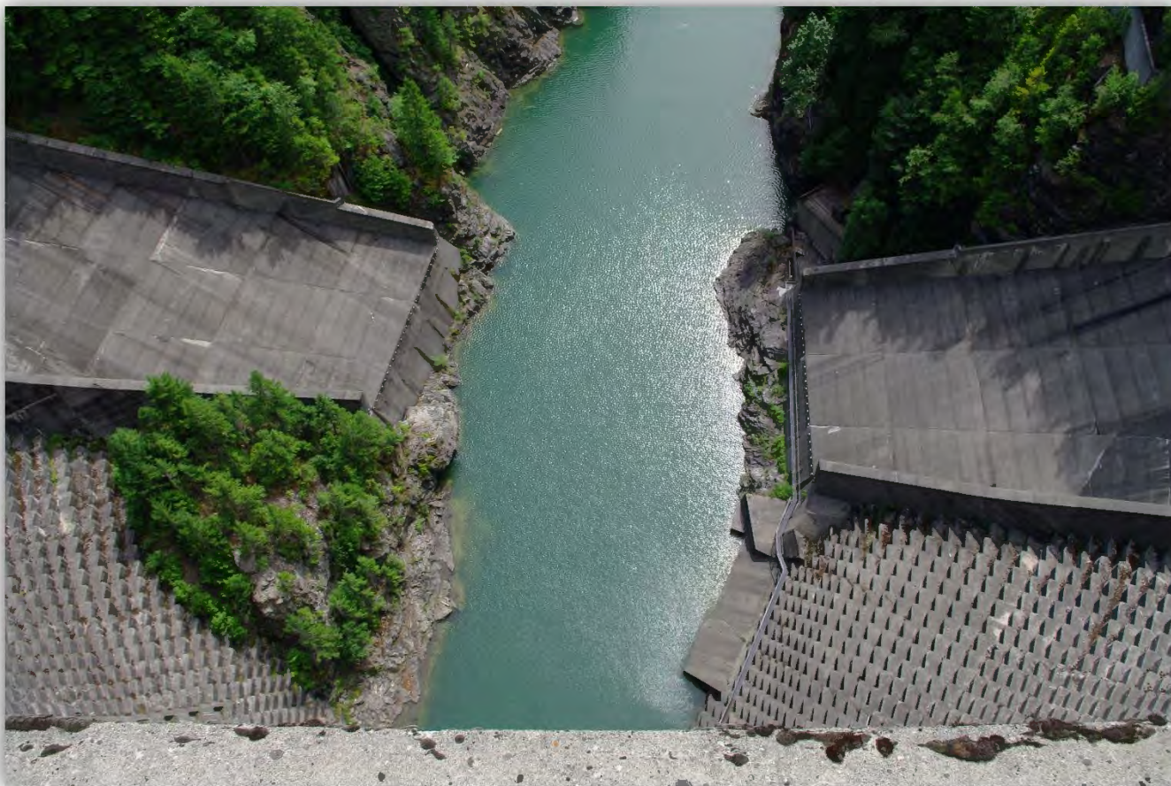
Looking down Ross Dam – June 2014 NPS Photo – A. Braaten
