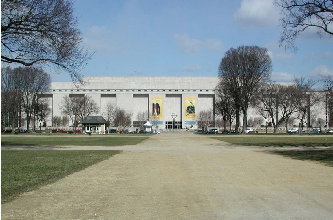
North-south Mall walks are aligned with the Washington street grid. The walk running between the National Museum of American History and the Department of Agriculture follows the route of 13 th Street. (CLP file “NMAH façade on axis clr” Feb. 18 2005)
