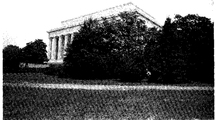
Figure 68- Existing west side foundation plantings, July 23, 1996. LINC 10-17.
