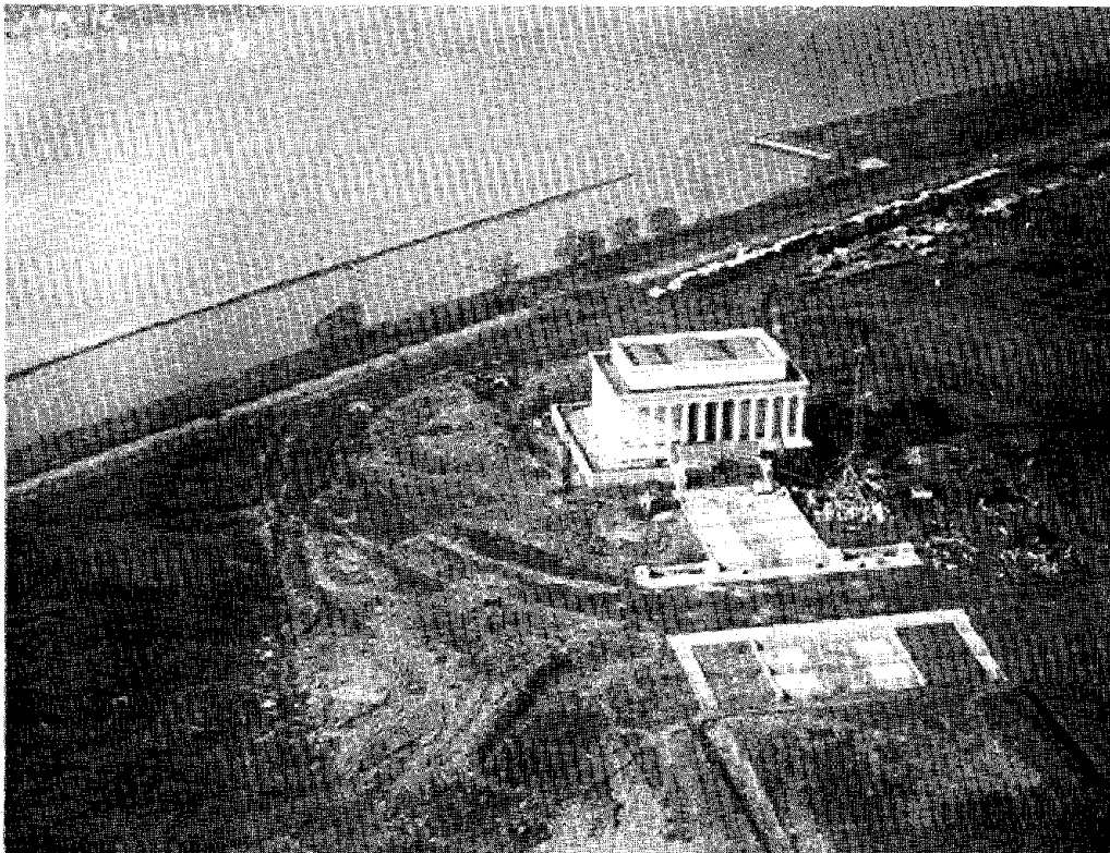
Figure 3 - Construction of approachway, Dec. 12, 1918. U.S. Navy photo. MRC 1-58.
