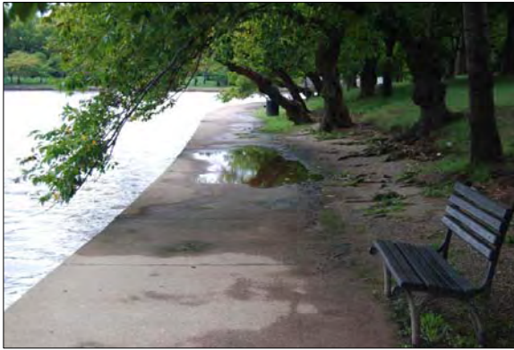
The walkway around the Tidal Basin is frequently flooded by high water.
