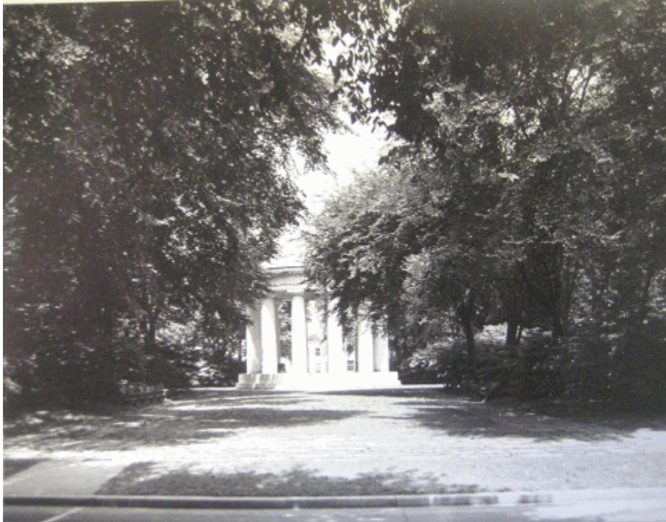
Figure 18. A view of the DC War Memorial looking north from Independence Avenue in July, 1946 shows the impact of the temporary World War II buildings on the landscape of the site, including views (NAMA files).
