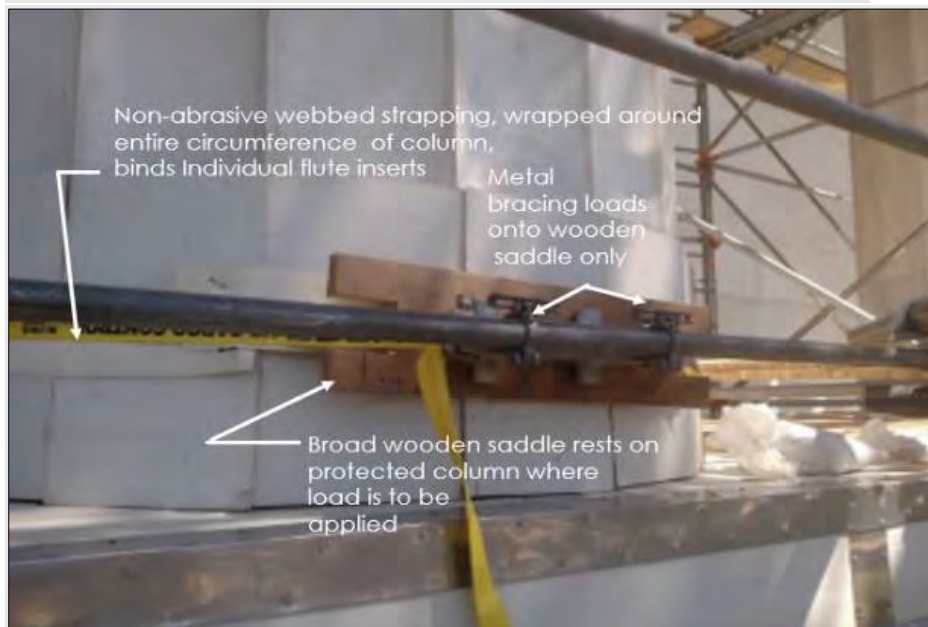
FIGURE 47. EXAMPLE OF COLUMN PROTECTION HIGHLIGHTING PROTECTION AT FLUTE RIDGE FIGURE 48. EXAMPLE OF COLUMN PROTECTION HIGHLIGHTING BRACING OF WOODEN SADDLES.
