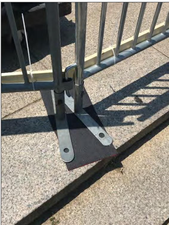
FIGURE 4. TEMPORARY FENCING WITH NON-STAINING CUSHIONING MATERIAL ON HISTORIC GRANITE.
