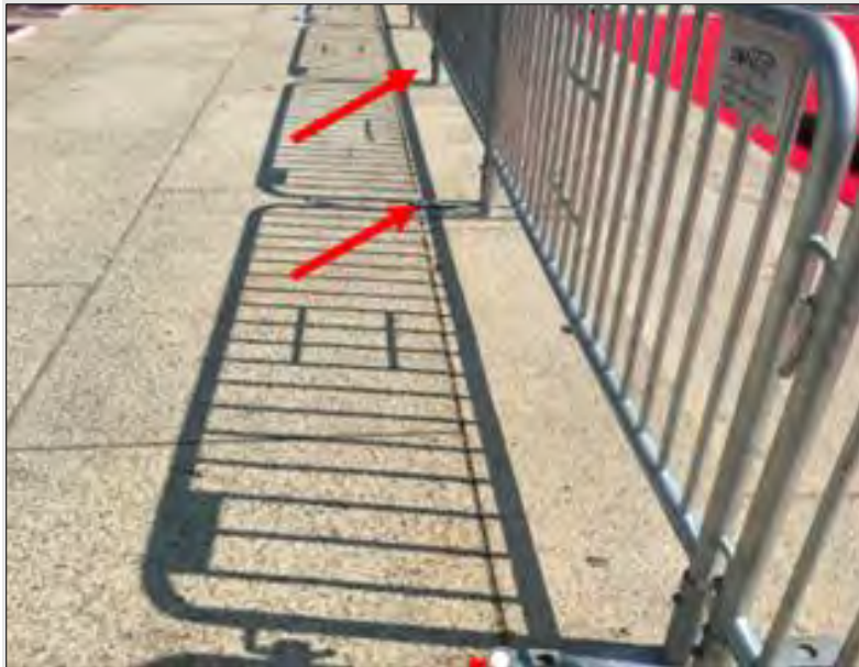
FIGURE 1. EXAMPLE OF TEMPORARY PROTECTION ON HARDSCAPE WITHOUT PROTECTION ON HISTORIC GRANITE.
