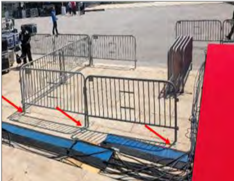
FIGURE 2. EXAMPLE OF TEMPORARY PROTECTION ON HARDSCAPE ON HISTORIC GRANITE.
