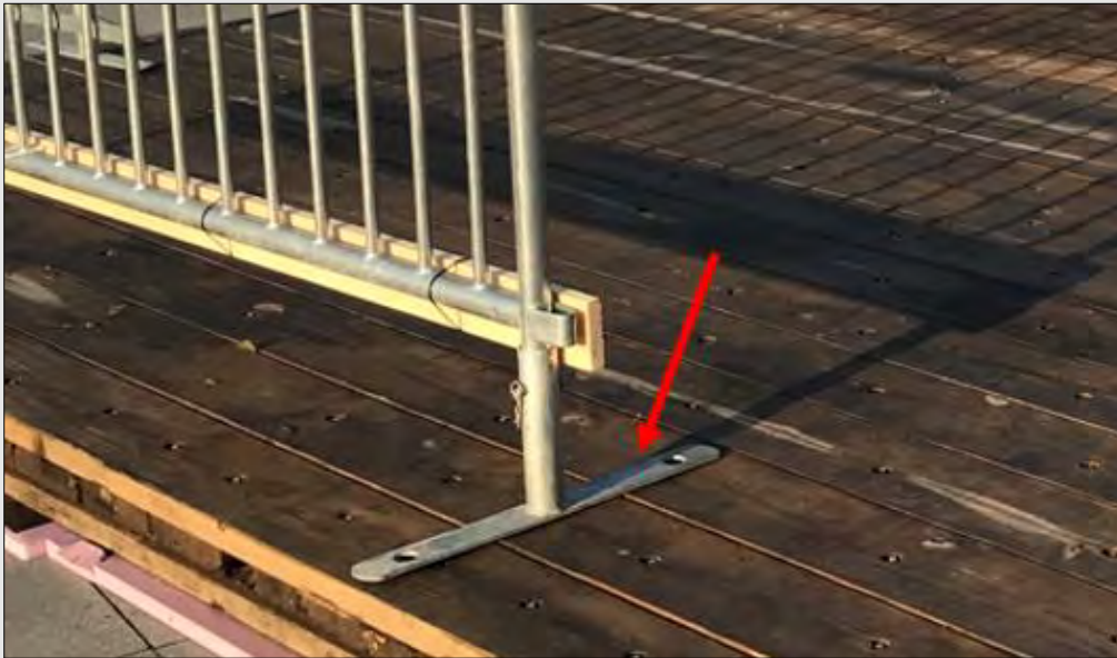
FIGURE 3. GRANITE PAVING PROTECTED BY WOOD AND POLYSTYRENE BASE.
