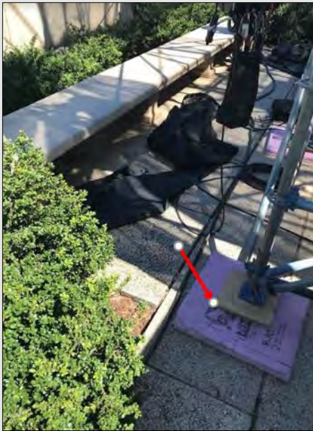
FIGURE 5. PROTECTION UNDER ALL POINTS OF CONTACT OF SCAFFOLDING.
