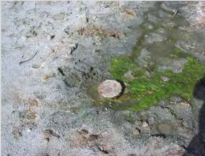
Watson Well is a capped drilled well
