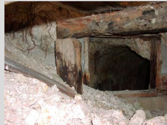
Budweiser Spring water source is in a tunnel excavated in granitic rock
