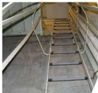
Metal ladder and safety cage at Delta-01.
