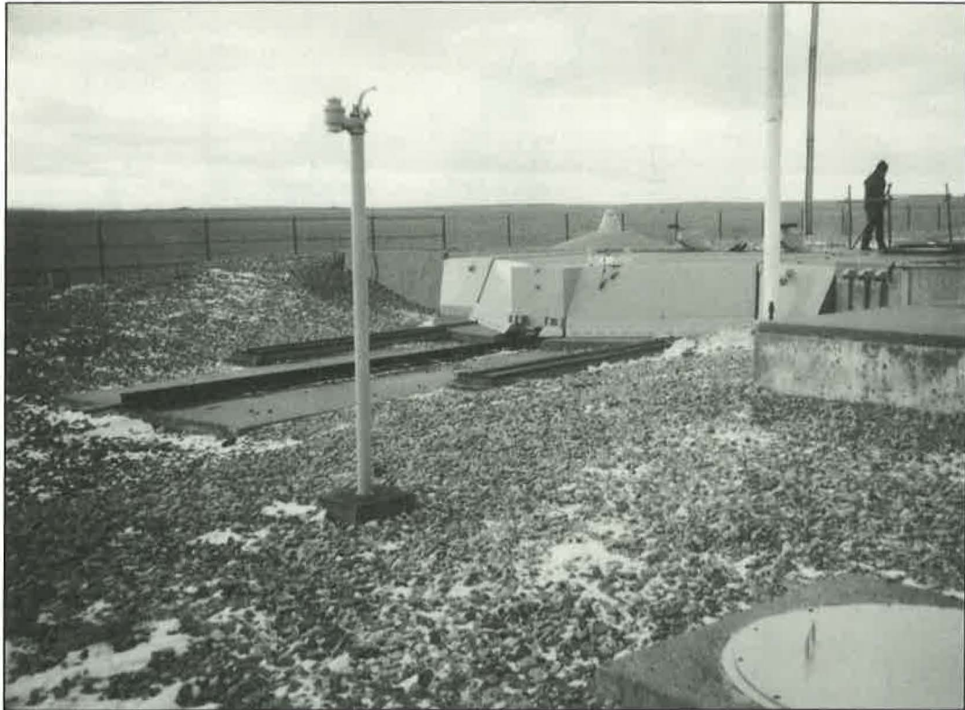
An 80-ton, sliding, reinforced-concrete, closure door covered the silo. Upon receiving the order to launch, explosive gas generators would have quickly pushed the door open.
