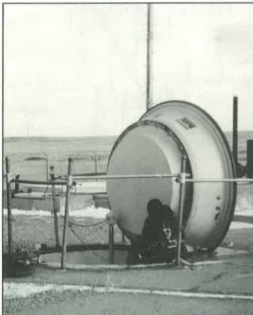
The personnel hatch at Delta Nine provides access to the missile silo and below-ground equipment rooms.
