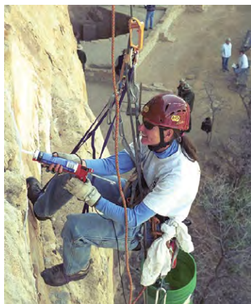
Applying silicon beading at Spruce Tree House.
