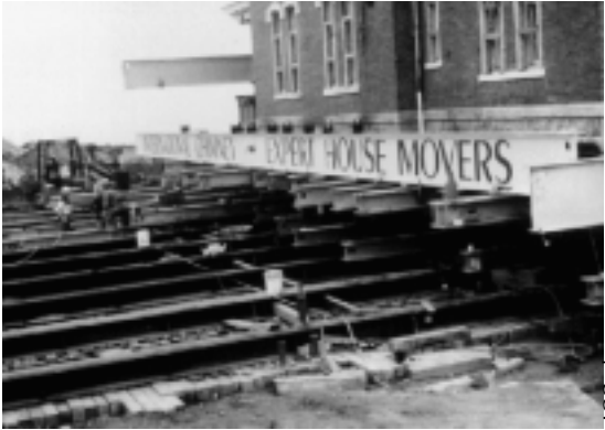
Figure 21. After the first leg of the journey was completed, the track steel was repositioned for a 90° turn.
