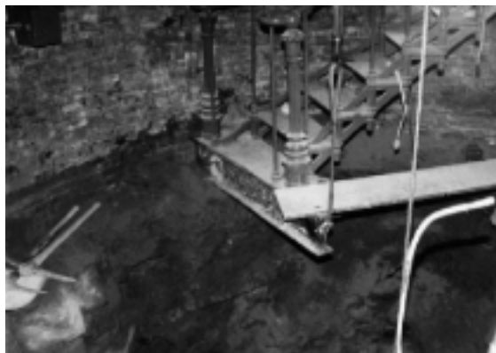
Figure 14. The concrete floor of the light tower was removed and earth excavated by hand in order to perform stabilization from the interior of the structure.
