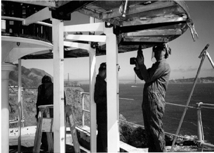
Figure 41. Final fitting and installation of the new aluminum deck plate.
