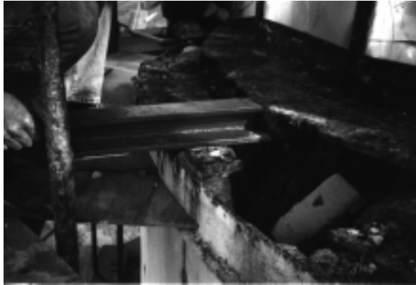
Figure 49. Reconstructing the gallery deck. After removing the existing concrete, remnants of the original cast-iron deck were found.
