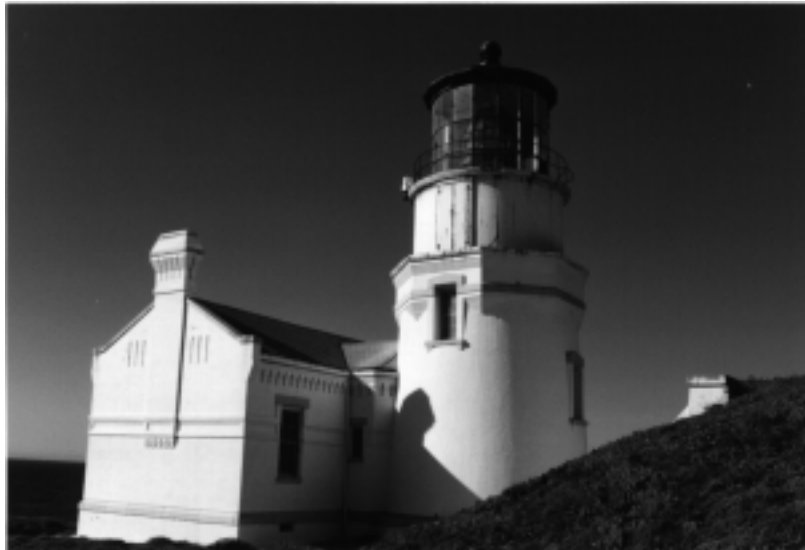
Figure 44. Before the rehabilitation. Note the doors at the watch room. A new louvered panel will be installed for added ventilation.
