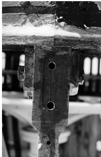
Figure 36. View of the gallery bracket tenons after the holes have been drilled. The tenon on the right connected to the exterior gallery; the tenon on the left is part of the interior gallery deck bracket. The 'v' that has been stamped in the end of the left tenon is an assembly identification mark.
