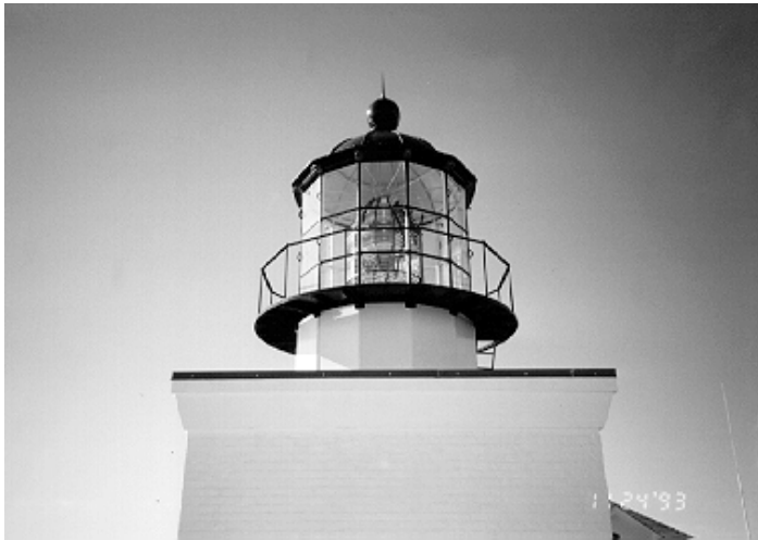
Figure 42. View of the Point Bonita Lighthouse after the gallery deck replacement.
