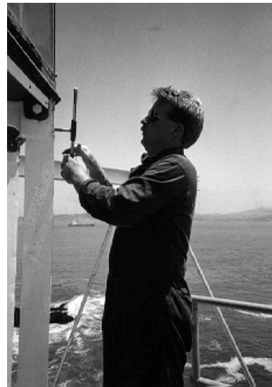
Figure 37. After drilling, threads were cut into each hole using a hand-operated tap.
