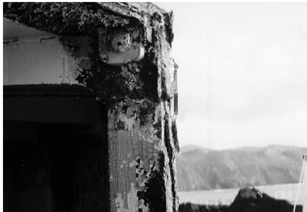
Figure 34. Close-up showing what remained after the gallery deck brackets were cut off with a torch. Note the heavy rust and paint failure caused by exposure.
