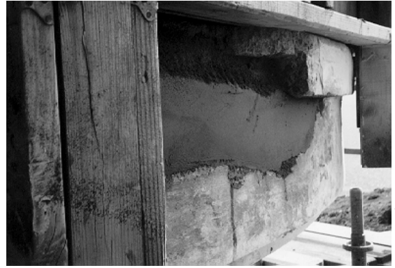
Figure 29. The first application of the mortar patch material to the damaged concrete.
