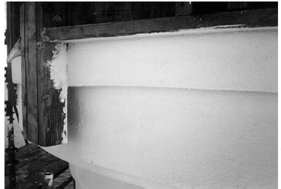
Figure 30. The finished concrete repair is virtually invisible after the surface has been painted.
