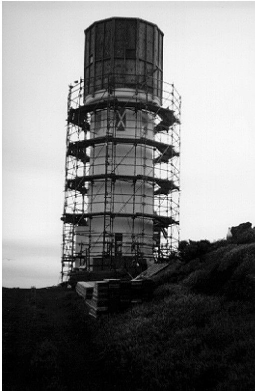
Figure 21. View of the plywood lantern enclosure and scaffolding.
