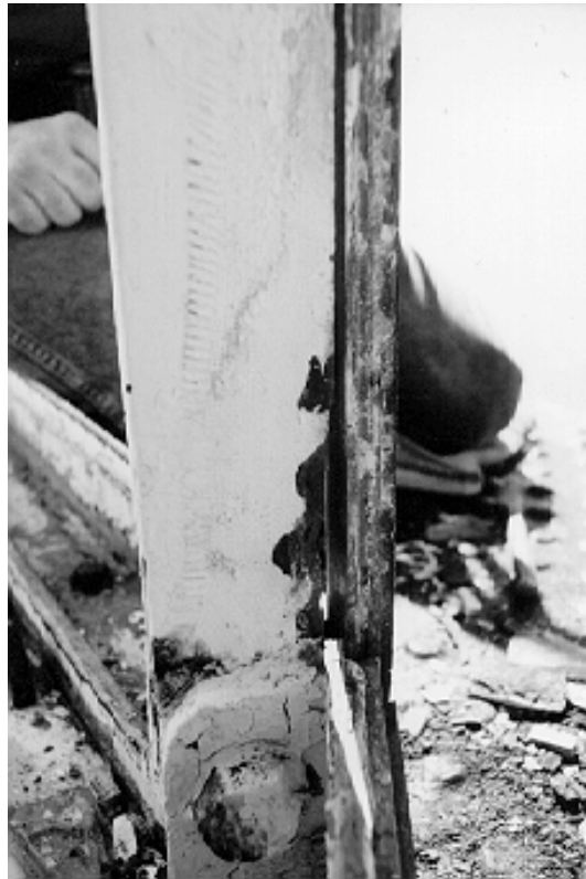
Figure 11. The extent of the damage to the cast-iron column through exfoliation can be seen in profile after the removal of loose rust and the lower bronze mullion.
