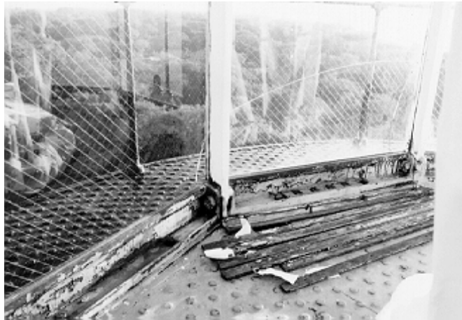
Figure 10. Oblique of the interior of the lantern room with exterior bronze astragals stored in the foreground before cleaning and removal of the extent wire-glass panels.
