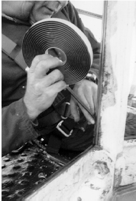
Figure 15. The polybutyl sealant tape was placed on all receiving surfaces on the plane of the interior face of the glass and on the inside faces of the exterior astragals.
