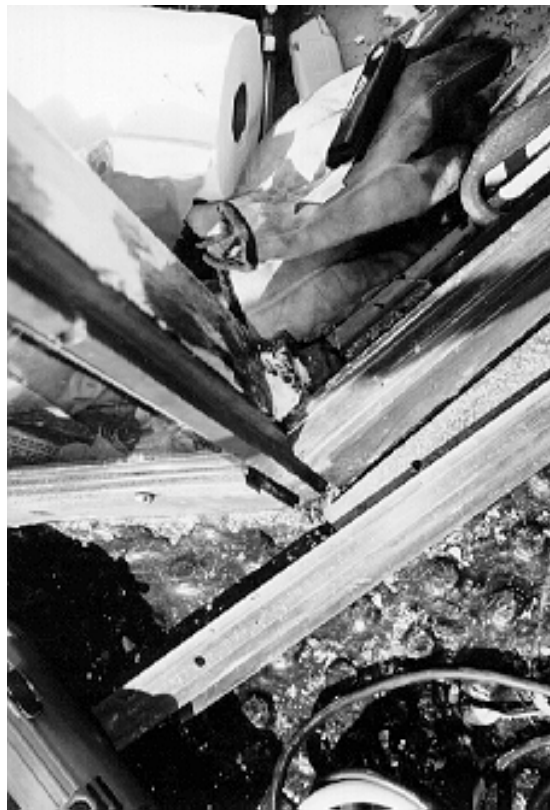
Figure 14. Following placement of the restored bronze mullion, the fenestration is ready to receive the new glazing system.
