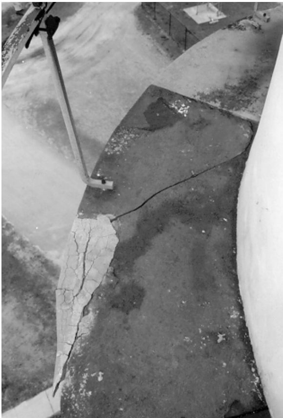
Figure 19. The repair made to this stone gallery deck has begun to deteriorate; moisture penetration is occurring. This condition should be addressed before mothballing.
