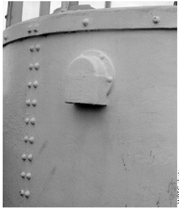
Figure 9. An example of a parapet-wall-mounted vent on a fourth-order lantern.
