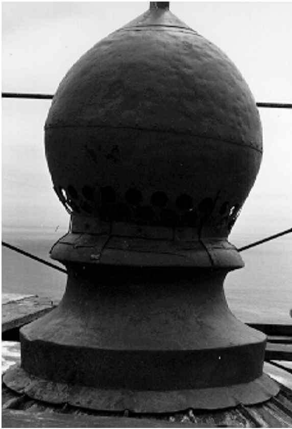
Figure 8. Despite the fact that this first-order lantern ventilation ball has been repaired several times, it still provides adequate lantern ventilation.
