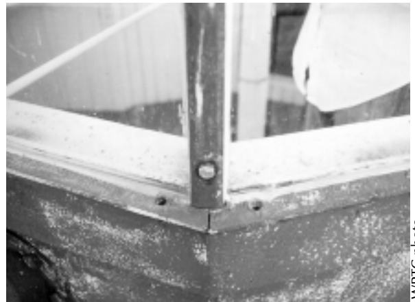
Figure 10. Close-up of missing clamp bolts; these bolts should be replaced to keep this area weather tight.
