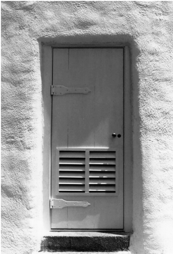
Figure 3. View of the simple pre-Civil-War-style replacement plank door at the Ocracoke Lighthouse, North Carolina.
