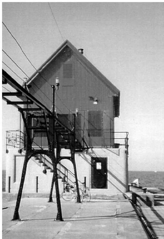
Figure 15. View of watertight 'ship' style door installation on the Grand Haven South Pierhead Front Range Light, Grand Haven, Michigan.
