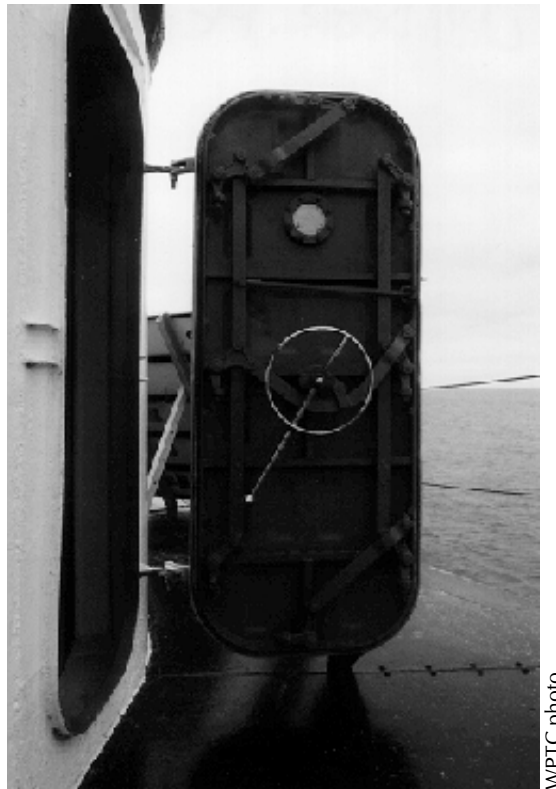
Figure 8. An example of a typical watertight 'ship' style door at Los Angeles Harbor Lighthouse, California.
