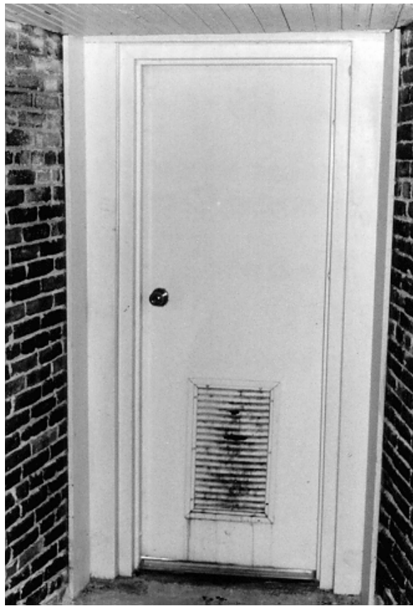
Figure 10. Interior view of the modern metal door at the Ocracoke Lighthouse before its replacement; corrosion like this should be removed and the affected areas treated with a rust-inhibiting coating system.
