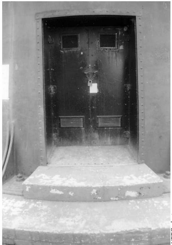
Figure 7. Another variation on the double-leaf, sheet-iron door configuration at the Cape Canaveral Lighthouse, Florida.
