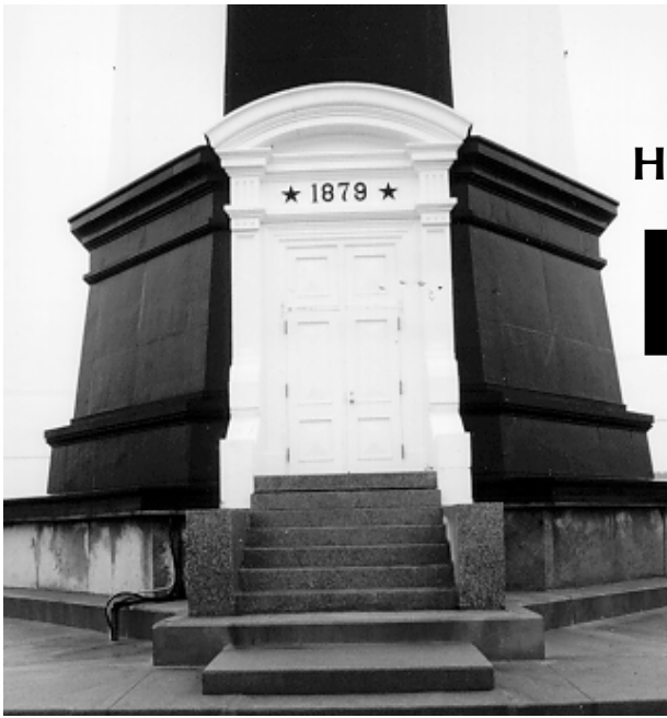
Figure 1. Close-up of large, double-leaf, wood-frame and panel doors at the Cape Henry Lighthouse (second tower), Fort Story, Virginia.
