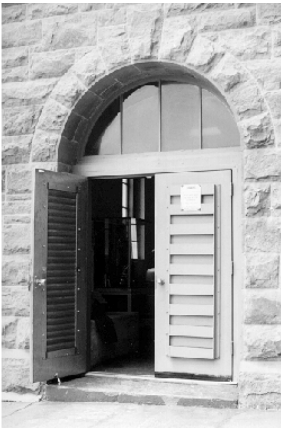
Figure 11. These louvered doors have been installed at Point Sur Light Station for security and ventilation. Note the baffles on the exterior and the screened louvers on the interior.
