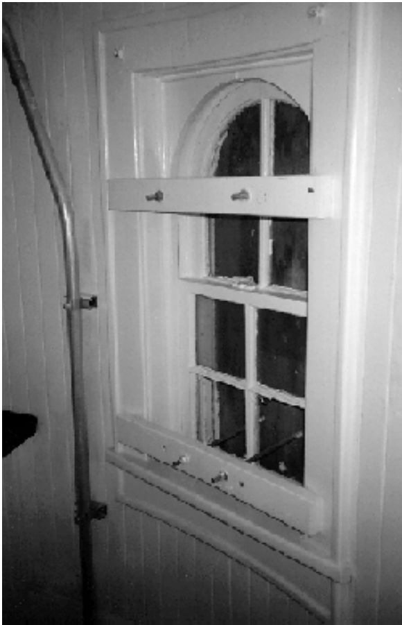
Figure 5. Interior view of the blocked window. If possible, a better solution would have been to raise the lower sash and lower the upper sash and pass the bolts through the openings.
