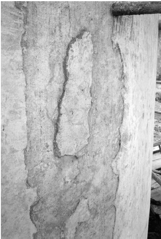
Figure 9. Patches of spalled concrete: familiar with lighthouse preservation the one pictured here should be repaired to protect the underlying concrete structure.
