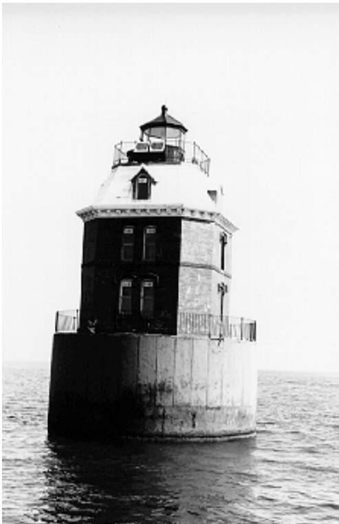
Figure 3. For the construction of this caisson-style lighthouse, unreinforced concrete was used as ballast to sink the cast-iron caisson foundation deep into the mud on the bottom of the Chesapeake Bay in Maryland.
