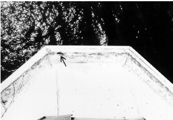
Figure 8. View of a wood-framed lighthouse roof; the arrow indicates where a large hole (approximately 2 by 4 inches) is present in the built-in gutter system. Water entering this hole has caused extensive damage to the interior wood framing members and wood interior wall paneling.
