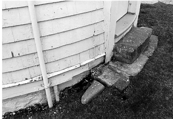
Figure 10. This door sill has a positive slope to ensure proper drainage; the joint where the door surround meets the shingles should be checked for gaps and recaulked if necessary.
