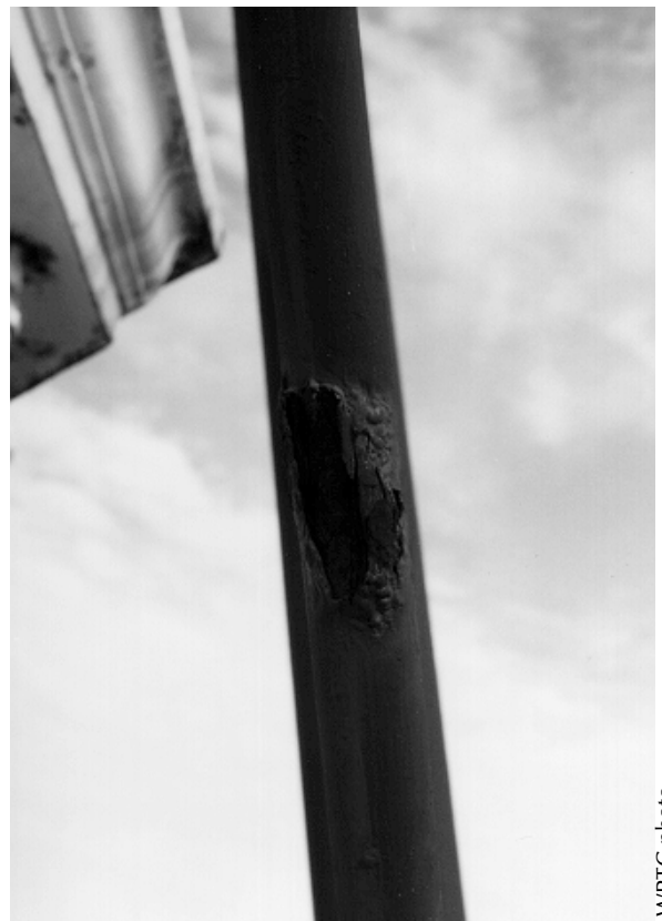
Figure 39. The finish on this tension rod failed and localized corrosion (rust) has formed. The rust is exfoliating in layers that are trapping moisture and causing corrosion to occur deeper and deeper into the tension rod. The result is pitting that will compromise the strength of the tension rod. If the area had been touched up in time, the corrosion might not have formed.
