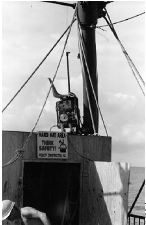
Figure 35. This motorized chair was used to hoist workers as they removed paint from the cast-iron columns at the Sand Key Lighthouse. The chair’s motor is attached to a hoist, so the chair actually climbs a cable that has been strung alongside the column.
