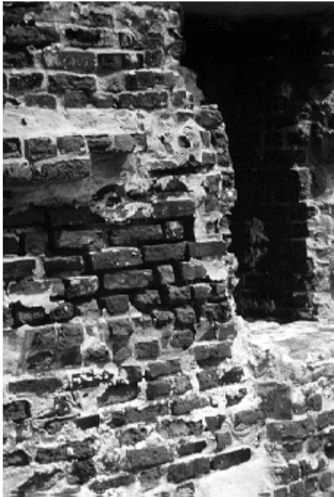
Figure 25. View of the lower portion of the tower showing the more severe deterioration. Note that a large percentage of the first brick wythe is missing or has been removed. The white areas are remains of a portland-cement-based parging applied in the late 1960s in an effort to protect the deteriorating bricks.
