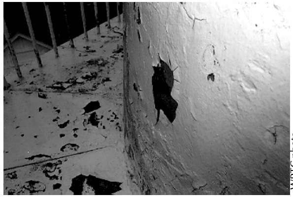
Figure 14. Detail of failing paint, a problem which should be addressed during stabilization and protection. In this particular case, spot painting may be all that is required to maintain a weatherproof protective coating.
