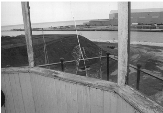
Figure 7. Lantern glass with holes and/or cracks should be replaced as soon as possible to minimize water infiltration. If immediate replacement is not feasible, the glass can be temporarily patched.
