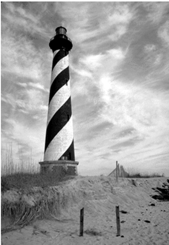
Figure 16. Daymark patterns are a character-defining feature and should be preserved.
