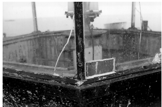
Figure 8. Detail of an acceptable temporary repair to a lantern glass using a piece of painted sheet metal that has been adhered to the glass with a high quality, exterior grade caulk. This type of temporary repair will prevent water from entering the lantern and therefore help avoid further damage. This fix should be considered only as an interim treatment until replacement of the lantern glass.
