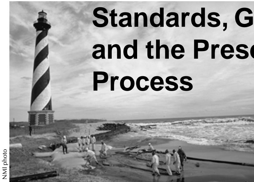
Figure 1. Sandbags are used to protect Cape Hatteras Lighthouse, Buxton, North Carolina, from further shoreline erosion.
