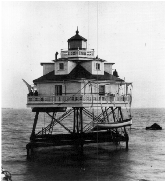
Figure 6. Thomas Point Shoals Lighthouse with screwpile foundation located in Maryland's Chesapeake Bay; shown here in 1885.
