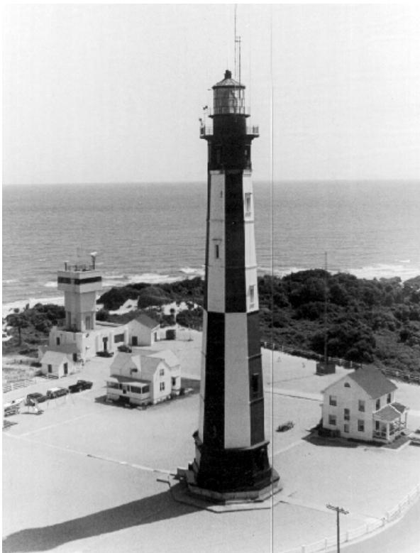
Figure 4. Cape Henry Light Station, cast-iron tower, Fort Story, Virginia.
