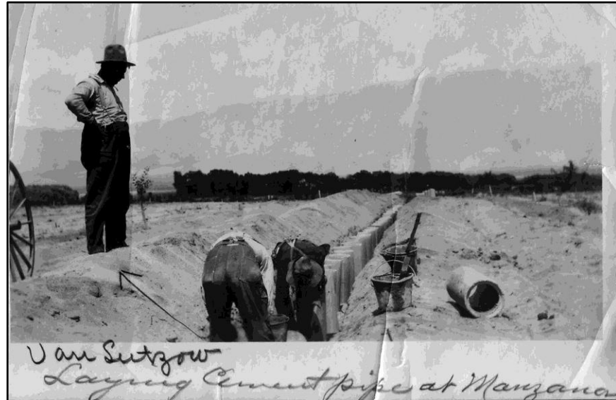
Figure 57: Laying concrete irrigation pipe at Manzanar, ca. 1910 (County of Inyo, Eastern California Museum).
