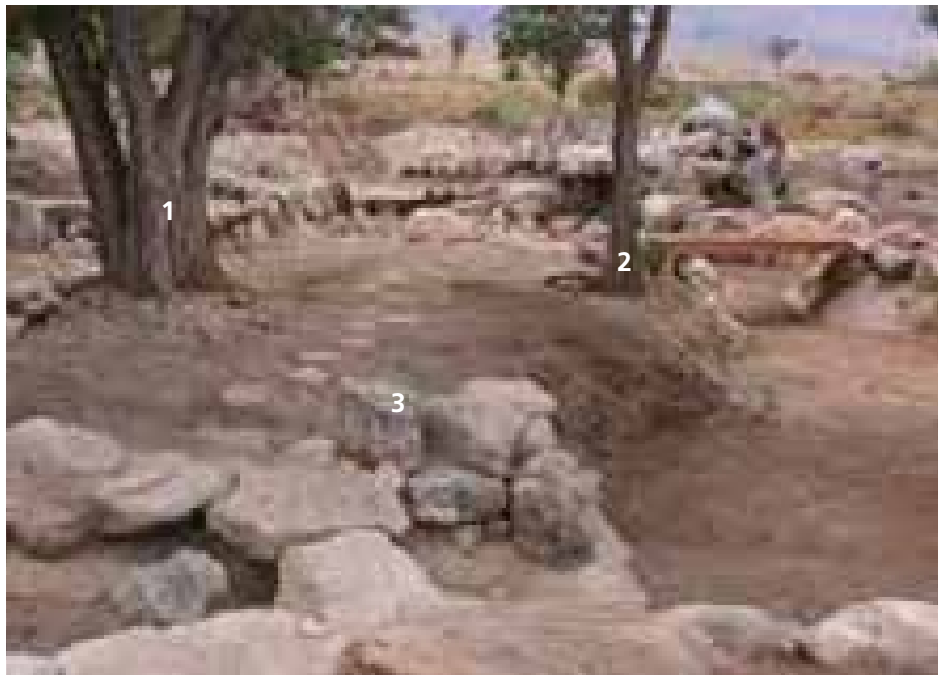
Figure 4.397. Trees (1 and 2) and rock (3) at upper pond at Merritt Park after excavation.
