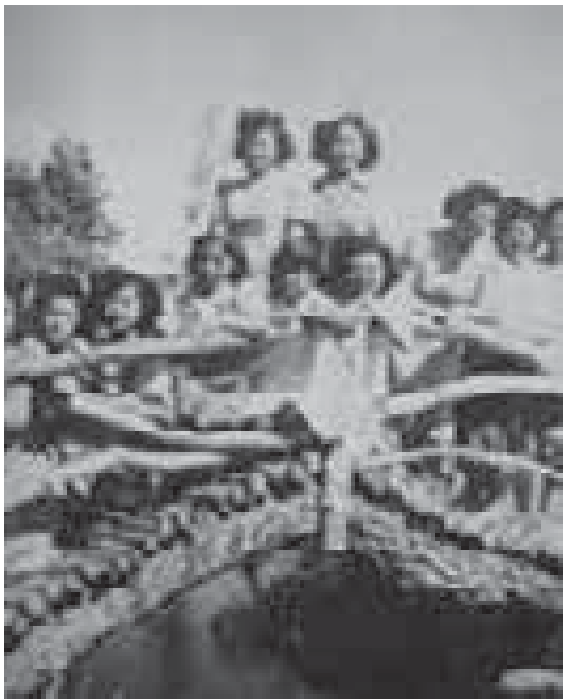
Figure 2.75. Arched bridge at Merritt Park (Mary Ichino Collection, Manzanar NHS).
