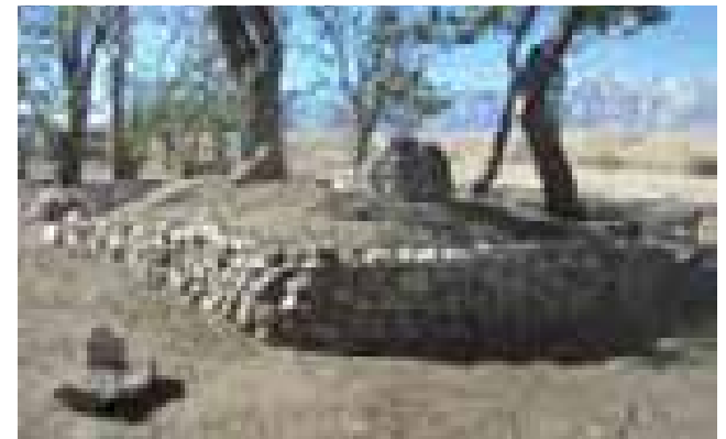
Figure 4.77. Retaining wall at Block 12 mess hall garden after restoration.
