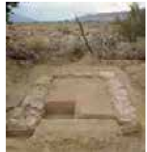
Figure 4.494. Foundation of sentry post at the military police compound.
