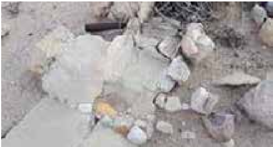
Figure 4.347. Stepped water course at Block 36 Barracks 12 Apartment 4 garden.
