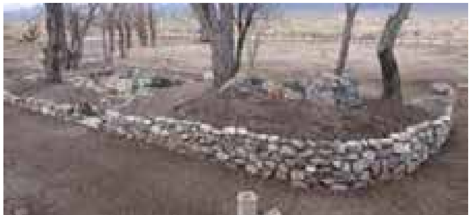
Figure 4.66. Retaining wall at Block 12 mess hall garden.
