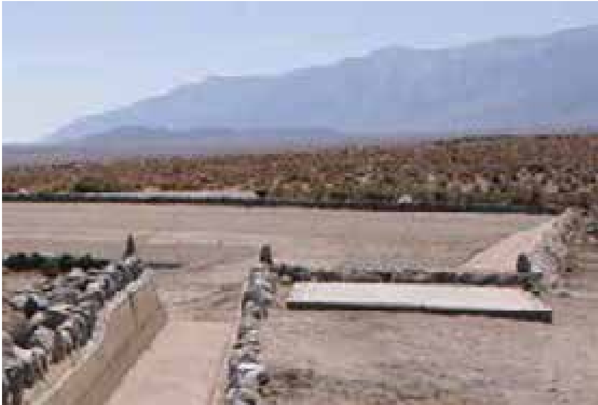
Figure 4.518. Reservoir inlet with vertical rocks.
