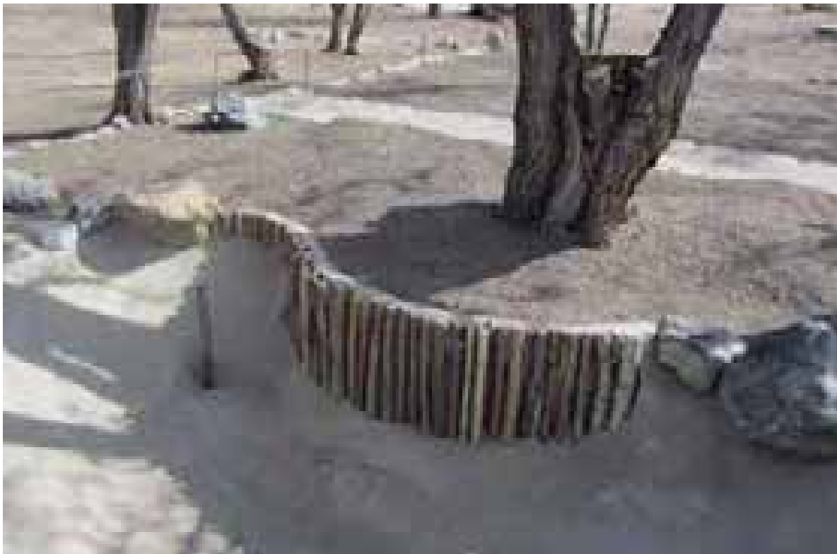
Figure 4.80. Restored rangui post wall at Block 12 mess hall garden.
