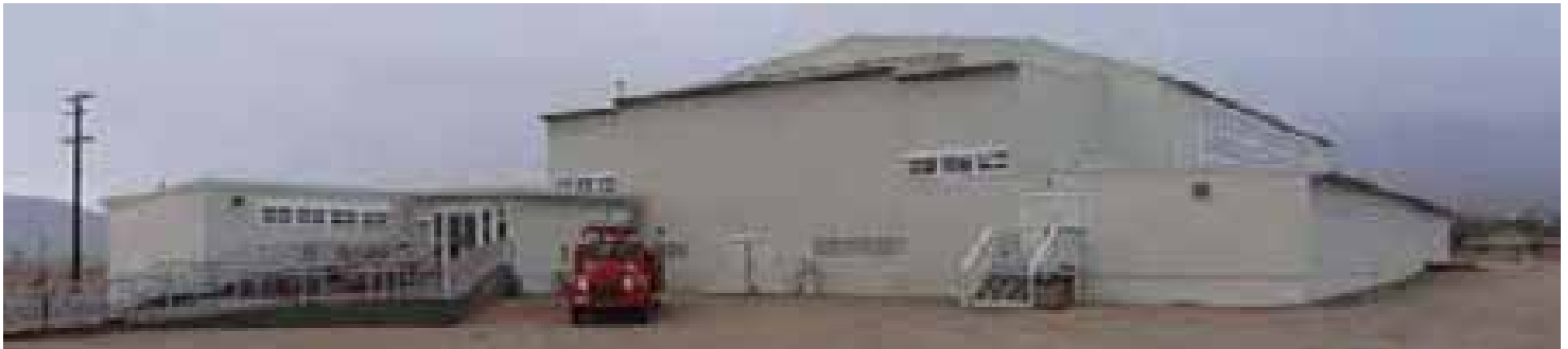
Figure 7.6. Rehabilitation: auditorium visitor center (photograph by Dick Lord).
