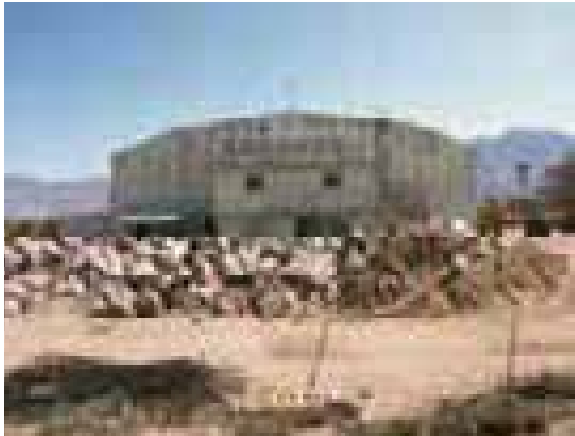
Figure 4.496. West side of the auditorium in 1993.
