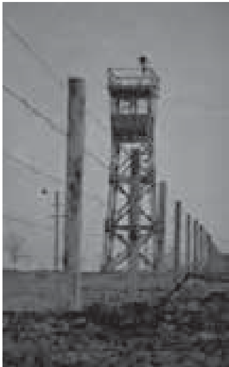
Figure 2.179. Guard tower (Yuri Matsunaga Collection, Manzanar NHS).
