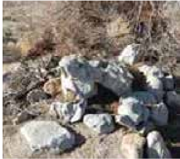
Figure 4.271. Lantern leg made of rock and concrete between Barracks 8 and 9 in Block 26.
