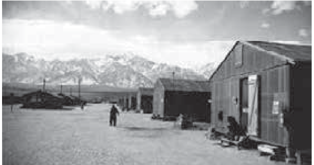
Figure 4.12. Barracks 8 (foreground) through 14 in Block 2 (Ansel Adams, Library of Congress).
