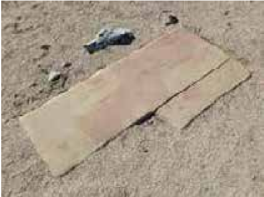
Figure 4.51. Faux-wood entry at Block 9 mess hall.
