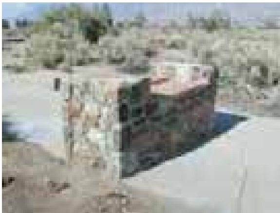
Figure 4.480. Rock and concrete pedestal with faux-wood at staff housing Building C.
