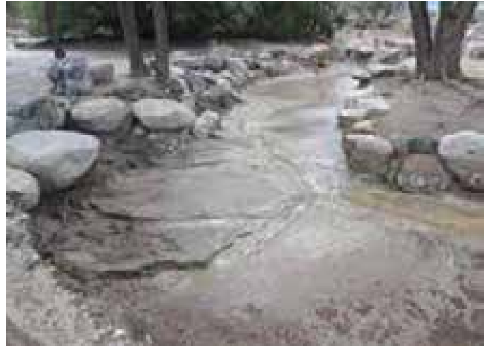
Figure 4.443. Flood damage to upper pond at Merritt Park.
