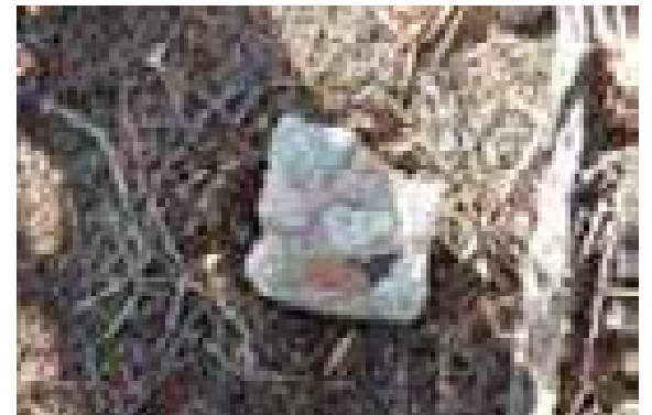
Figure 4.220. Top of concrete pedestal at Block 22 Barracks 12.
