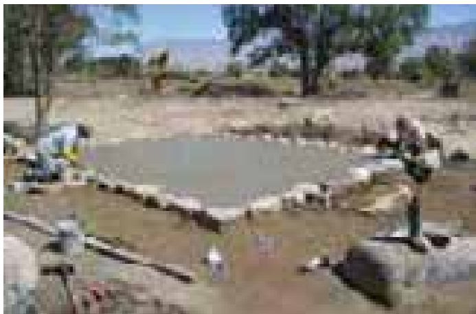
Figure 4.399. Replacing concrete slab at Merritt Park tea house.
