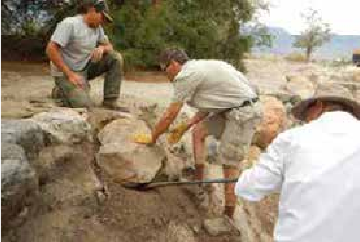
Figure 8.4. Resetting fallen rock at Merritt Park in 2014.
