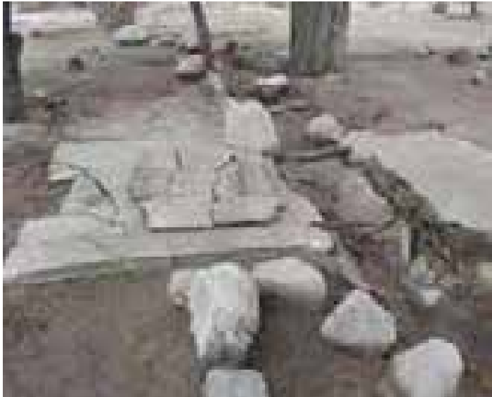
Figure 8.10. Broken concrete bridge at Block 24 Barracks 5.
