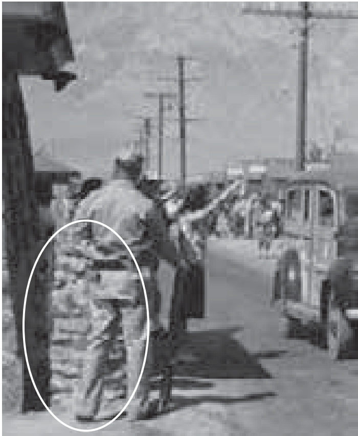
Figure 4.458. Faux-wood stump under construction at military police sentry post (Merritt Collection, Eastern California Museum).
