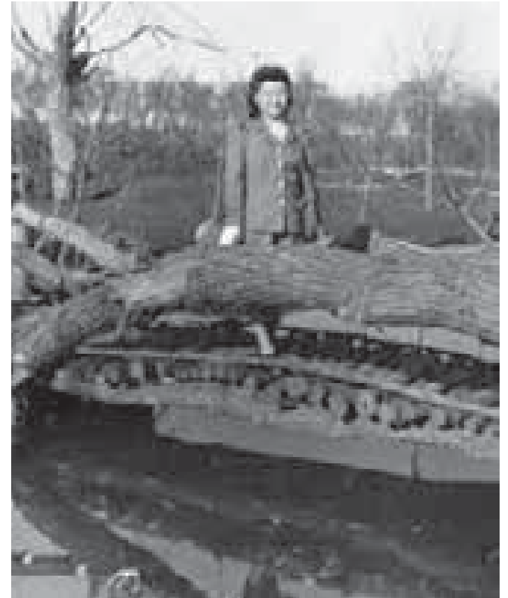
Figure 2.84. Bridge across lower pond at Merritt Park (photograph by Toyo Miyatake, reproduced with permission © Toyo Miyatake Studio).
