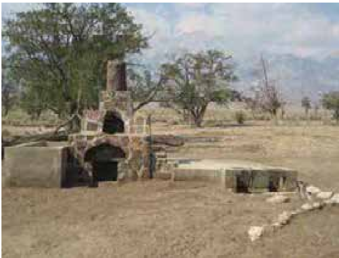
Figure 4.505. Chicken ranch incinerator.
