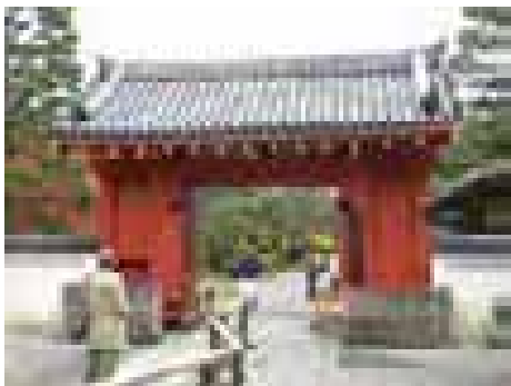
Figure 5.11. Entrance gate at Byodo-in, Uji.
