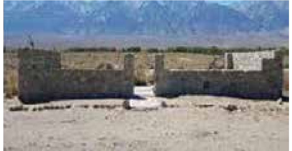
Figure 4.489. Patio wall at staff housing Building G today.
