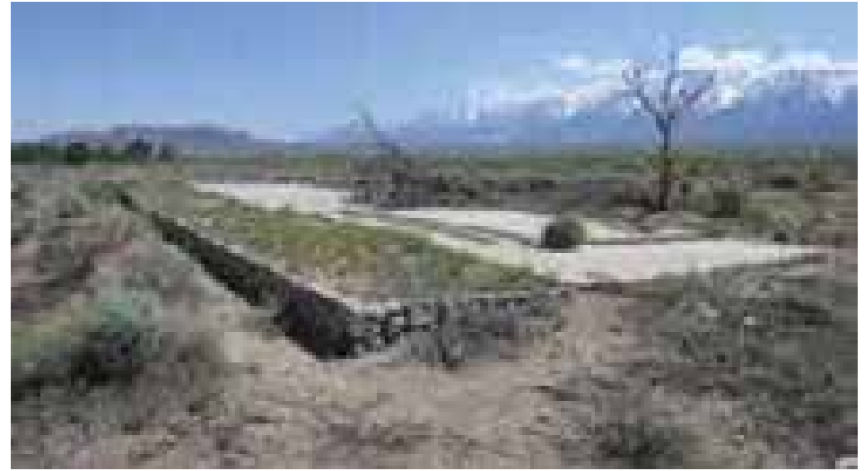
Figure 4.372. Retaining wall at hospital laundry.
