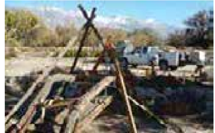
Figure 4.446. Bridge reconstruction at lower pond of Merritt Park in 2014.
