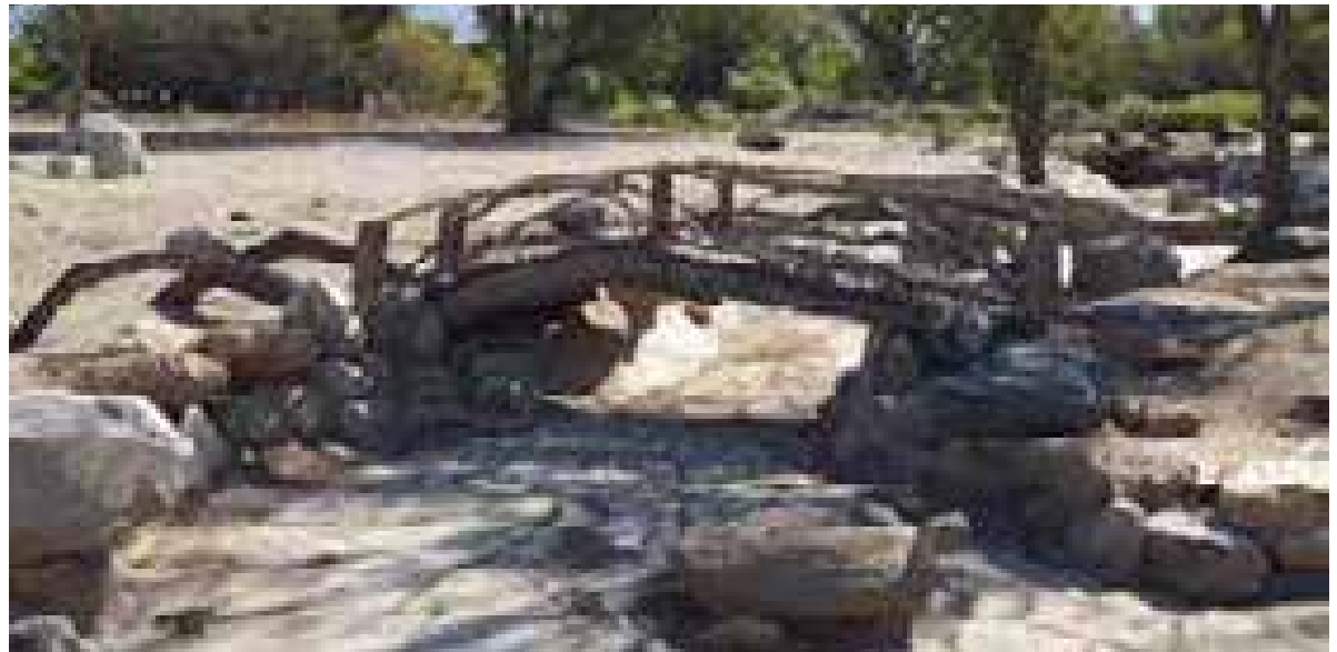
Figure 4.434. Reconstructed bridge at upper pond of Merritt Park.
