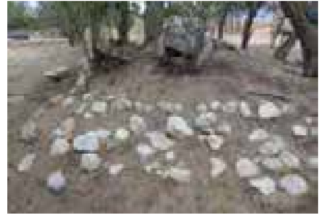
Figure 4.75. Retaining wall at Block 12 mess hall garden prior to preservation work.
