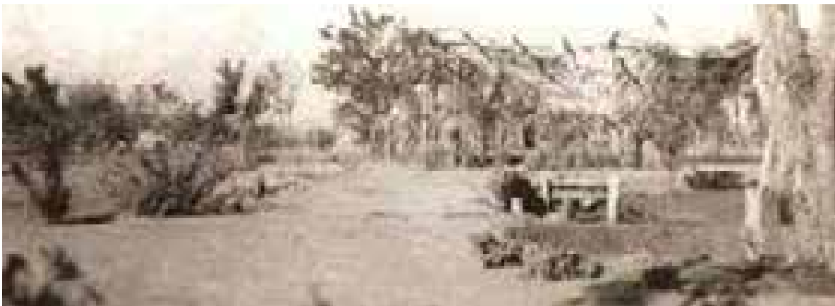
Figure 2.58. Earth-covered bridge at Cherry Park (Yoshie Sakamoto Collection, Manzanar NHS).
