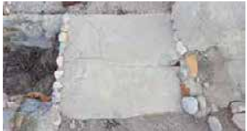
Figure 4.348. Concrete bridge at Block 36 Barracks 12 Apartment 4 garden.
