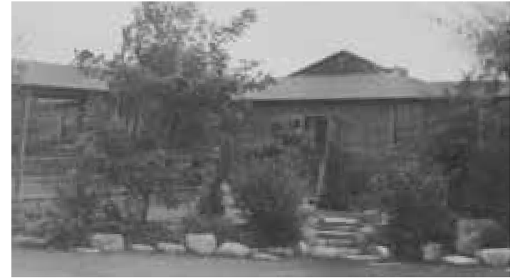
Figure 2.49. Steps and landscaping at the hospital wards (Mary Ichino Collection, Manzanar NHS).
