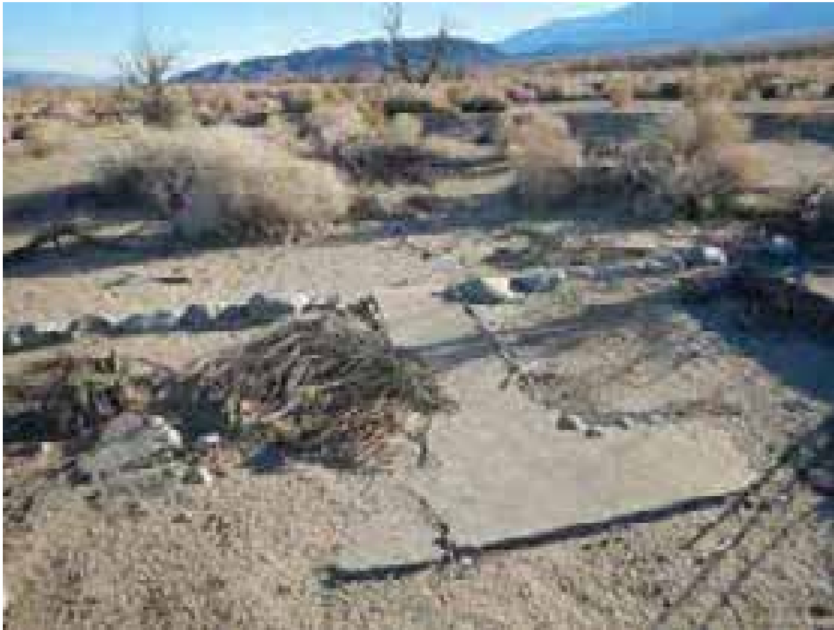
Figure 4.100. Concrete walkway at Block 15 Barracks 8 Apartment 1.
