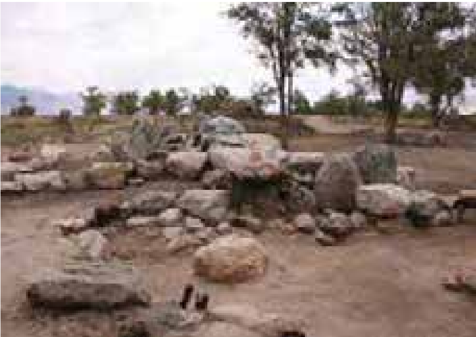
Figure 10.6. Waterfall at Merritt Park after excavation and before stabilization (2008).
