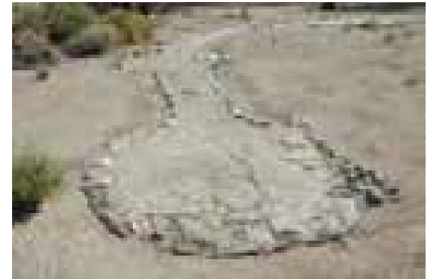
Figure 4.253. Rock-lined concrete walkway on north side of Block 24 mess hall.
