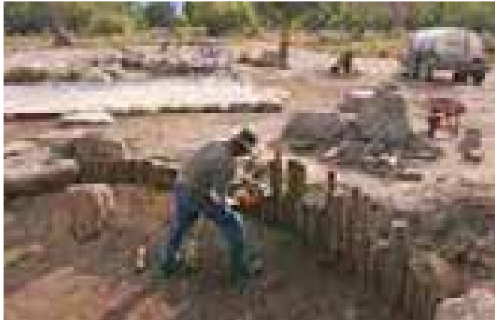
Figure 4.398. Rebuilding rangui post walls at Merritt Park.
