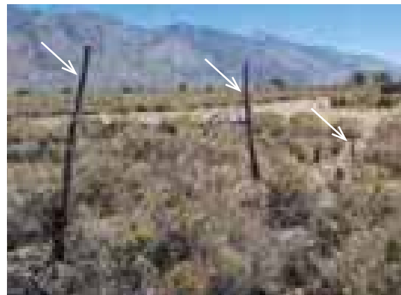
Figure 4.474. Fence posts at staff housing Building A.
