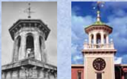
Boott Mill tower, before and after.
