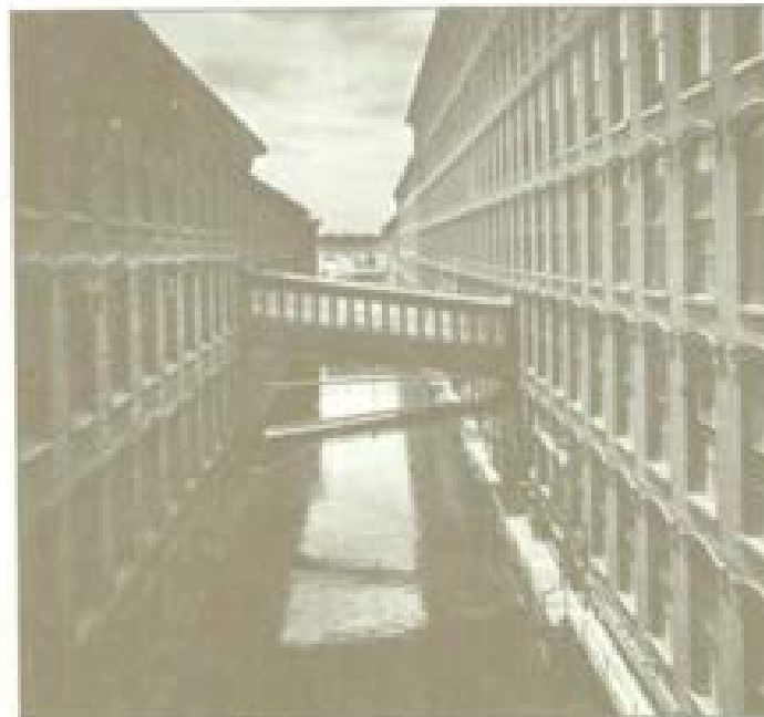
Surviving mill buildings are among Lowell's most important architectural assets. It is imperative that their historic character be preserved.
