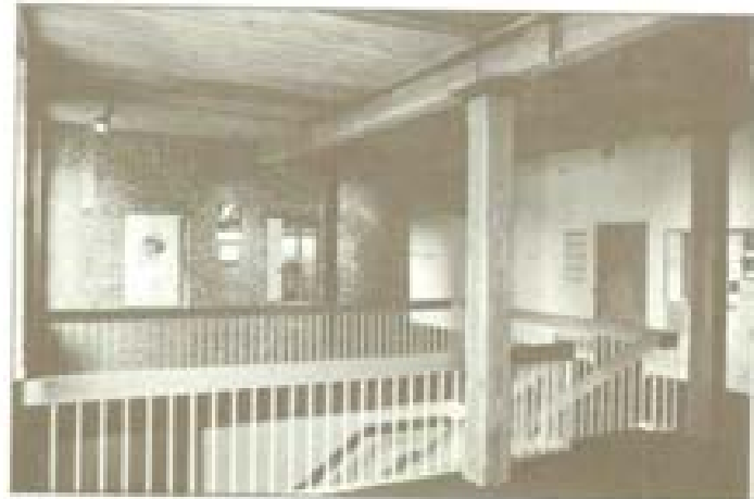
The historic character of a mill interior can be preserved by leaving exposed original brick walls and heavy timber framing.
