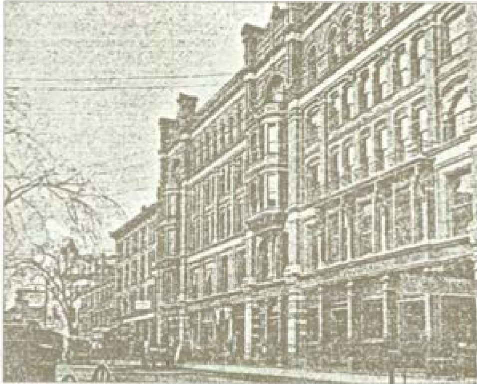
HILDRETH BUILDING 1883 45 Merrimack Street
