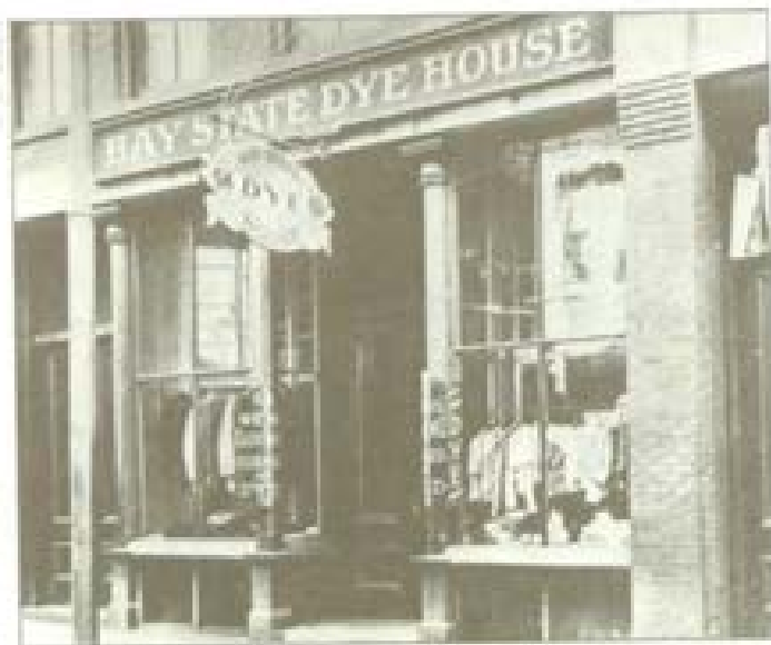
Historical signs usually blended well with building design. The signage was scaled to the pedestrian and isolated so that the essential architectural features were not lost.
