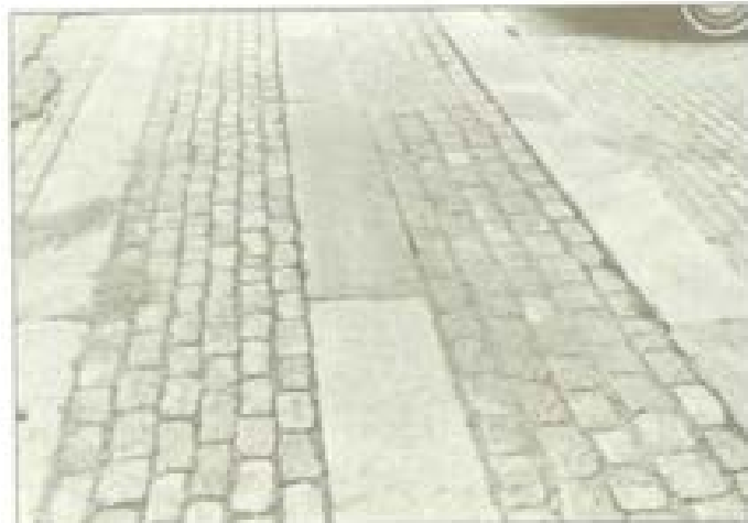
Granite pavement still exists under the asphalt covering on most of the downtown Lowell streets-- its restoration by the City is a good example of what is being recommended in the Standards.
