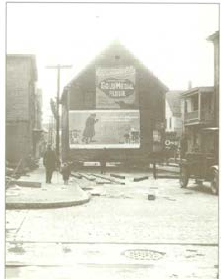
Relocating buildings is an old American practice and also occurred in Lowell. As a last resort to demolition, relocation may need to be considered.
