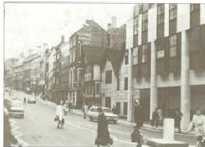
Infill structure of contemporary design was detailed to work with historic facades in Nottingham, England.
