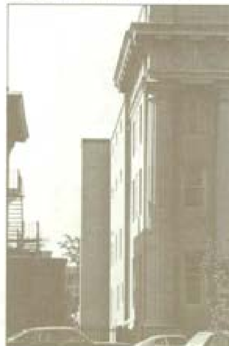
An added elevator or stair tower which has no negative impact on a principle facade of a building can usually be attached to a secondary exterior location.
