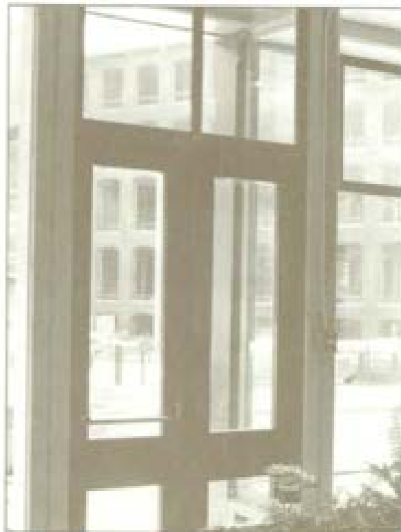
The building code requires two means of egress. This can often be provided in a way that preserves the character of original doorways.
