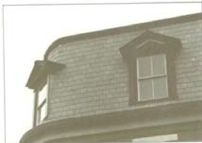
The shape of and materials covering roofs of historic buildings are important. Many of the remaining slate roofs in Lowell are in good condition and should be retained.
