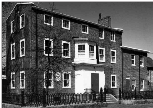
Cambridge Neighborhood House, 79 Moore St., demolished 1973
