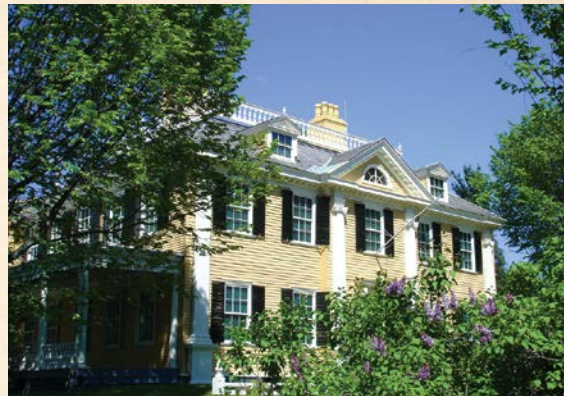
JOHN VASSALL HOUSE
