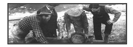
pieces of gold are picked out by hand or with tweezers. Finer grained gold is separated from the commonly associated black sand by using a magnet. After drying, a magnet will attract the magnetite, or "black sand," and leave the gold. "Flour" gold will typically be
