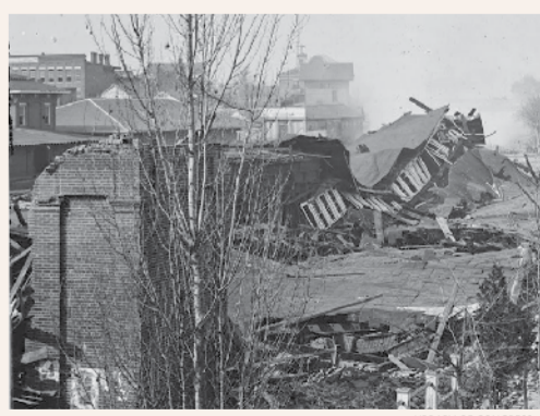
Sherman ordered the destruction of all military and government buildings. The depot was among the casualties (above).
