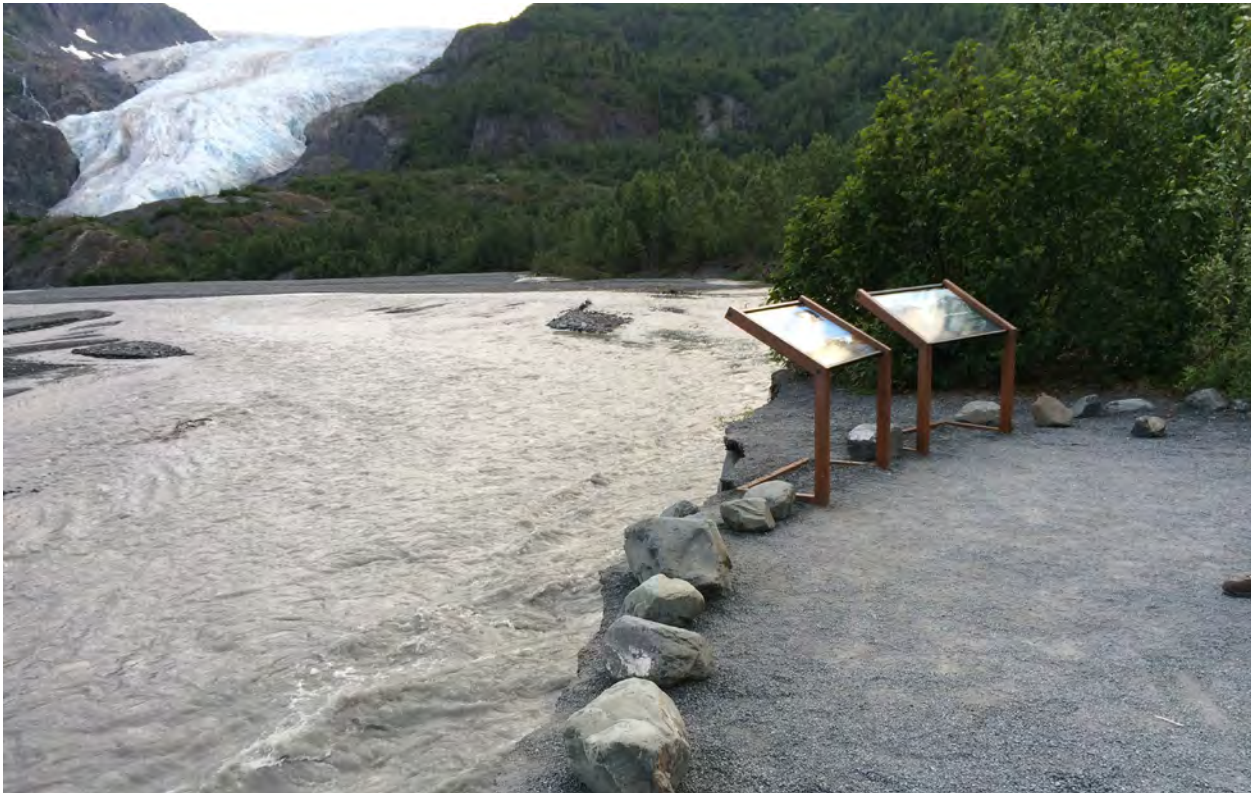
Figure 9 — Erosion at Glacier View Loop Trail in 2014
