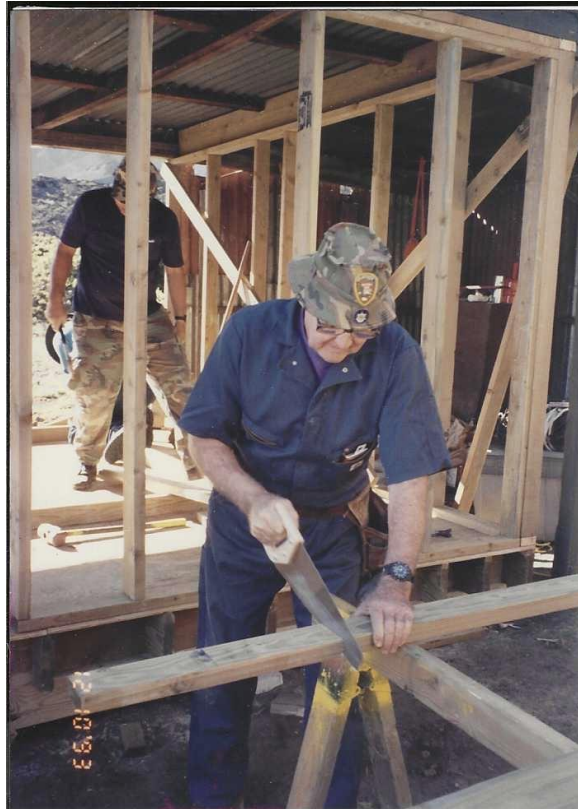
Hōlua Hilton wall framing – Eric Andersen's dad
