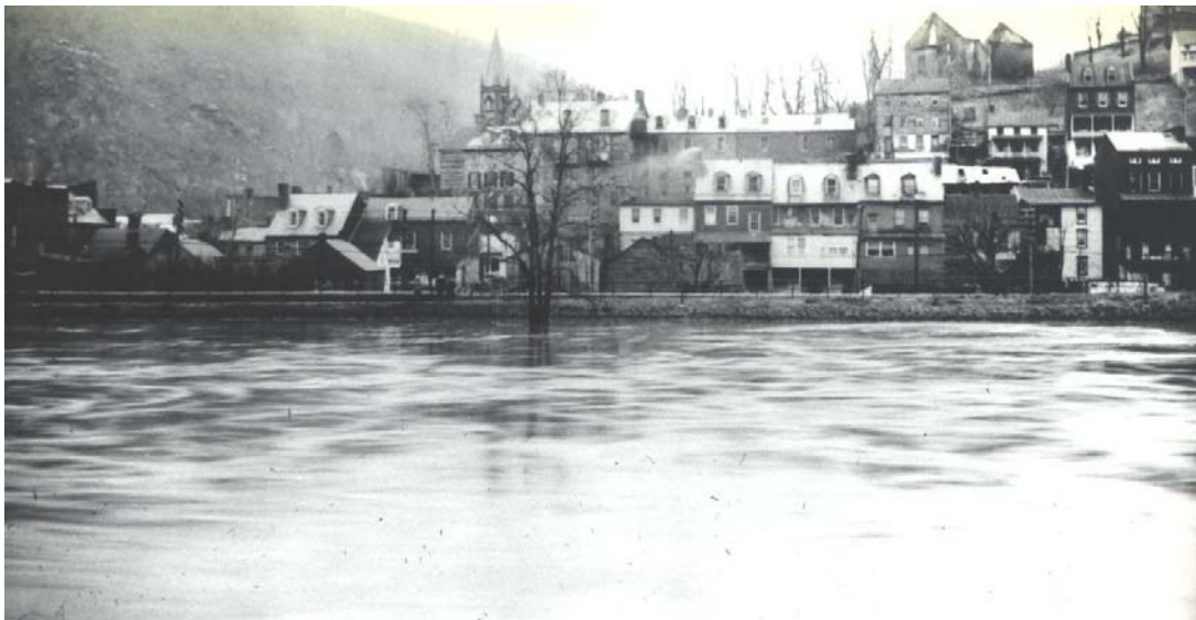
Figure 62 1936 photograph of the Armory site during the largest flood recorded in the town's history. NPS Collection.
