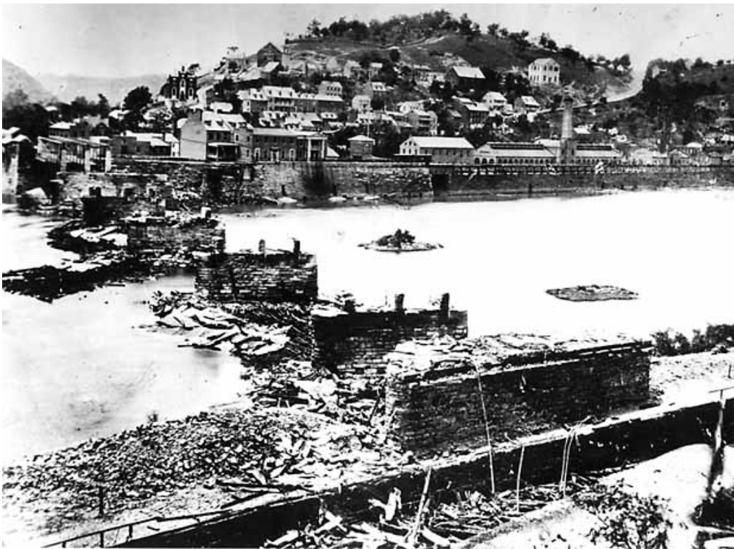
Figure 31 Ruins of Baltimore and Ohio Railroad bridge destroyed by Confederate forces on June 14, 1861. NPS Collection.
