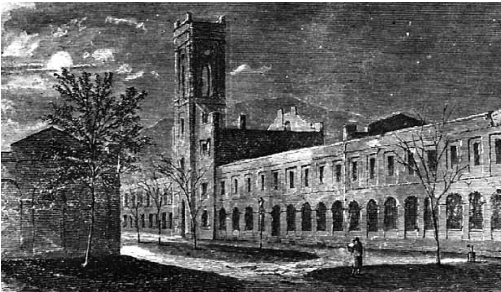
Figure 28 "Harper's Ferry Armory as it now appears," published by Harper's Weekly on July 20, 1861. The square crenellated bell tower was erected between 1860 and 1861. On the right of the tower was a "Workshop for files and cutting and milling machines." NPS Collection.
