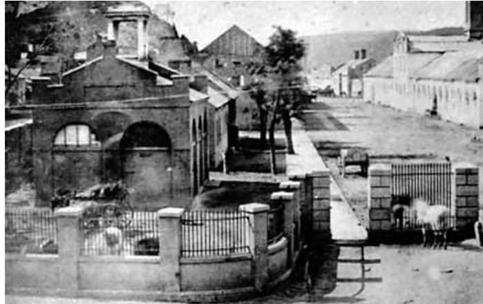
Figure 20 Civil War-era photograph of the armory entrance illustrating wrought iron gates and gate posts. NPS Collection.
