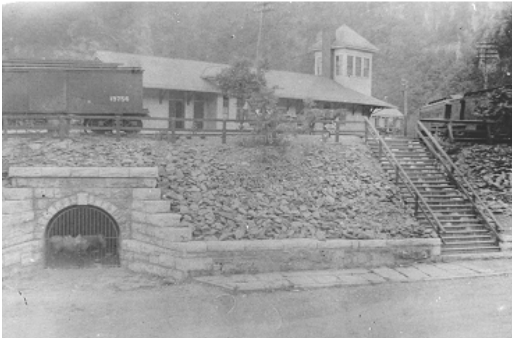
Figure 56 Circa 1894-1900 photograph of the Harpers Ferry train station and drainage culvert at the east end of Shenandoah Street. NPS Collection.
