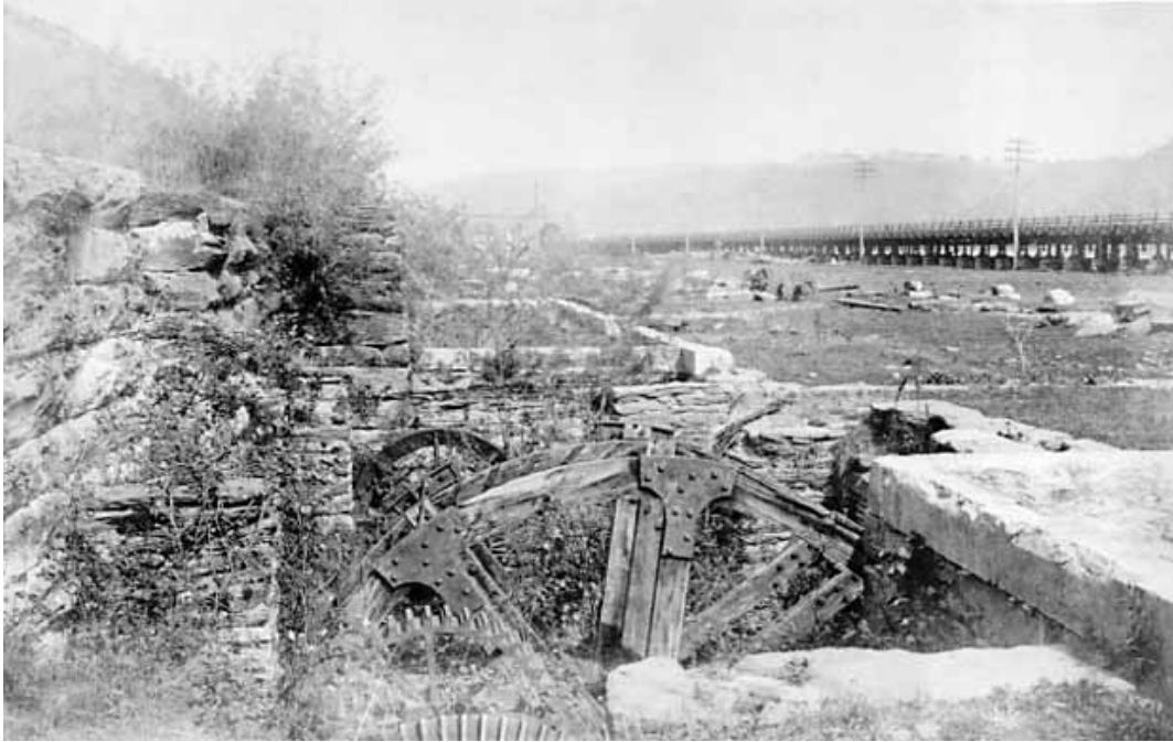
Figure 41 1886 photograph showing the remains of a 15 ft. water wheel at the site of the armory ruins. NPS Collection
