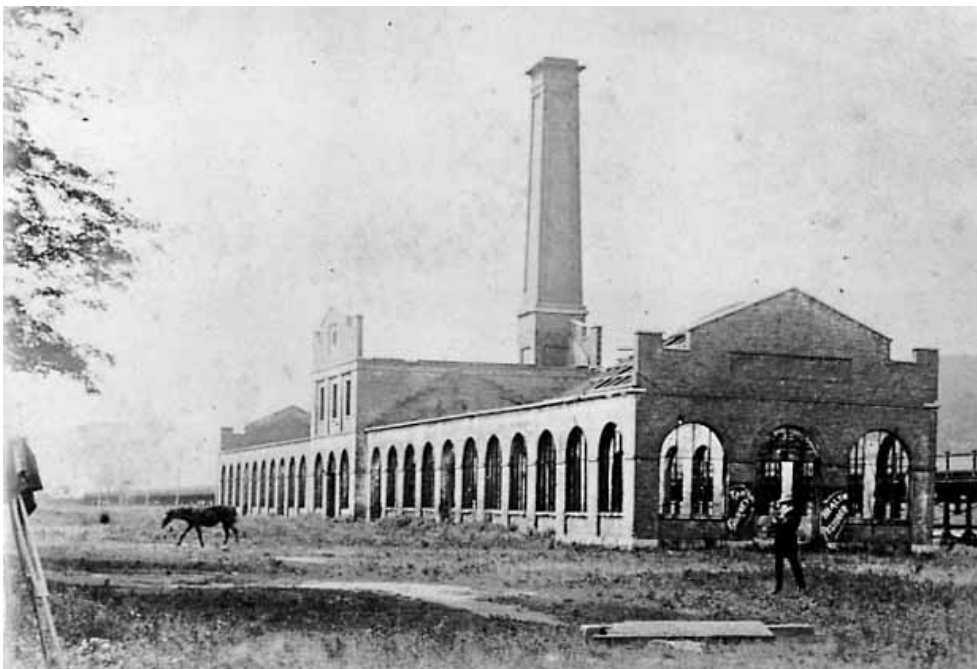
Figure 18 1886 photograph of the Smith and Forging Shop illustrating Symington's standard design plan for a three-part structure. NPS Collection.
