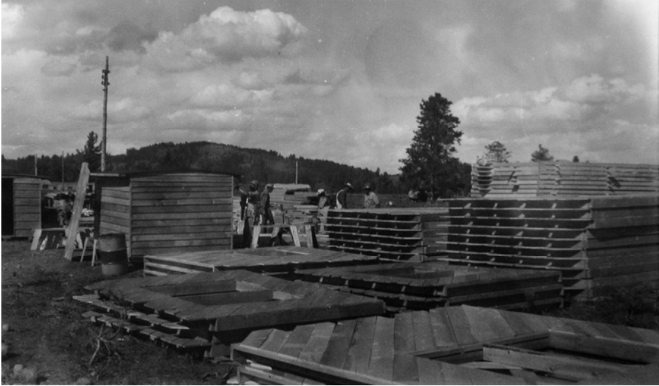
Fig 1.1. Timber wood frame as used in the Employee's Dormitories and the Staff Housing. Rockefeller Archives Center.
