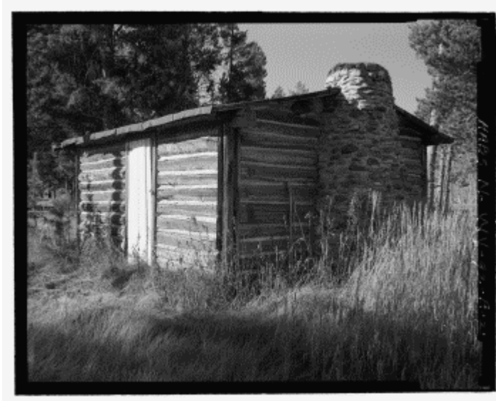
Figure 8- Bar BC Dude Ranch Cabin HABS Photograph
