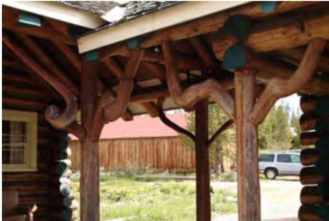
Burlled log hallway at northwest corner
