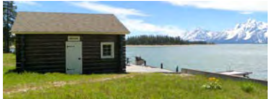
North elevation facing west
