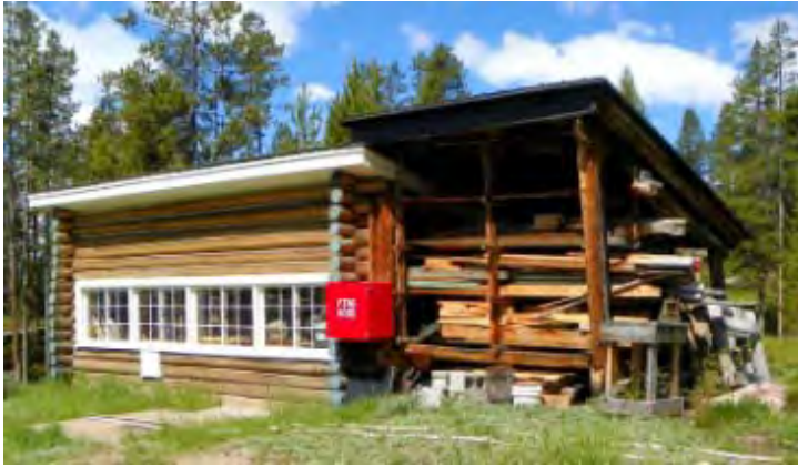
South-facing façade and east elevation
