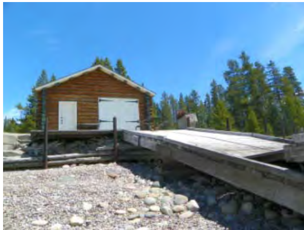
North elevation facing east
