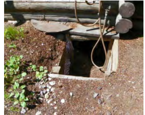
3. Open crawl-space access
