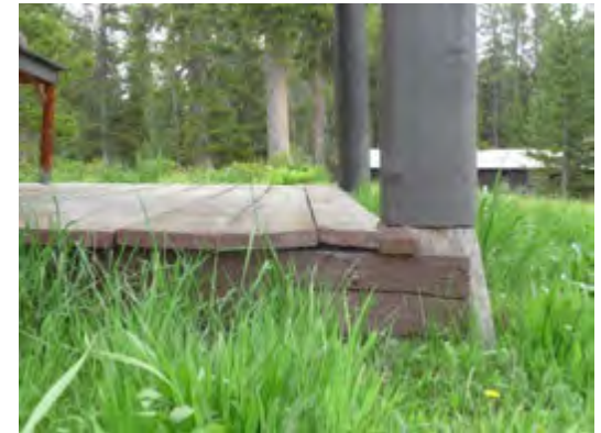
3. North end of porch deck
