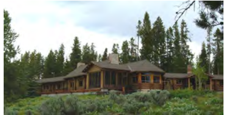
West and south elevations
