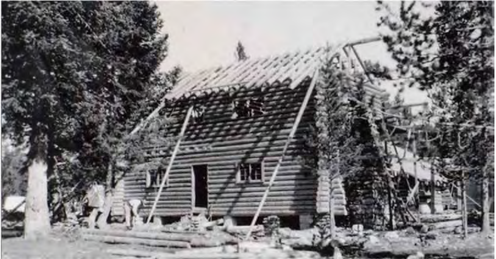
The Johnson Lodge under construction in 1927
