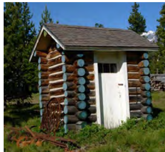
East-facing façade and south elevation
