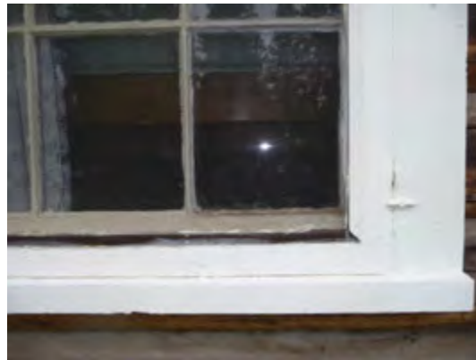
2. Window screen and glazing
