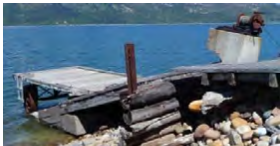
2. Aging mechanical systems.
