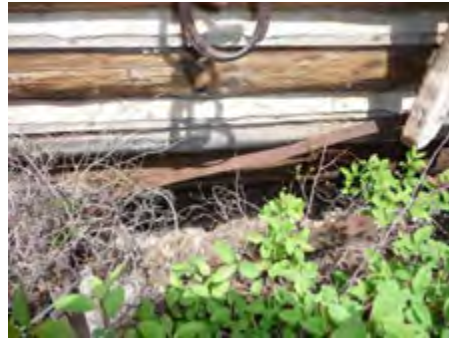
2. Pit under building
