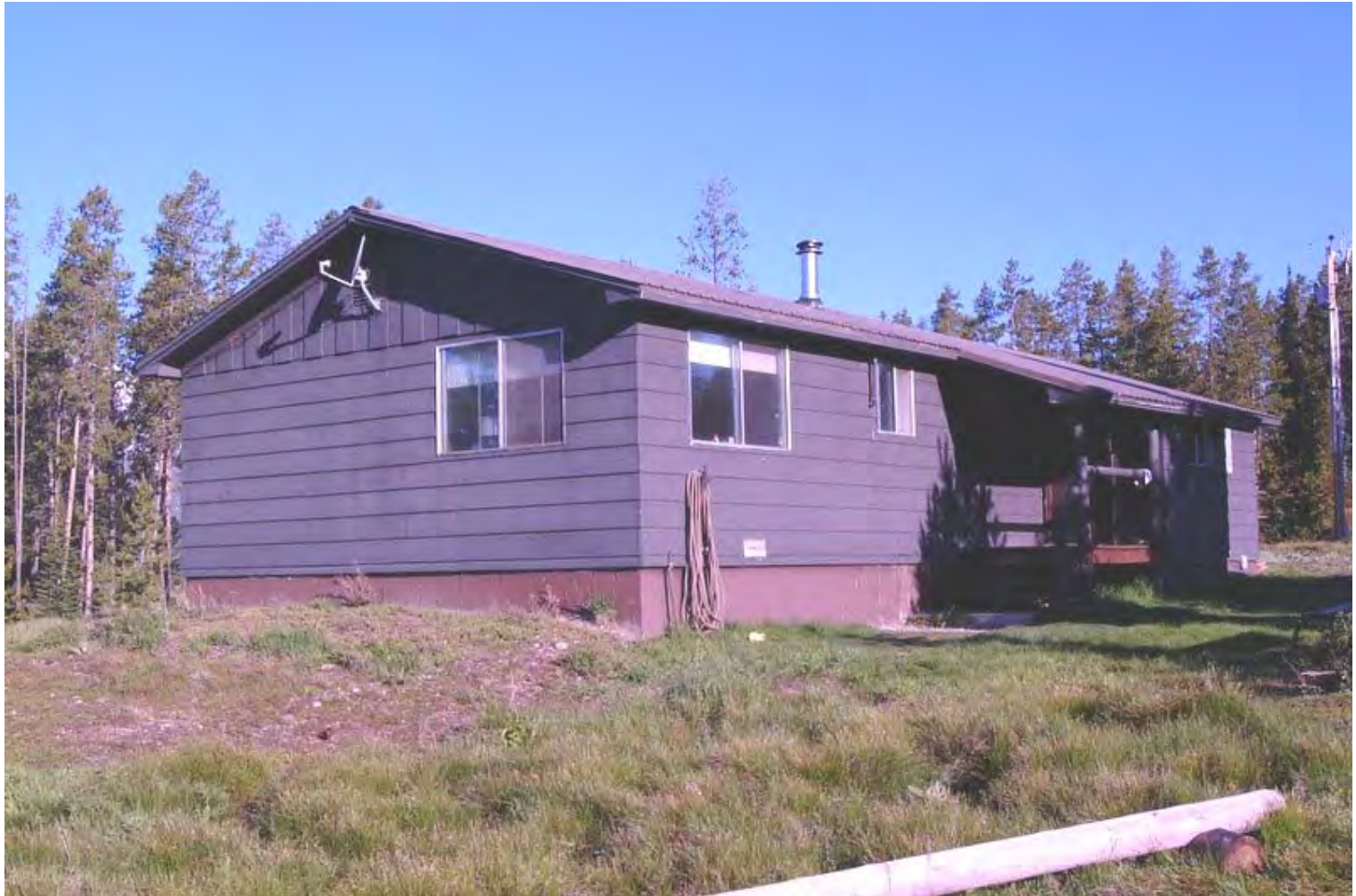
East-facing façade and south elevation
