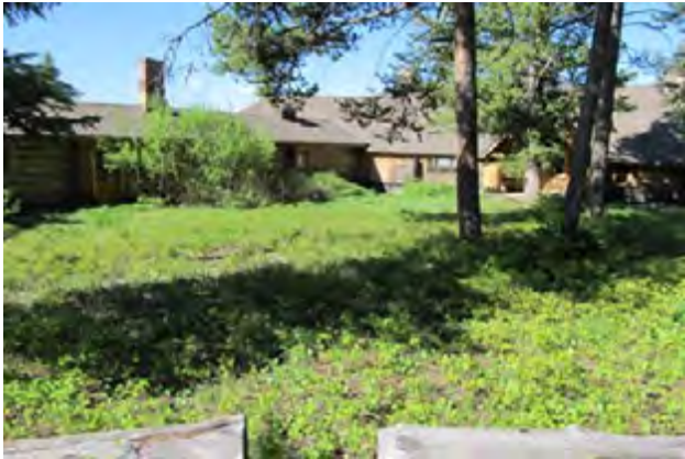
Water drains down hill directly under building
