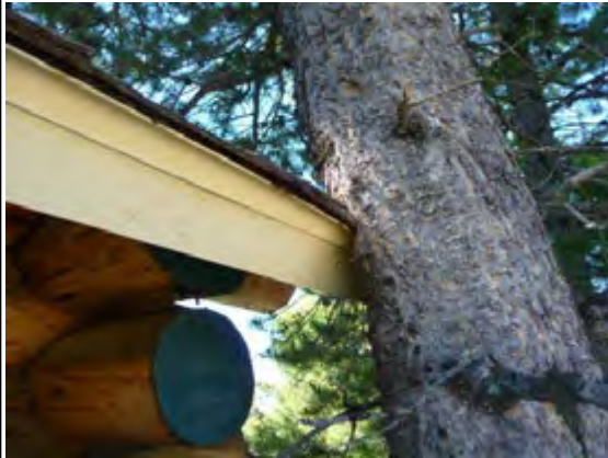
1. Tree at NW corner of roof
