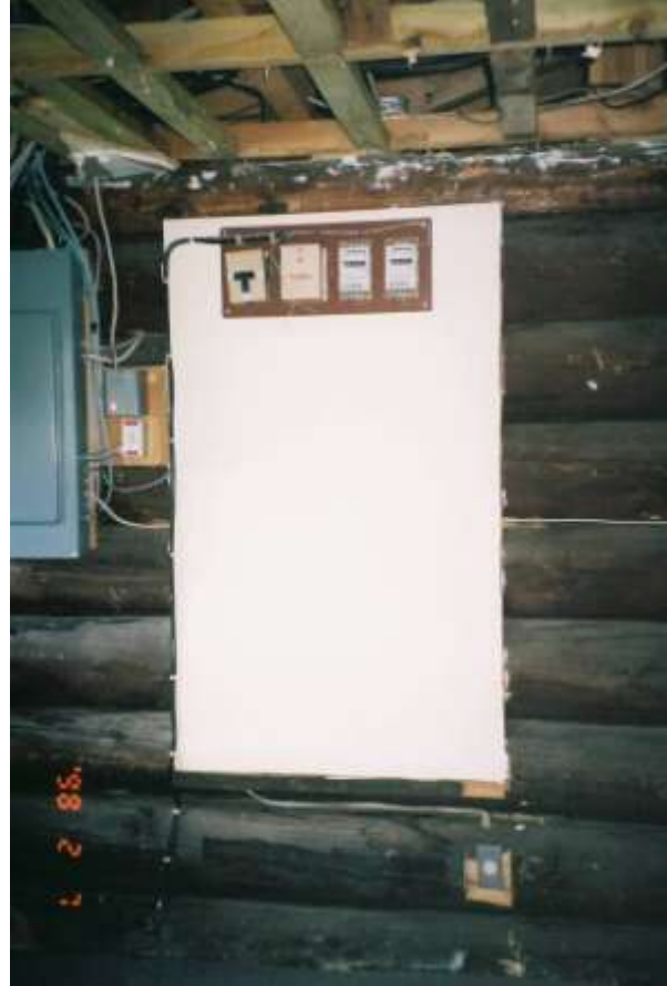
Interior room #10, electrical panel and other utilities
