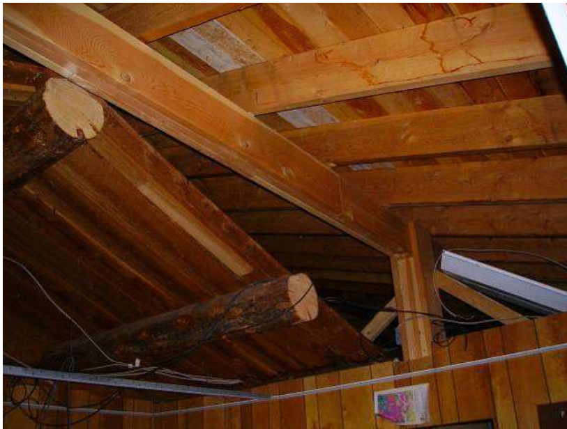
Figure 16 Roof framing visible in Rm. #11
