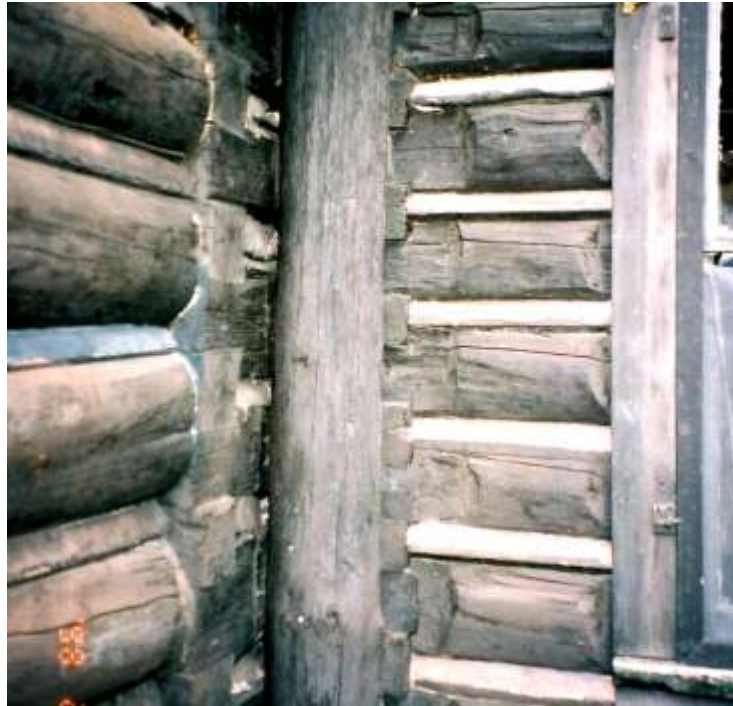
Figure 29 Joint of Rm. #1 and #13
