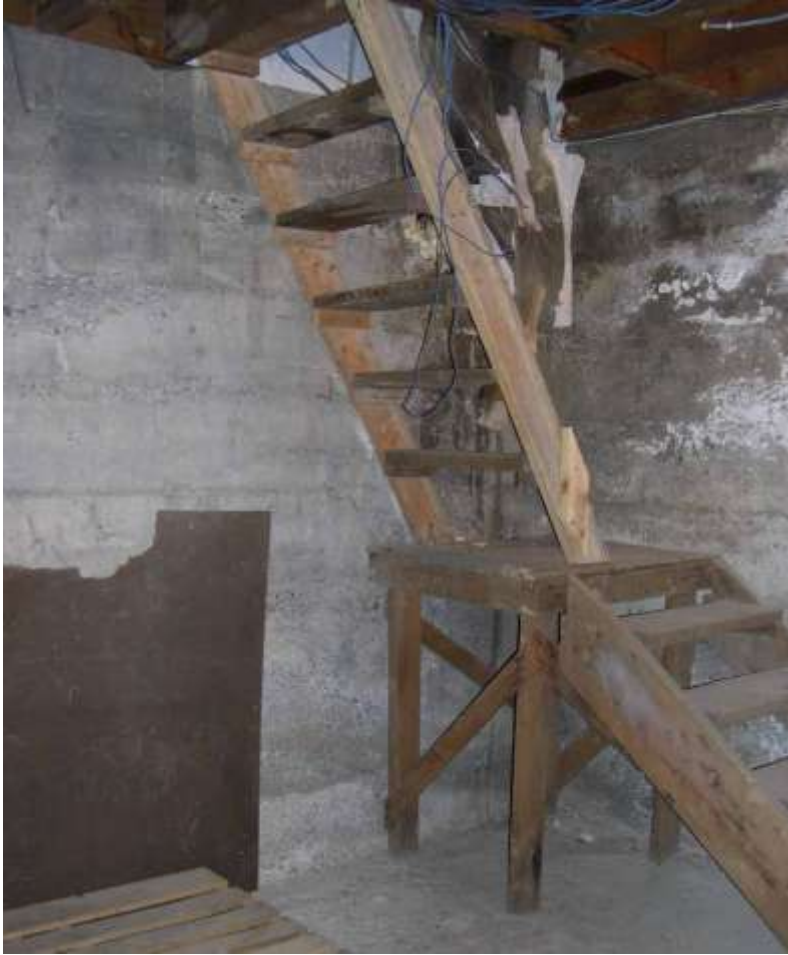
Figure 32 Basement stairs and interior basement walls
