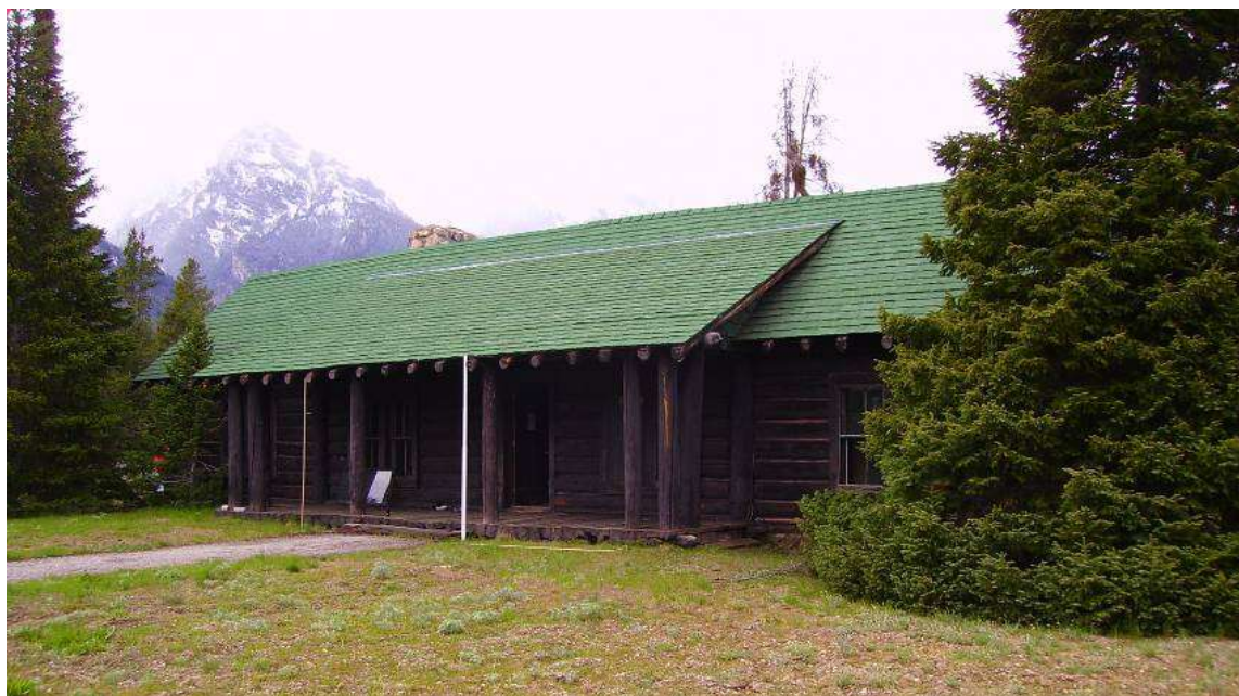
Figure 20 Current entrance with vegetation
