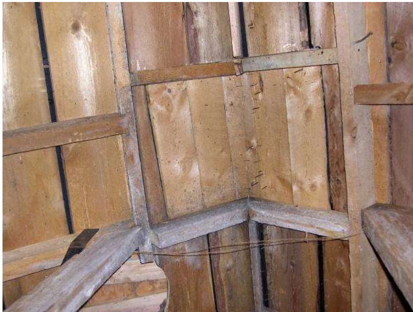
Figure 8 Rms. #3a and #4 with patch of chimney location
