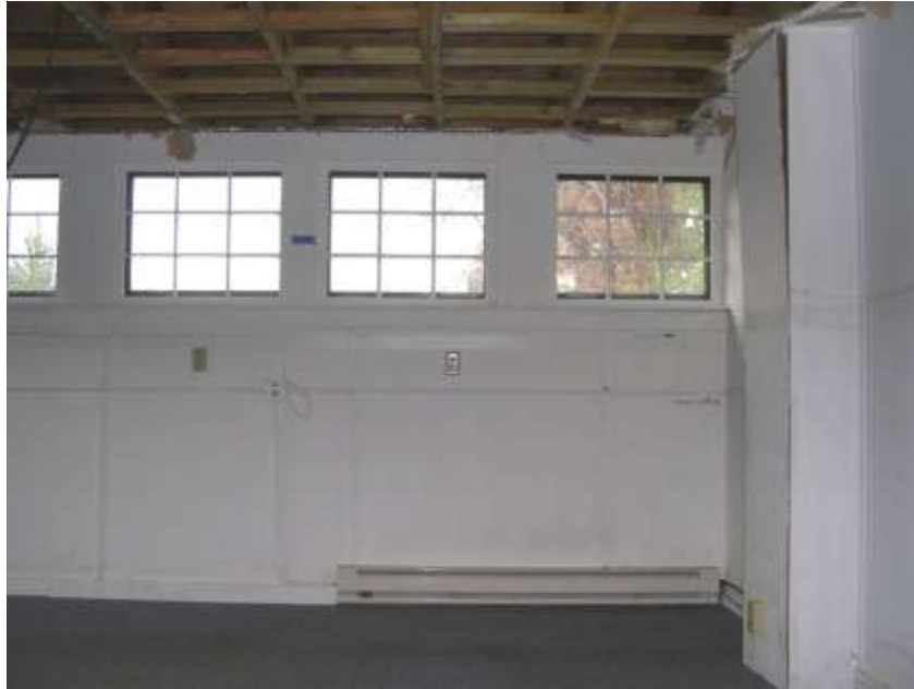
North wall of 1956 addition, windows and walls in overall good condition
