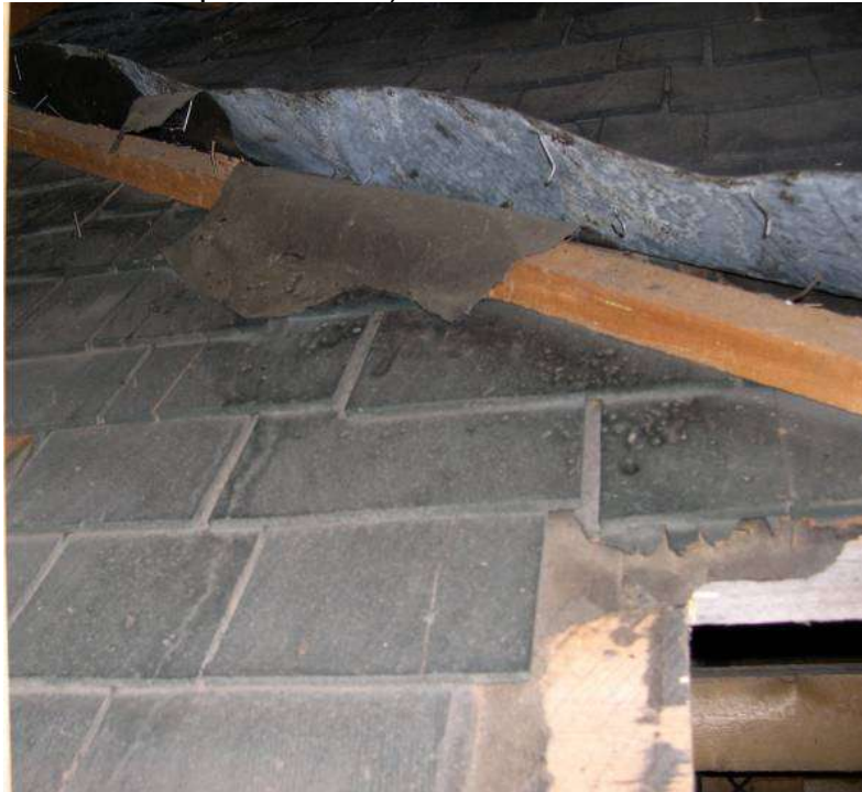
Figure 17 Space under 'new' hipped roof
