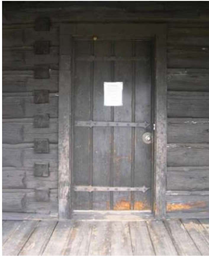
Front entry with wear on bottom right corner, otherwise in good condition, especially decorative hardware
