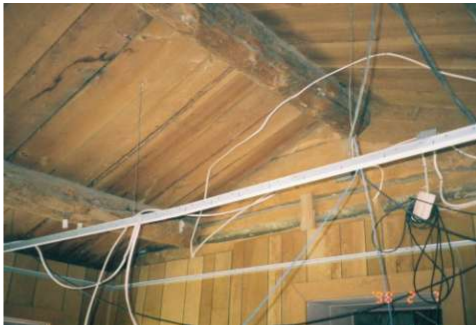
Junction of north wall of hipped roof and south wall of earliest addition
