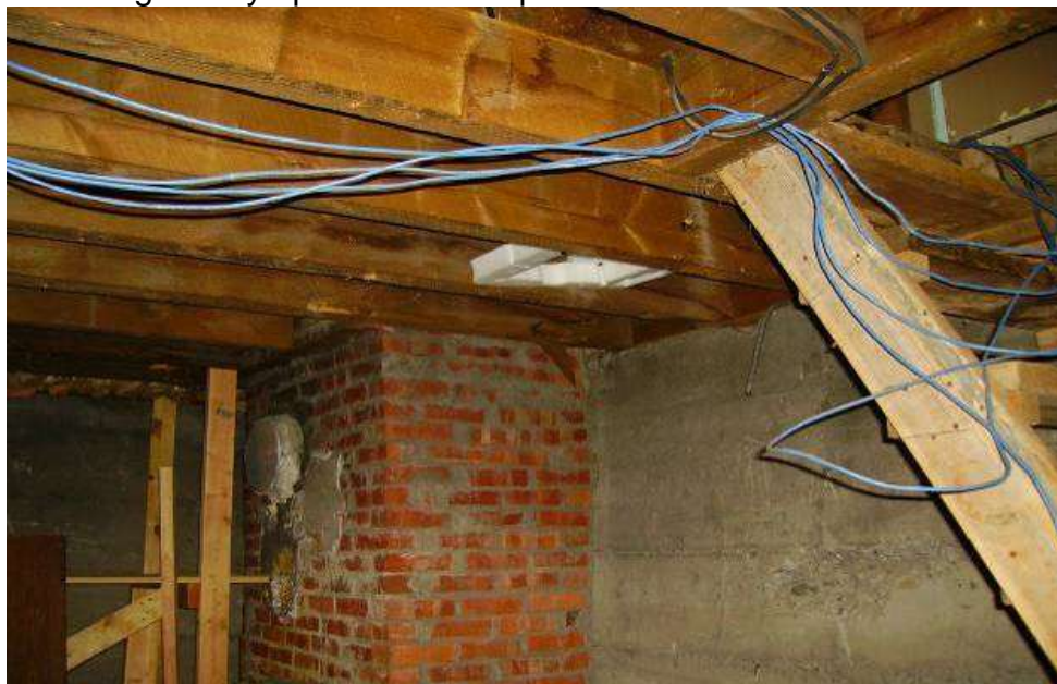
Figure 13 Basement under Rm. #5 showing chimney
