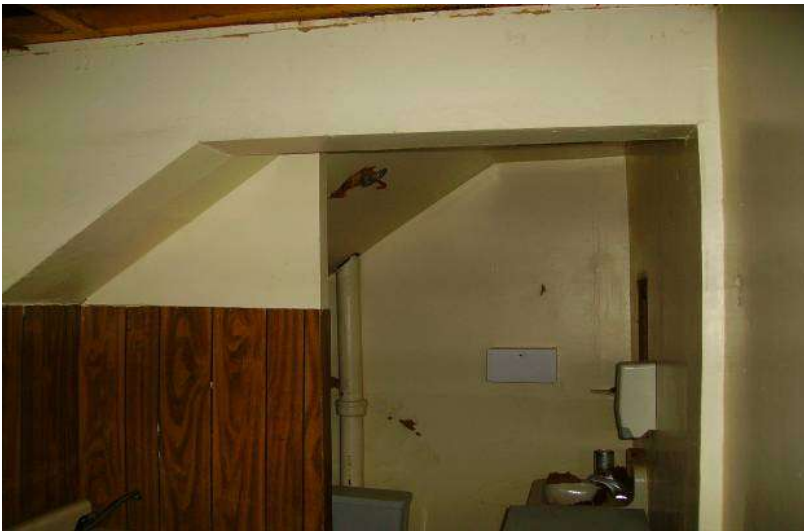
Figure 10 Rm. #8 showing evidence of lean-to roof
