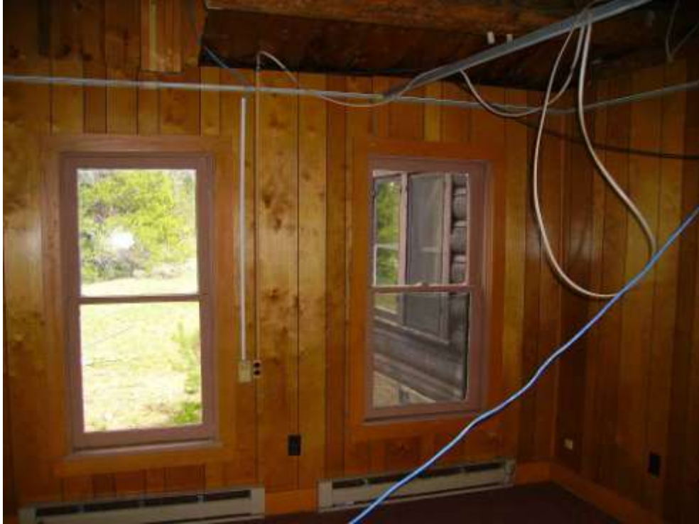
East wall of the earliest addition (room #13), windows in good condition
