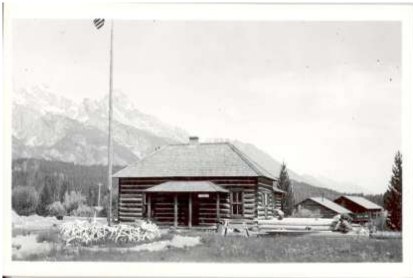
Figure 36 CCC construction of addition 1939
