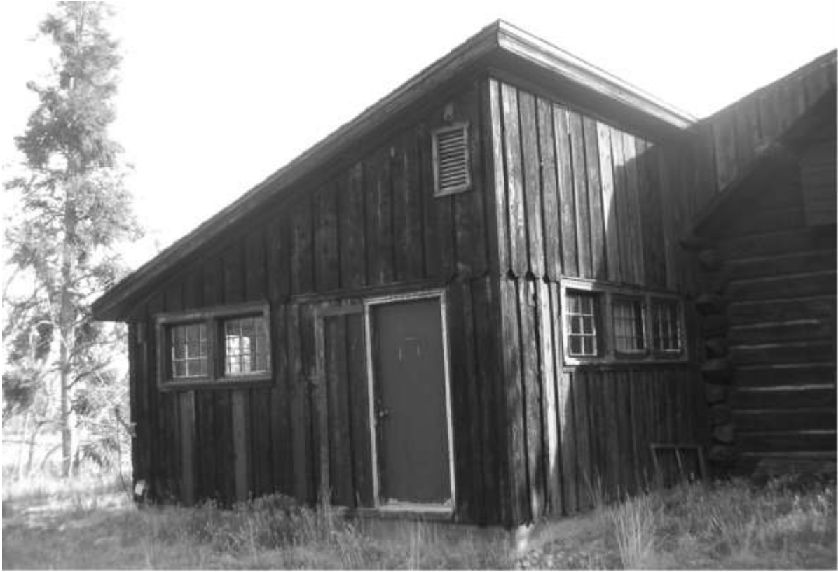
Figure 50 1956 addition from the southwest
