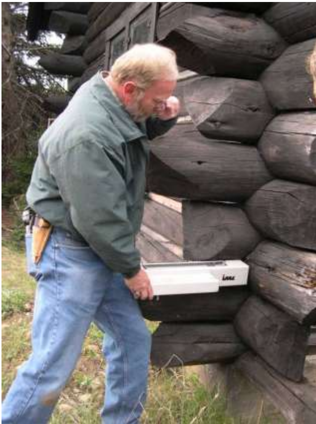
Figure 39 Resistance drill testing at east elevation 'beaver tail'
