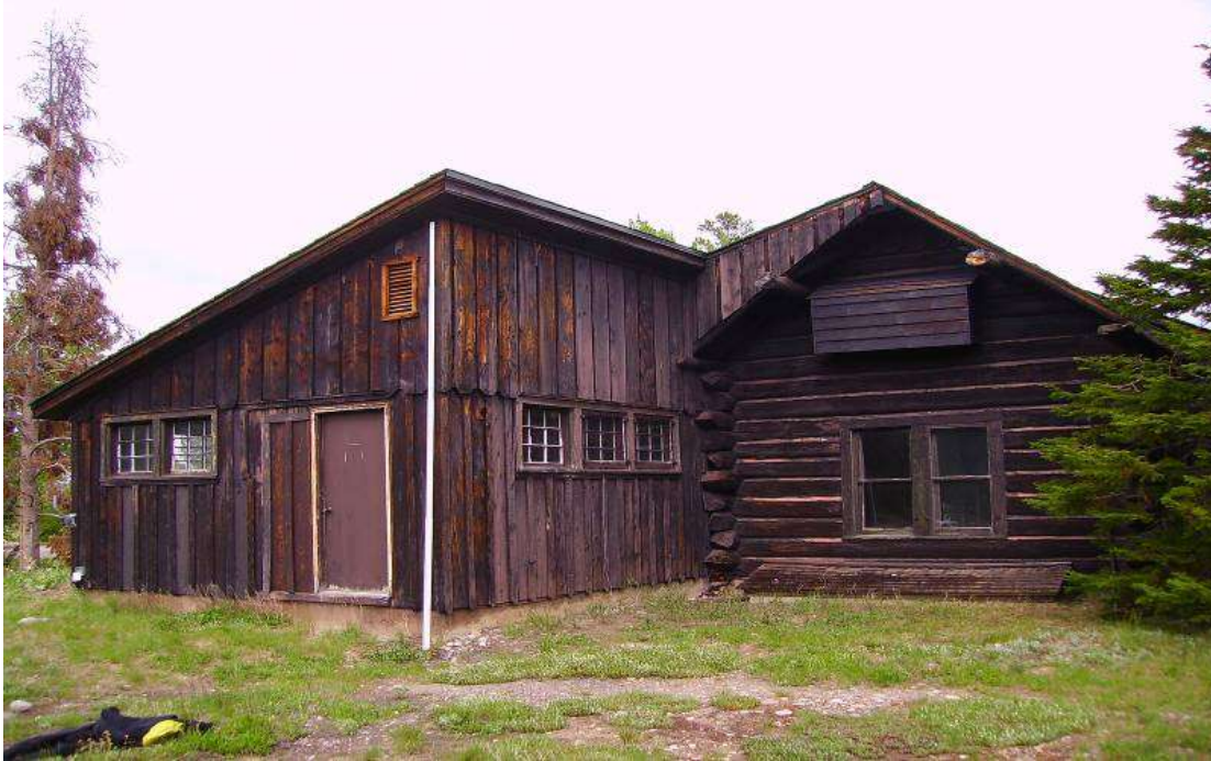
Figure 53 1956 addition at west elevation. Note bat habitat on gable end
