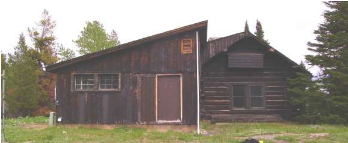
Figure 25 West elevation showing 1956 addition abutting 1939 addition
