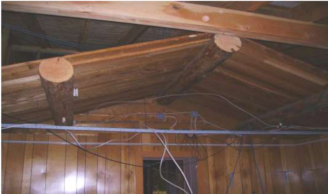
Figure 45 Exposed purlins and shed roof rafters above
