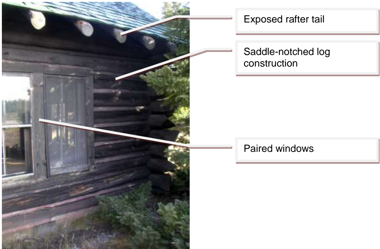
Figure 33 East side of south elevation
