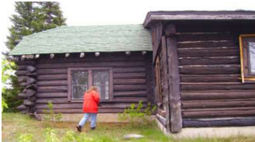
Figure 28 North elevation of Rm. #1
