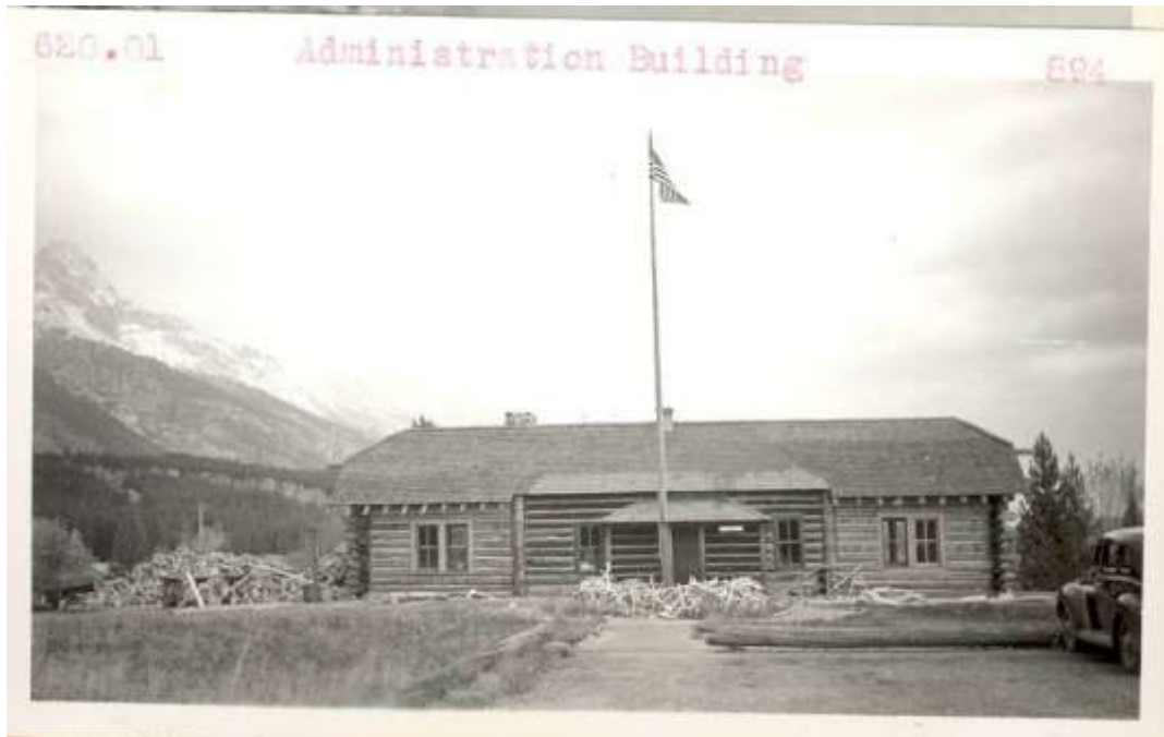
Figure 19 Archival photograph c. 1939
