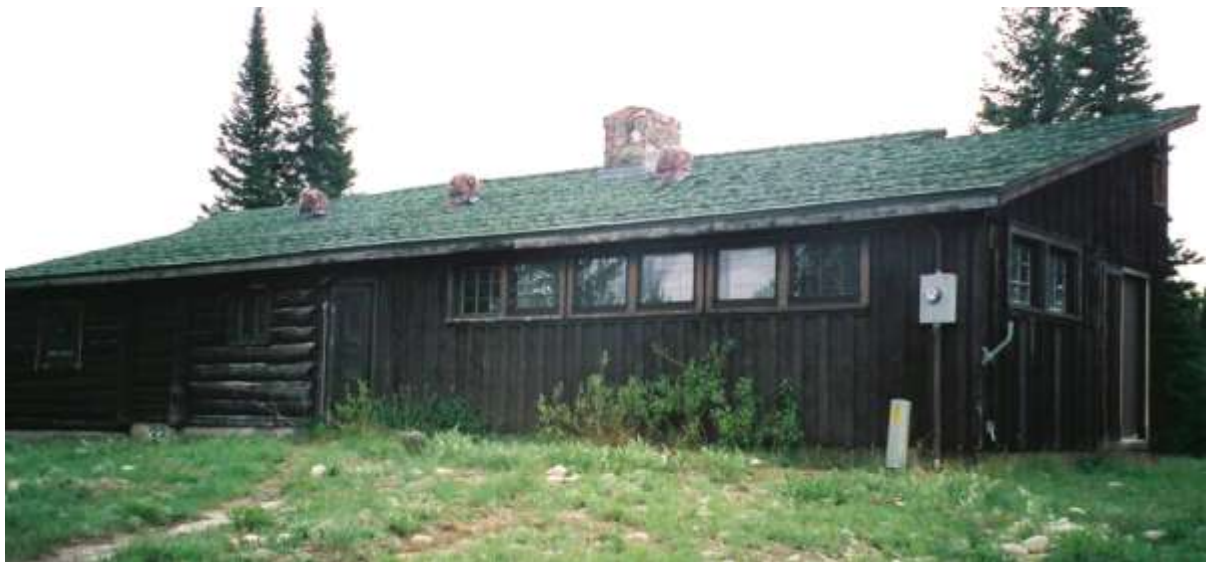
Figure 31 View from north showing eco-shake roof
