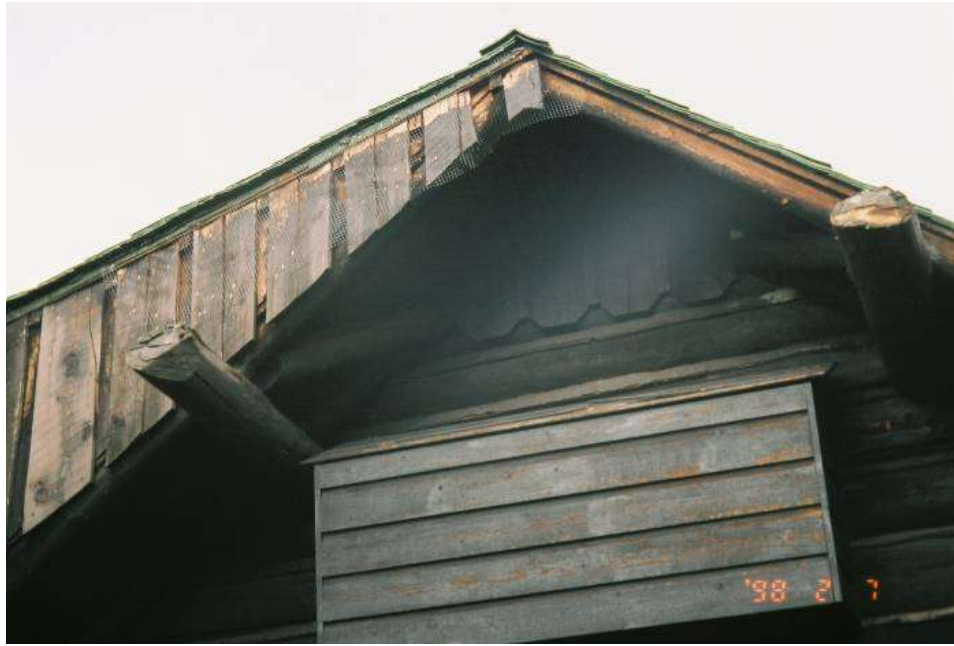
Figure 18 Detail of over roof
