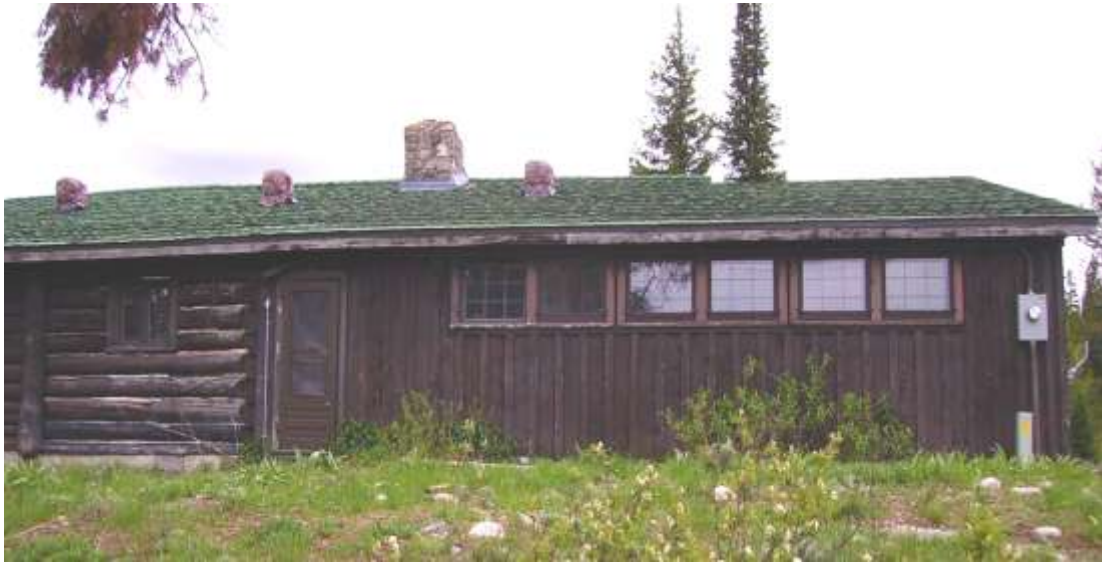
Figure 26 North elevation showing 1956 addition abutting earlier construction
