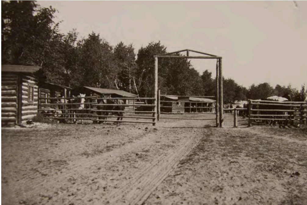
Camp Store and Entry Gate c. 1930 (North Facing)
