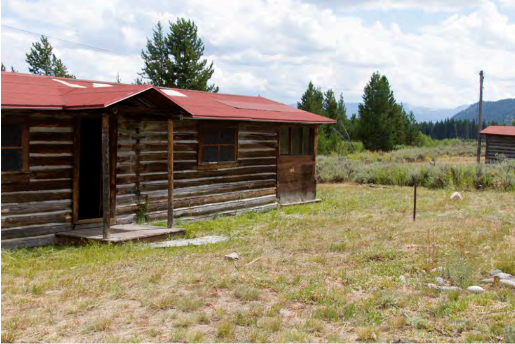
Cabin 1374 and Stone Ring 7/2015 (West Facing)
