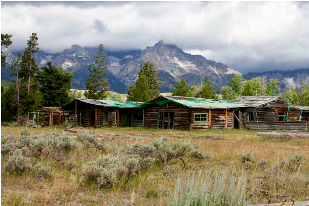
DRAFT Main Cabin 7/2015 (West Facing)
