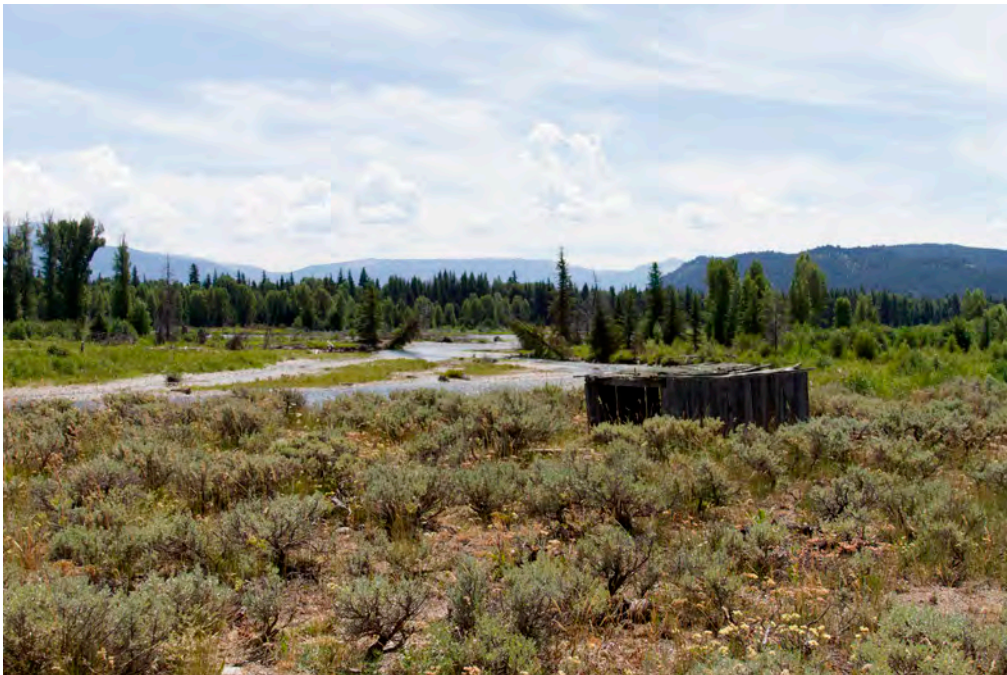
Skeet Shed 7/2015 (South Facing)
