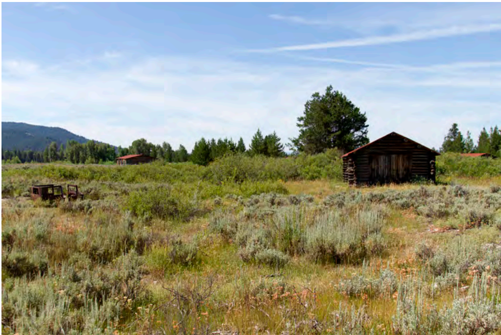
DRAFT Garage 1368 7/2015 (South Facing)
