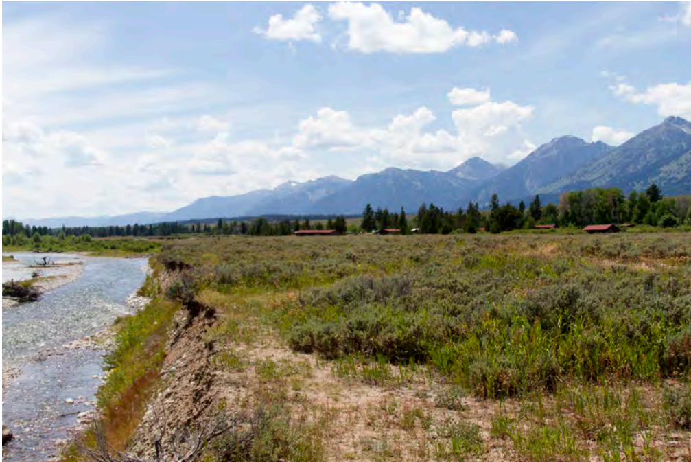
Snake River encroaching on Cabins 7/2015 (South Facing)
