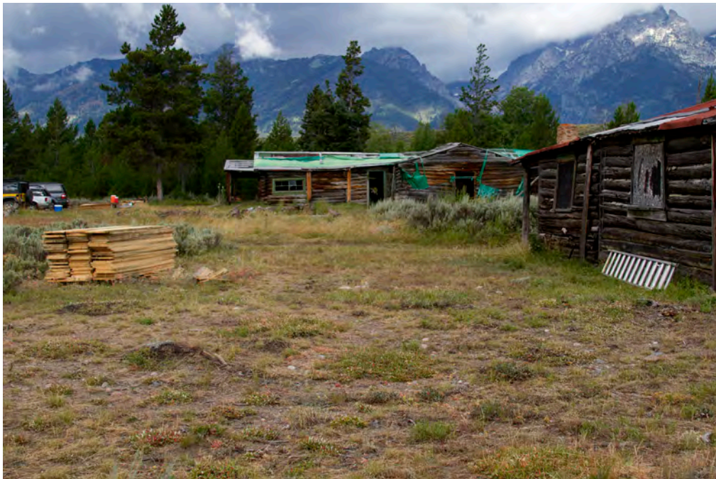
DRAFT Main Cabin 7/2015 (West Facing)
