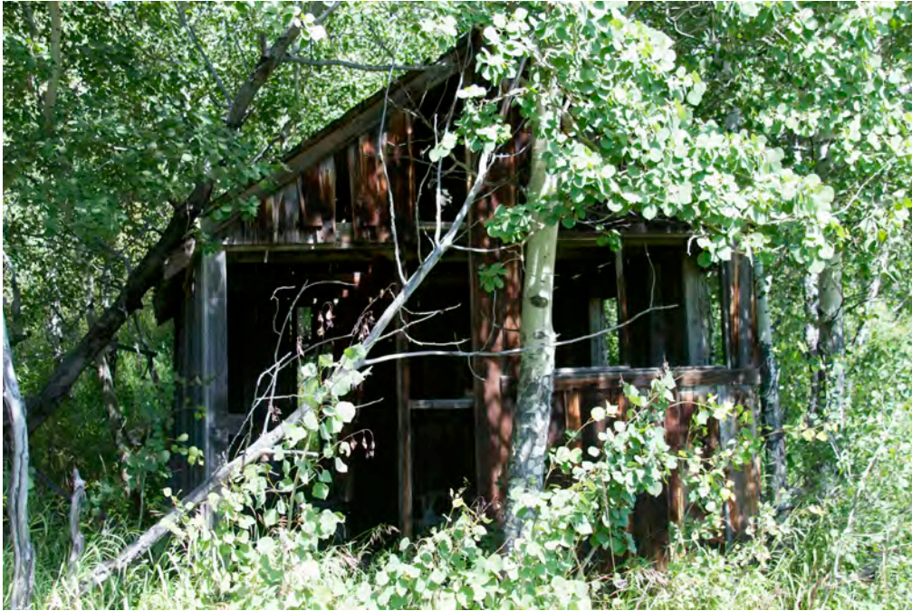
1401 Generator Shed 7/2015 (West Facing)
