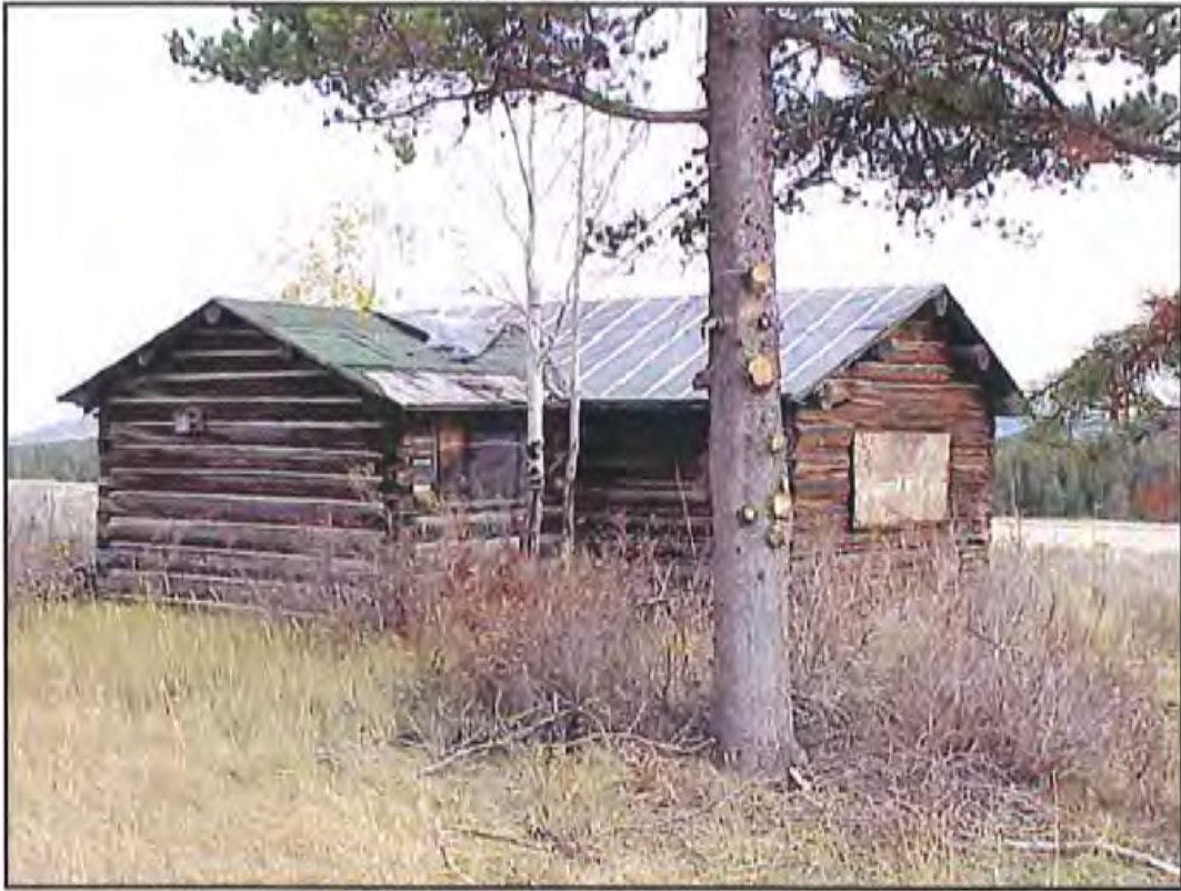
Figure 45. West and south walls of HS-1158, Cabin 10. Source: A&E Architects, 2004.
