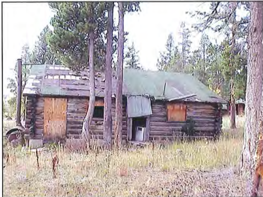
Figure 67. North wall of HS-1162, the Bathhouse. Source: A&E Architects, 2004.
