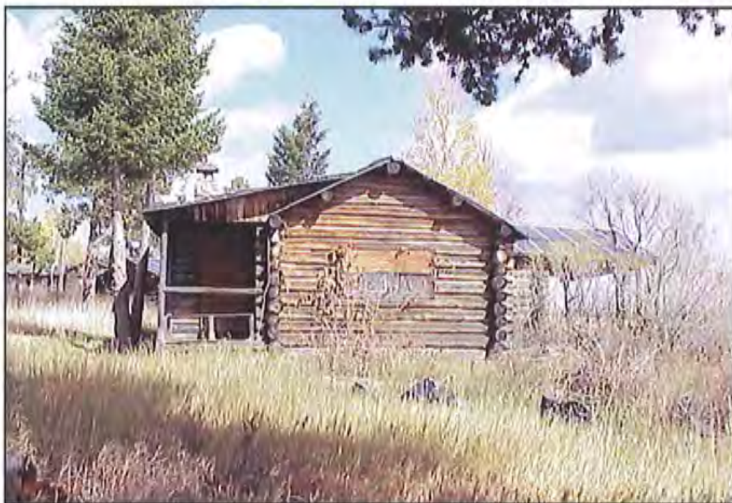
Figure 33. South wall of HS-1156, Hammond Cabin. Source: A&E Architects, 2004.
