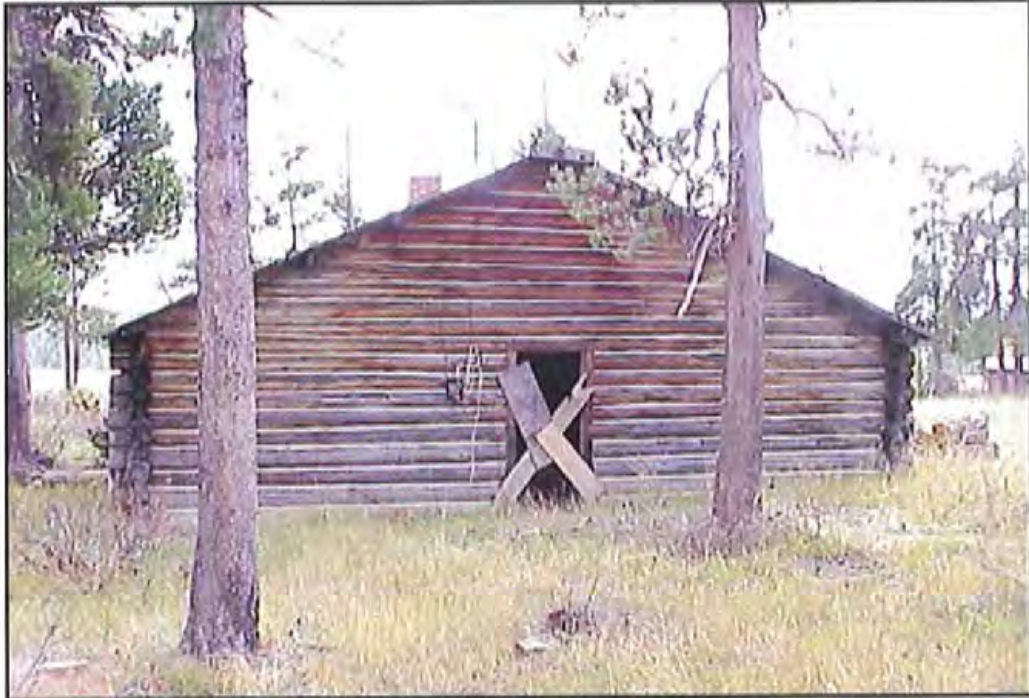
Figure 68. West wall of HS-1162, the Bathhouse. Source: A&E Architects, 2004.
