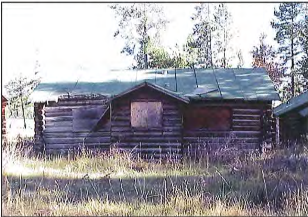
Figure 79. West wall of HS-1164, Cabin 6. Source: A&E Architects, 2004.
