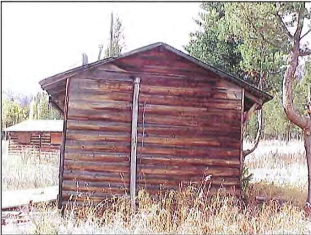
Figure 27. East wall of HS-1155, Cabin 15. Source: A&E Architects, 2004.
