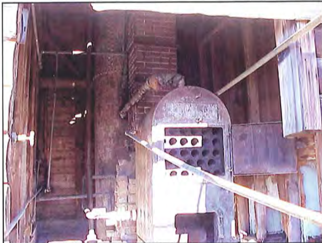
Figure 69. Interior of the east room of HS-1162, the Bathhouse. Source: A&E Architects, 2004.
