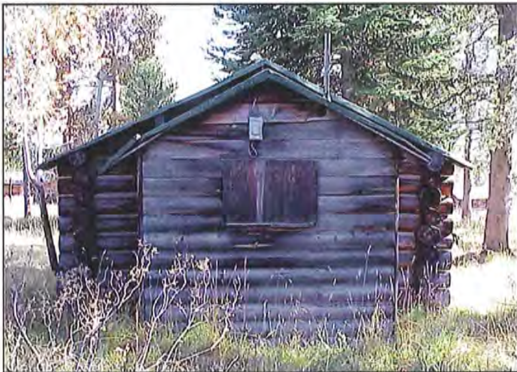
Figure 85. West wall of HS-1165, Cabin 5. Source: A&E Architects, 2004.
