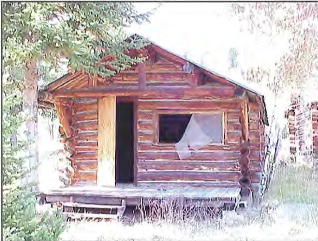
Figure 83. East wall of HS-1165, Cabin 5. Source: A&E Architects, 2004.
