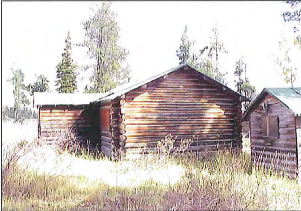
Figure 80. South wall of HS-1164, Cabin 6. Source: A&E Architects, 2004.
