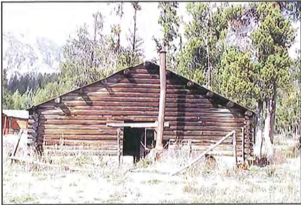
Figure 66. East wall of HS-1162, the Bathhouse. Source: A&E Architects, 2004.
