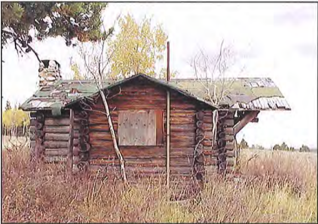
Figure 51. South wall of HS-1159, Cabin 9. Source: A&E Architects, 2004.
