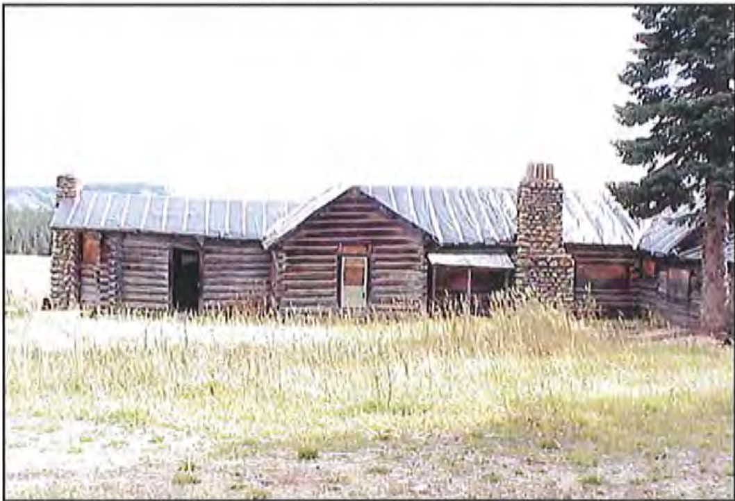
Figure 90. West wall of HS-1168, the Main Cabin. Source: A&E Architects, 2004.
