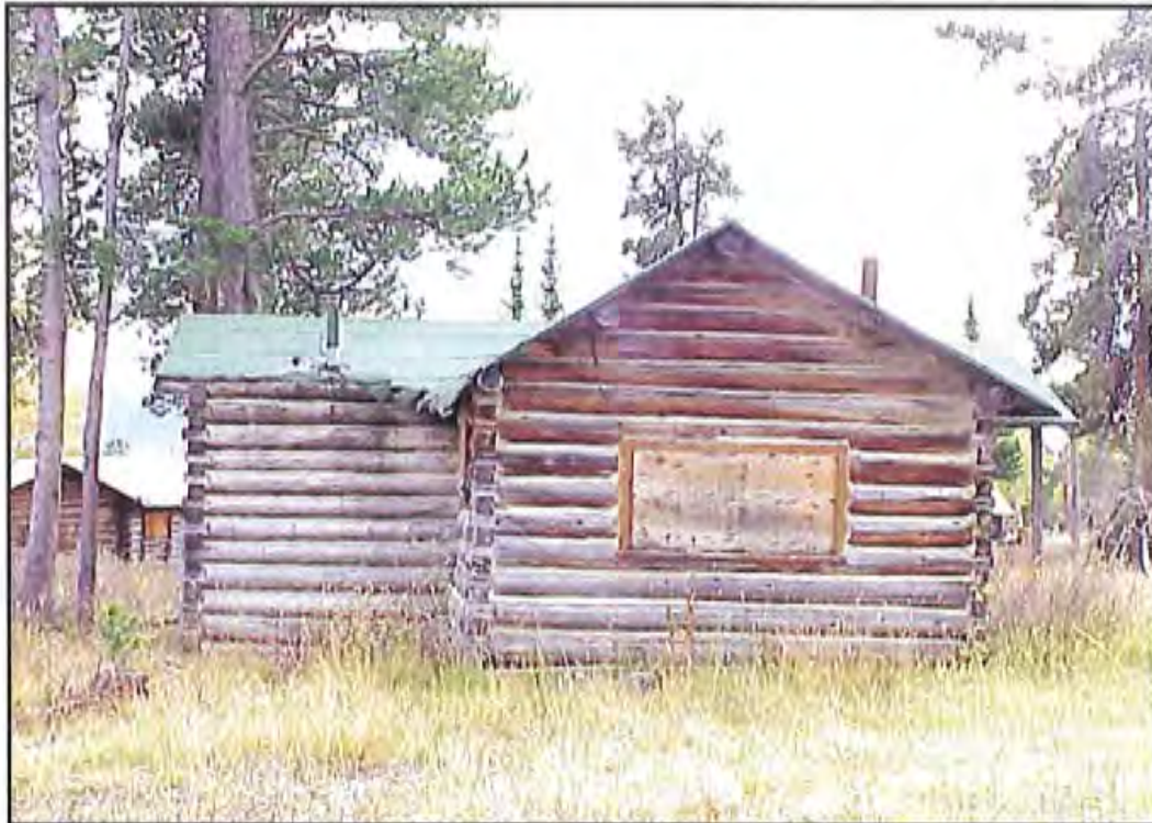
Figure 62. North wall of HS-1161, Cabin 11. Source: A&E Architects, 2004.
