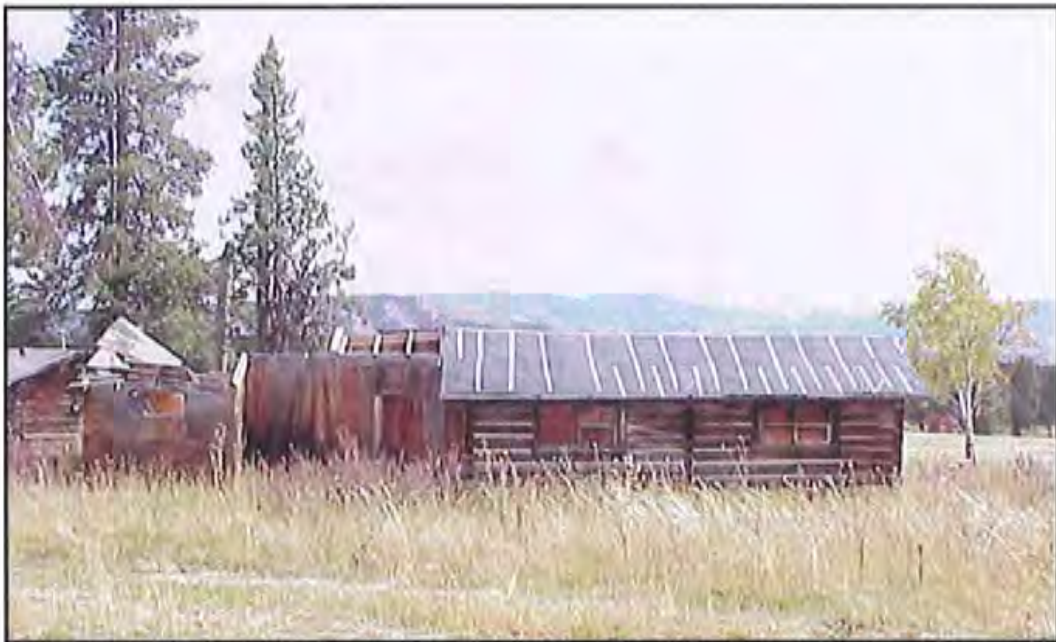
Figure 22. Looking east to the west wall of HS-1154, Girls' Cabin. Source: A&E Architects, 2004.
