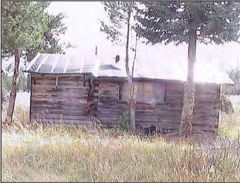
Figure 26. North wall of HS-1155, Cabin 15. Source: A&E Architects, 2004.
