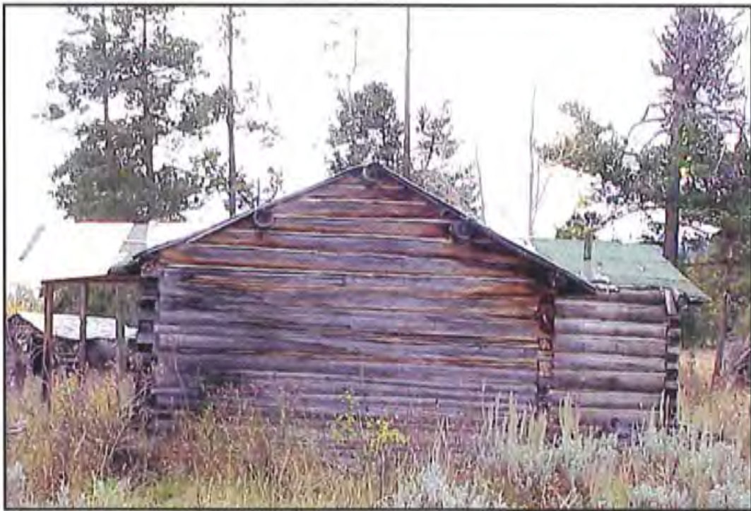
Figure 46. North wall of HS-1158, Cabin 10. Source: A&E Architects, 2004.
