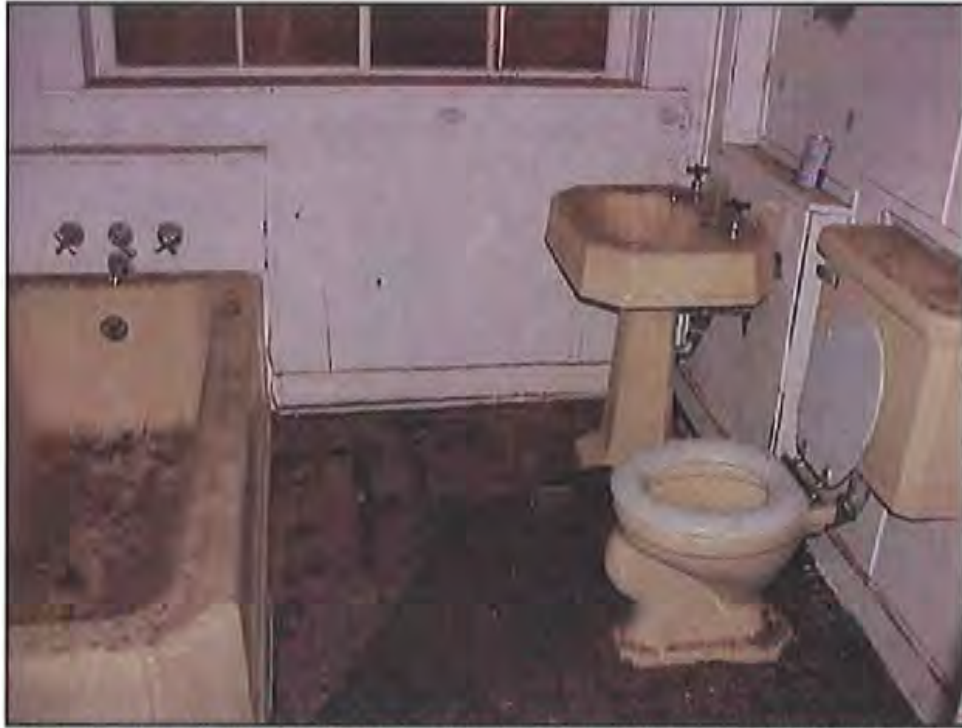
Figure 36. Detail of the interior of one of the bathroom additions, HS-1156, Hammond Cabin. Source: A&E Architects, 2004.
