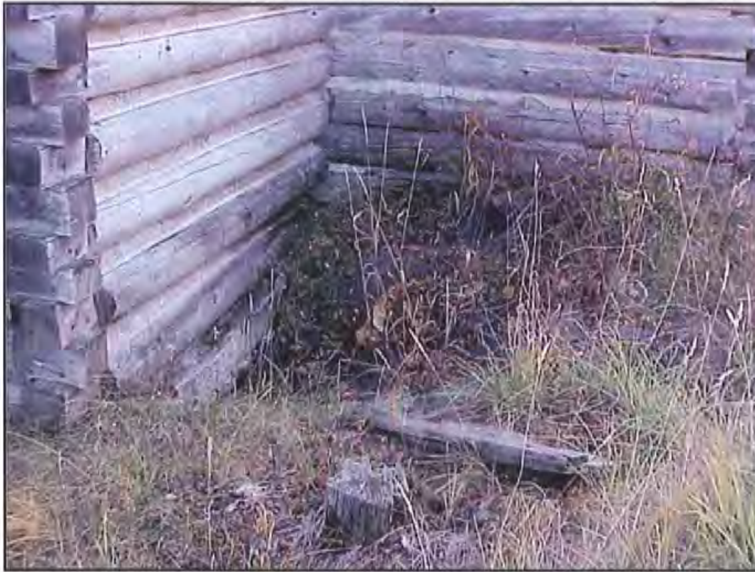
Figure 63. Detail of the junction of the addition (left) and the main volume (right), showing differences in daubing. Source: A&E Architects, 2004.
