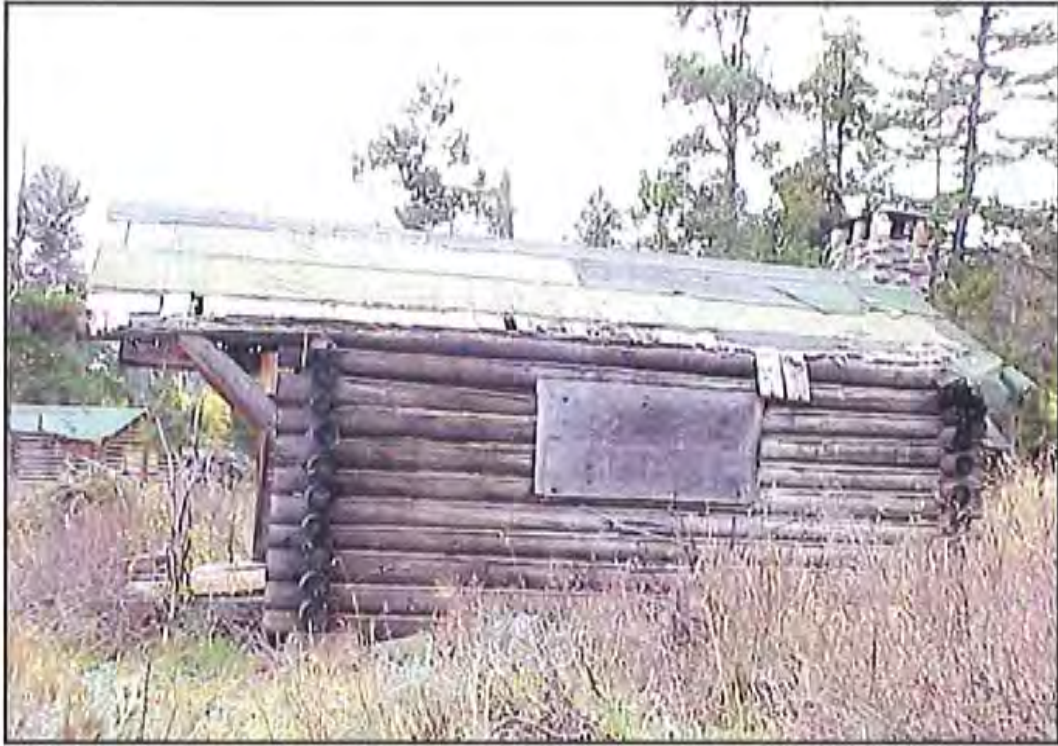
Figure 50. North wall of HS-1159, Cabin 9. Source: A&E Architects, 2004.
