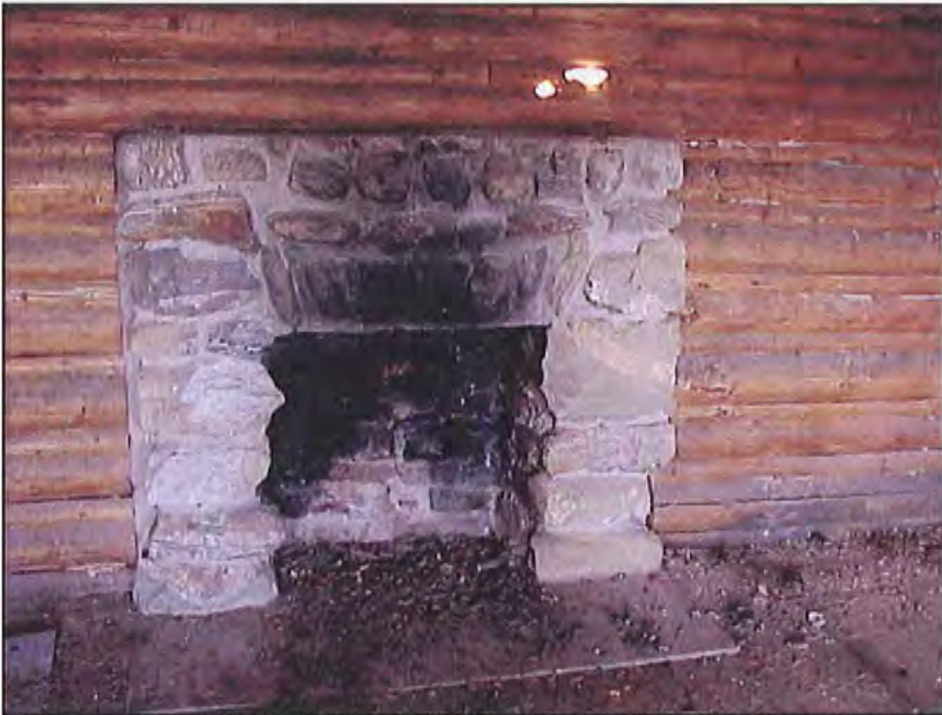
Figure 53. Interior fireplace, rear (west) wall of HS-1159, Cabin 9. Source: A&E Architects, 2004.
