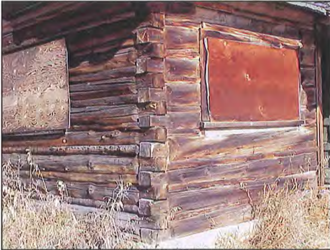
Figure 47. Detail of the southeast corner of HS-1158, Cabin 10. Source: A&E Architects, 2004.
