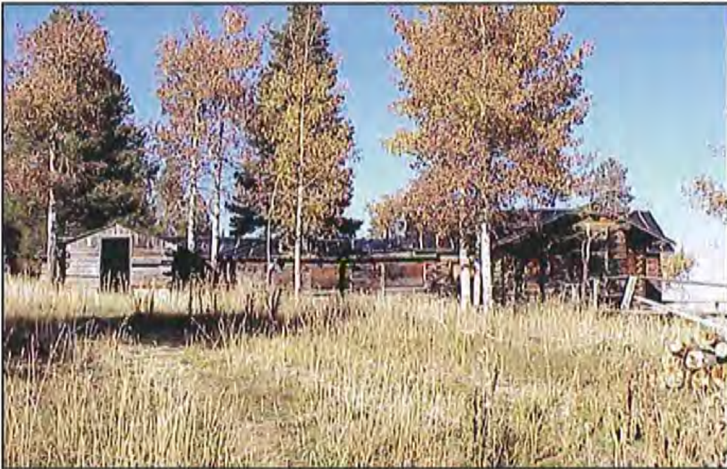
Figure 92. South wall of the west wing, original volume and south addition, HS-1168, the Main Cabin. Source: A&E Architects, 2004.
