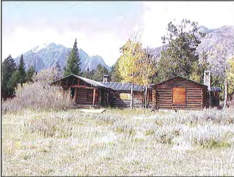
Figure 30. Front (east) wall of HS-1156, Hammond Cabin. The open porch visible at the south end of the building is part of the original building. Everything north of the porch is an addition. Source: A&E Architects, 2004.
