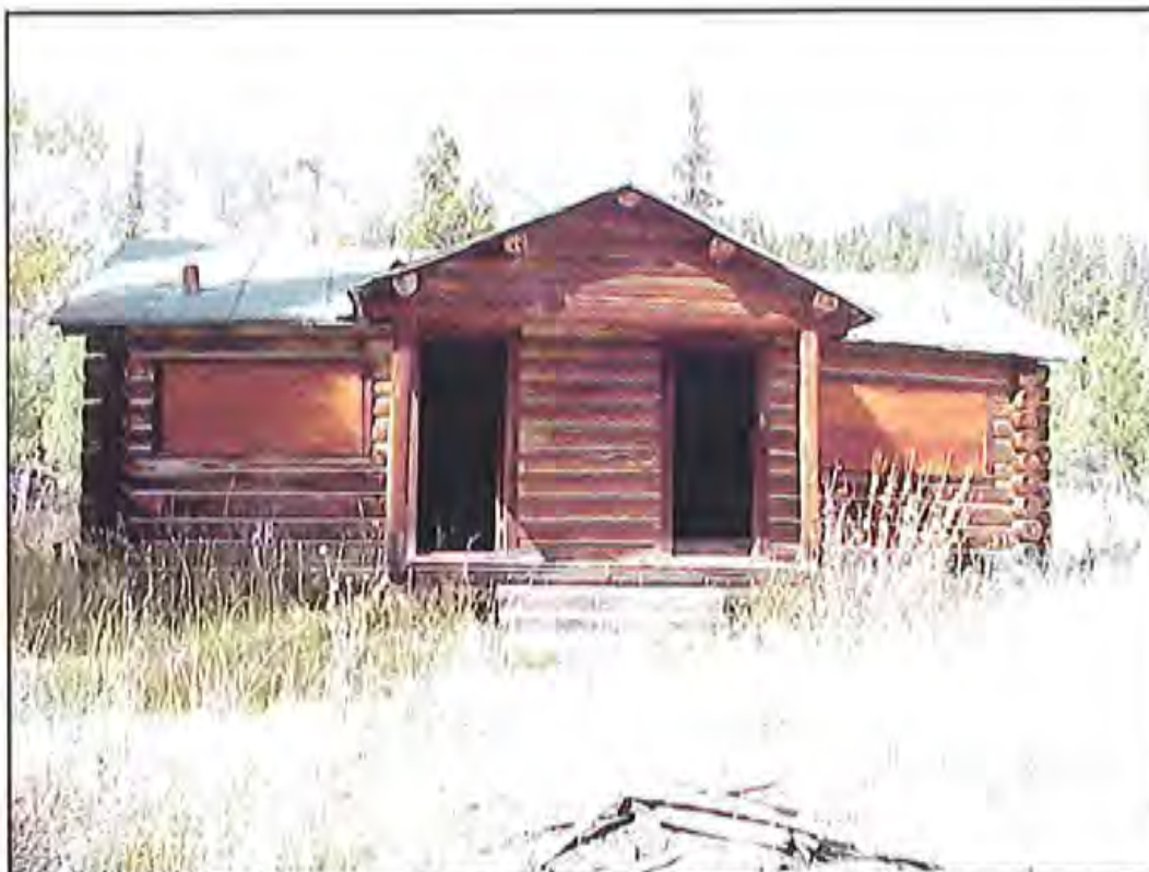
Figure 77. East (front) wall of HS-1164, Cabin 6. Source: A&E Architects, 2004.
