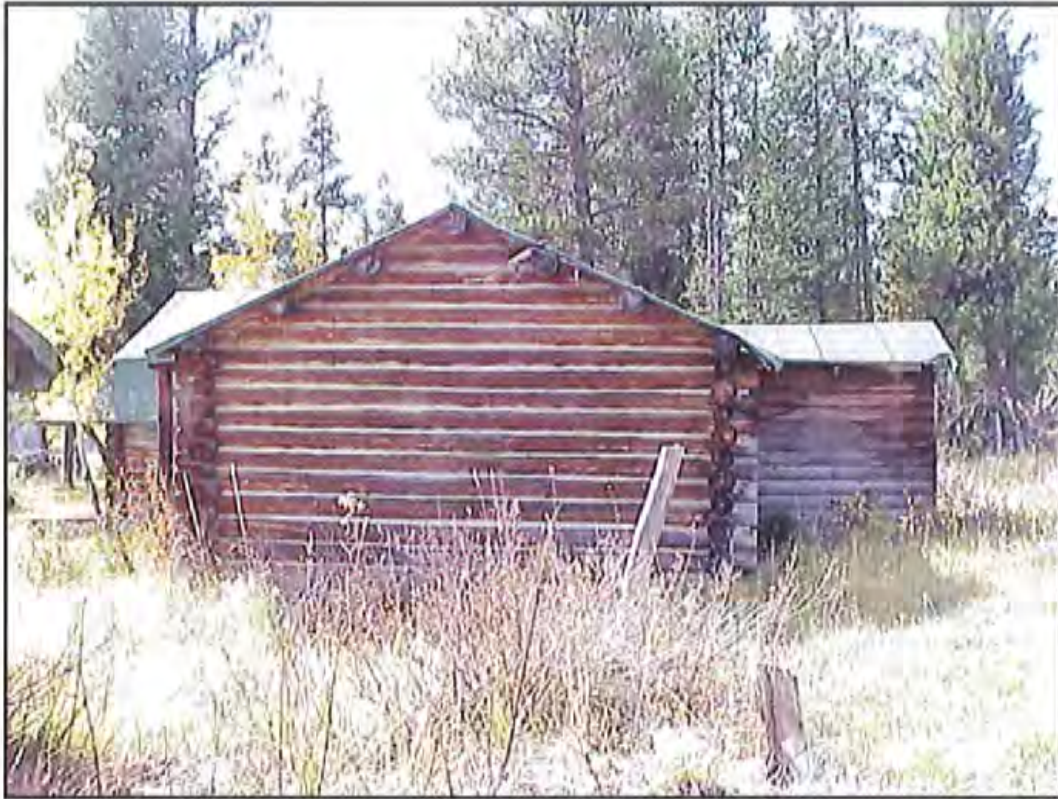
Figure 78. North wall of HS-1164, Cabin 6. Source: A&E Architects, 2004.
