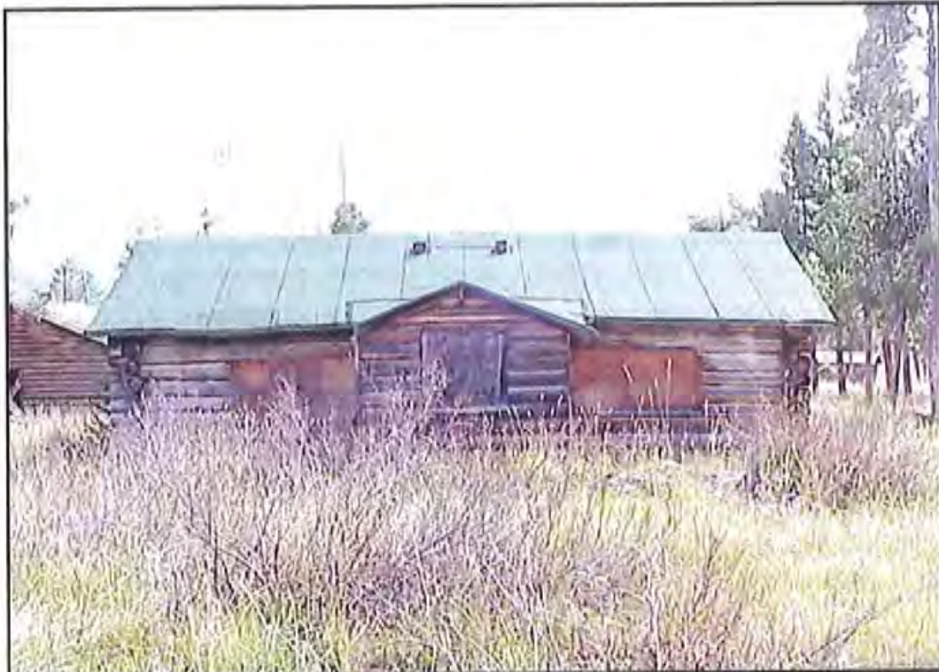
Figure 73. West (rear) wall of HS-1163, Cabin 7. Source: A&E Architects, 2004.
