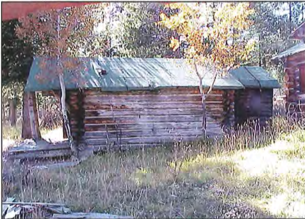
Figure 84. North wall of HS-1165, Cabin 5. Source: A&E Architects, 2004.
