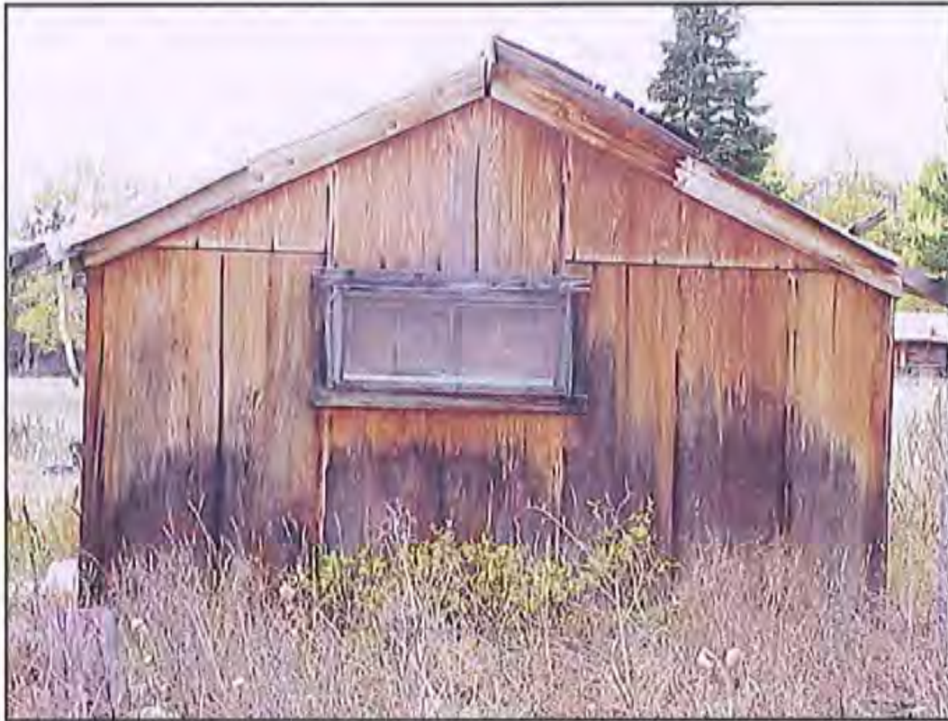
Figure 23. North wall of the addition HS-1154, Girls' Cabin. Source: A&E Architects, 2004.
