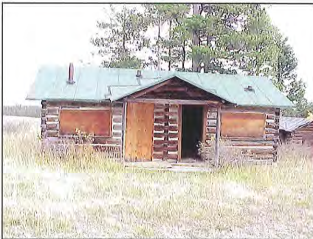
Figure 60. West (front) wall of HS-1161, Cabin 11. Source: A&E Architects, 2004.
