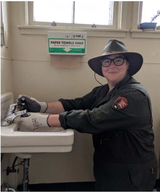
NPS staff replaces aerator
