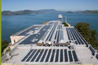
Solar panels at Alcatraz
