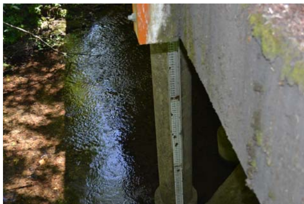
Staff plate at Muir Woods Road Bridge
