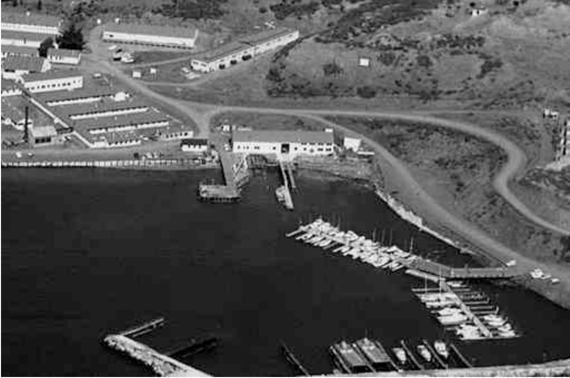
Presidio Yacht Club c1963. Windows have been enlarged in the bar and dining room. The 100-ton marine railway tracks remain but the cradle is gone. Floating piers extend out from the former Angel Island ferry dock (Bldg 669) at lower right. (PYC Collection)
