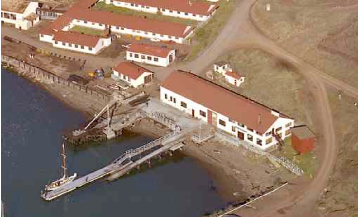
Presidio Yacht Club c1975. The truncated Repair Dock and its 10-ton derrick are at left. Note how the opening for the former 100-ton way has been planked over. The flat-roofed telephone cable building is clearly visible at right. (Golden Gate NRA, PARC, GOGA 35301-0903)
