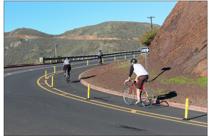
Recent changes to Conzelman Road include creating a one-way flow for cars downhill, adding parking, and creating a wider, protected uphill bike lane
