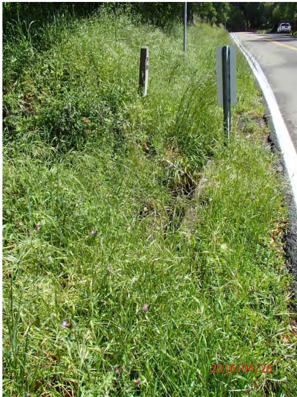
Photos 14 and 15. Photos taken of the hydrologically connected road and inboard ditch draining to stream crossing inlet at Site #159. Note that ditches are well vegetated, which promotes filtration of road surface runoff (sediment and pollutants).
