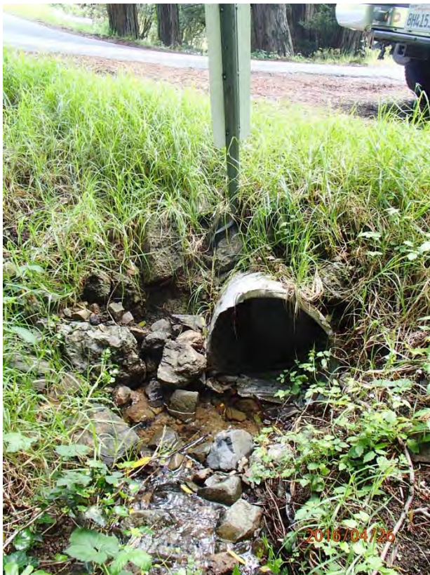
Photos 4 and 5. Photos taken of stream crossing Site #79. Photo 4 (left) taken upstream of the 20” diameter CMP inlet. Photo 5 (right) taken downstream of the CMP outlet. This 5’ x 1.5’ class 2 stream flows through an undersized culvert set shallow in the fill with a high plug potential. PWA recommends replacing this culvert with a properly sized and installed culvert.
