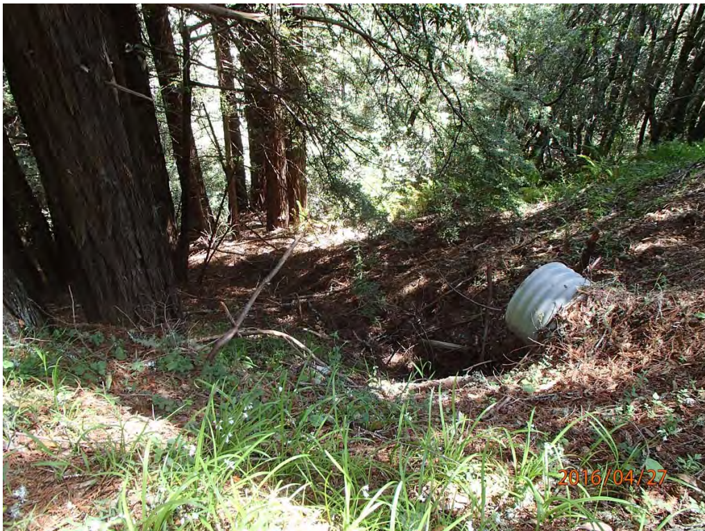
Photo 19. Photo taken from outboard edge of road looking downslope at the outlet of DRC Site #127. Note that the existing gully below the DRC outlet is stable and covered with duff.
