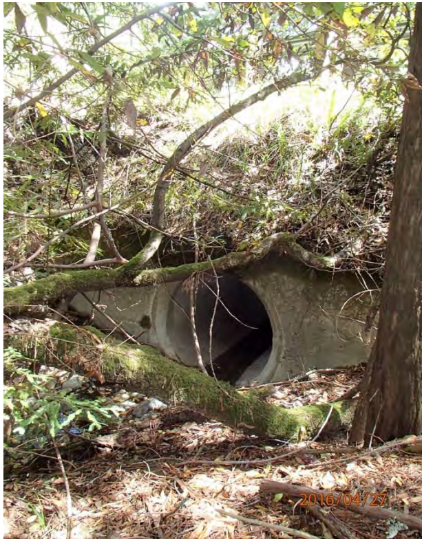
Photos 24 and 25. Photos taken from upstream looking at the stream crossing inlets at Site #140 (left) and #141 (right). The culvert at Site #141 is undersized; therefore, we recommend installing an overflow pipe and excavating material between Sites #140 and #141 for additional protection against diversion.
