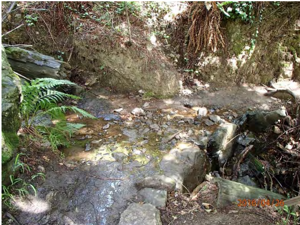
Photos 2 and 3. Photos taken from the left and right road approaches 5 (top and bottom photos, respectively) looking at where Site #78 hits the armored trail crossing. Note the outlet of DRC Sites #77, 78, and 80 all deliver to stream crossing Site #79.
