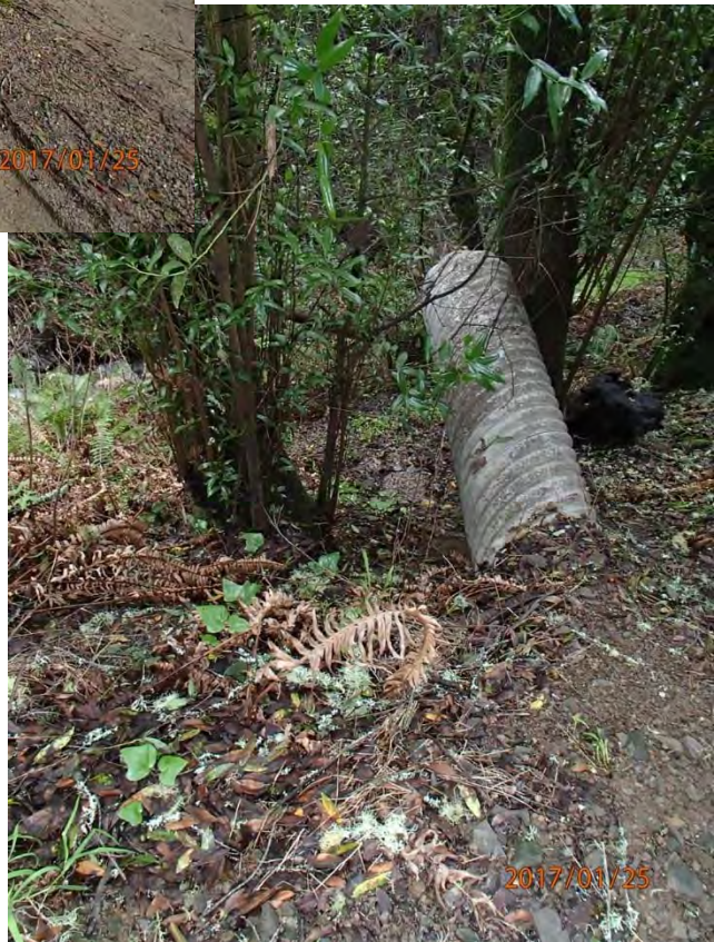
Photos 49 and 50. Photos taken of DRC Site #184. An 18” diameter DRC drains the connected right road approach and springy cutbank (left). The DRC is 30% plugged and is installed at a shallow grade, and the outlet is shot-gunned with a 5’ drop at the outlet (below).
