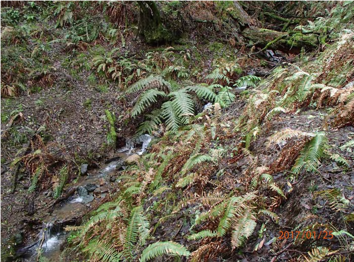
Photo 67. Photo taken of stream crossing Site #194. The road and stream crossing was decommissioned by NPS in 2003 when remaining fill was excavated from the crossing. Currently, stream appears to be stable.
