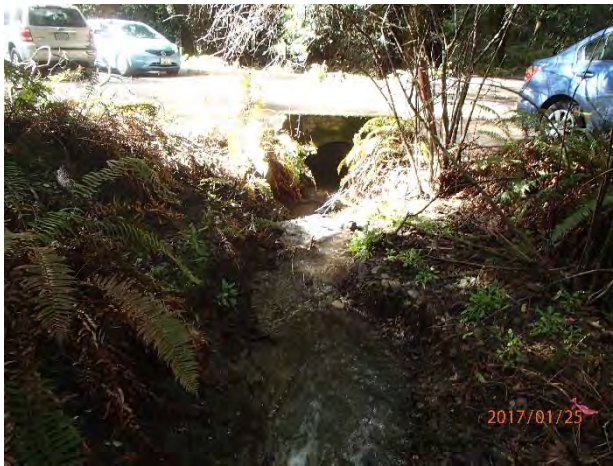
Photos 8 and 9. Photos taken at stream crossing Site #92. The stream is carried through an oval 41" wide by 30" tall culvert. Photo 8 (left) is taken from above the inlet of the culvert looking downstream. Photo on the left is view looking upstream at the outlet.
