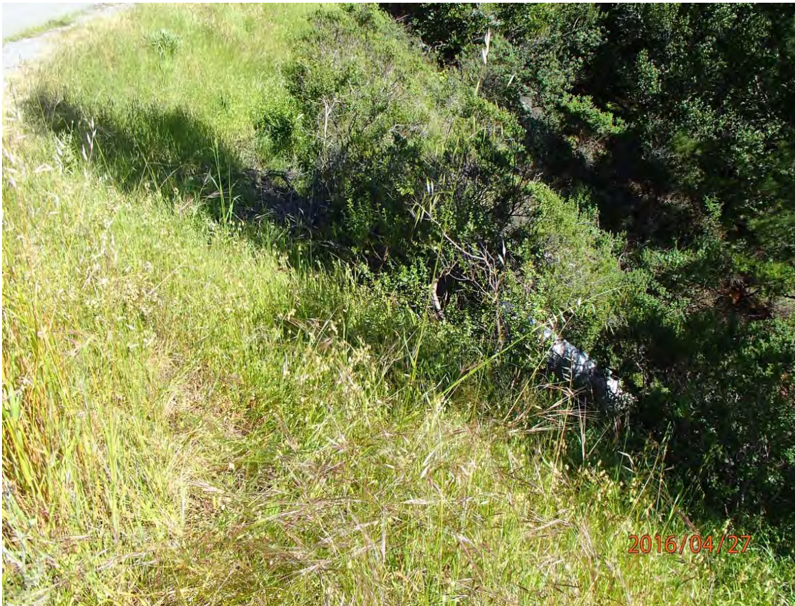
Photo 17. Photo taken of DRC Site #118 view of recently installed full round downspout attached to outlet to protect the fillslopes from further gullyng.
