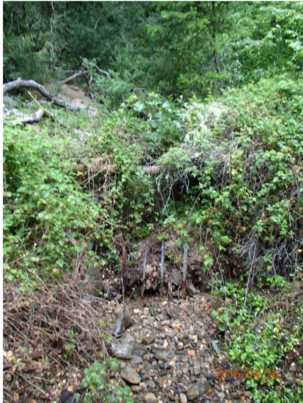
Photos 12 and 13. Photos taken at complicated stream crossing Site #94. Photo 12 (left) is taken from the inlet of the uppermost culvert looking upstream. The stream is carried through an undersized 24” diameter culvert from this point where the stream valley becomes buried by buildings, parking lot, and Muir Woods Road. The 24” culvert regularly plugs and flows across pavement and through a DRC. Flows from the 24” culvert are plumbed into an 18” culvert which outlets into Redwood Creek. Photo 13 (right) is taken below the outlet of the undersized 18” culvert delivering to Redwood Creek.
