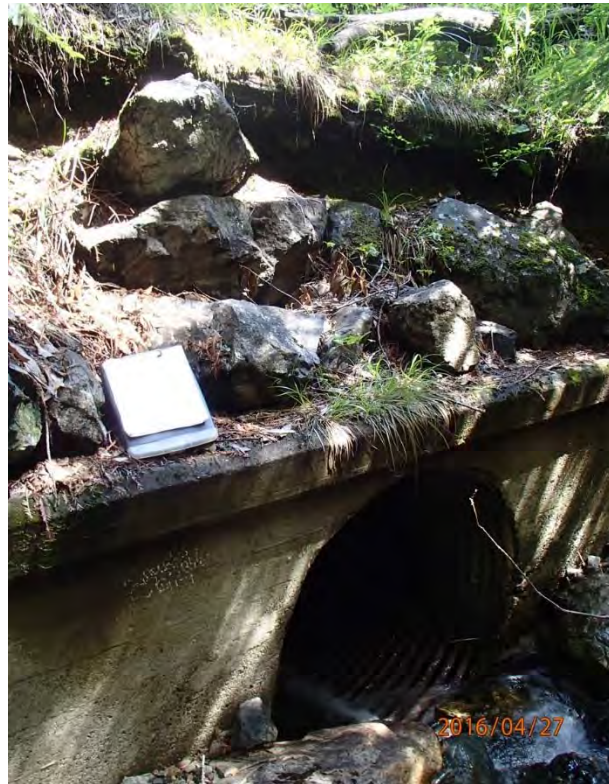
Photos 24 and 25. Photos taken from upstream looking at the stream crossing inlets at Site #140 (left) and #141 (right). The culvert at Site #141 is undersized; therefore, we recommend installing an overflow pipe and excavating material between Sites #140 and #141 for additional protection against diversion.
