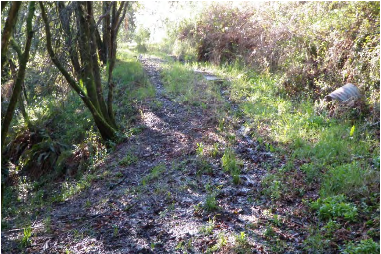
Photo 36. Photo taken of DRC Site #202. A 400' streamside road with an incised IBD drains to 10" rusted DRC. This delivers directly to the nearby channel.
