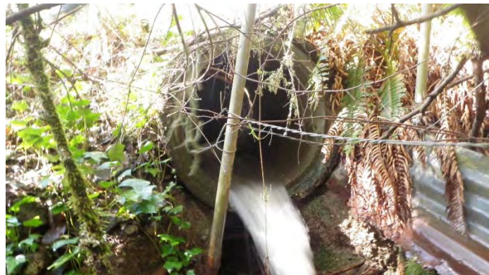
Photos 32 and 33. Photos taken of stream crossing Site #200. Stream valley has been filled and altered by both ancient debris fan deposits as well as mechanical disturbance. A debris trash rack has been installed above the 30” concrete culvert inlet (left) in an attempt to reduce plugging potential. Outlet seen in the photo above.
