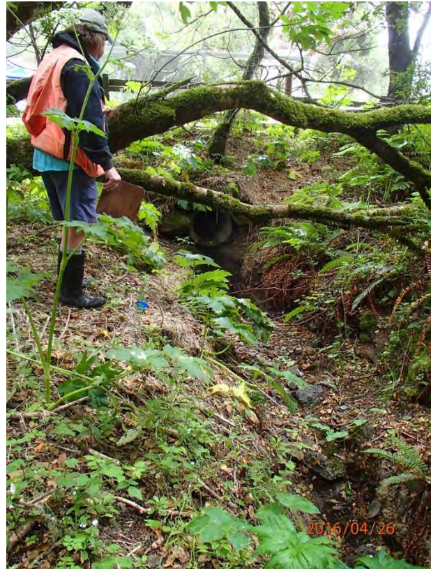
Photos 12 and 13. Photos taken at complicated stream crossing Site #94. Photo 12 (left) is taken from the inlet of the uppermost culvert looking upstream. The stream is carried through an undersized 24” diameter culvert from this point where the stream valley becomes buried by buildings, parking lot, and Muir Woods Road. The 24” culvert regularly plugs and flows across pavement and through a DRC. Flows from the 24” culvert are plumbed into an 18” culvert which outlets into Redwood Creek. Photo 13 (right) is taken below the outlet of the undersized 18” culvert delivering to Redwood Creek.
