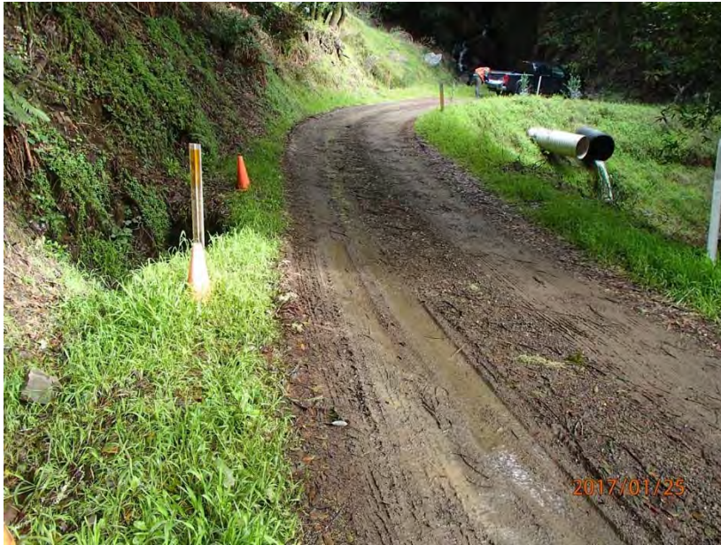
Photos 49 and 50. Photos taken of DRC Site #184. An 18” diameter DRC drains the connected right road approach and springy cutbank (left). The DRC is 30% plugged and is installed at a shallow grade, and the outlet is shot-gunned with a 5’ drop at the outlet (below).
