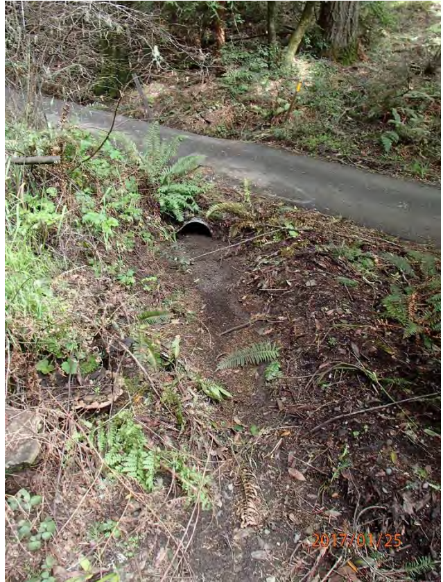
Photos 10 and 11. Photos taken at DRC Site #93. Photo above on left is taken from above the inlet of the 12" DRC. Photo to the right is taken below the outlet of the 12" culvert showing half plugged culvert.
