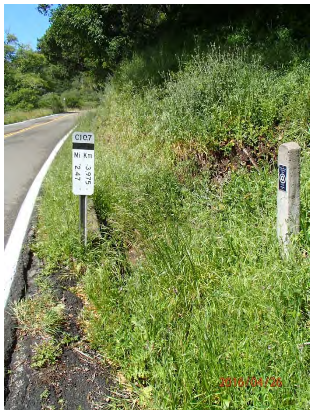
Photos 14 and 15. Photos taken of the hydrologically connected road and inboard ditch draining to stream crossing inlet at Site #159. Note that ditches are well vegetated, which promotes filtration of road surface runoff (sediment and pollutants).
