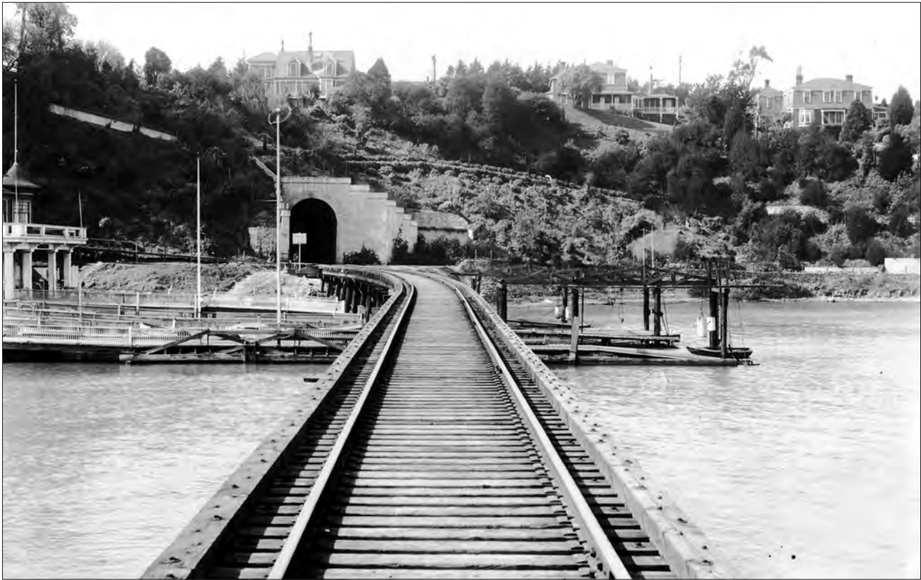
Figure 3.82. The East Waterfront area served utilitarian functions during the period of significance. Here, the Black Point Cove railroad trestle carried trains along the waterfront below Upper Fort Mason. View looking west, 1918 (NPS, San Francisco Maritime National Historical Park Archives).
