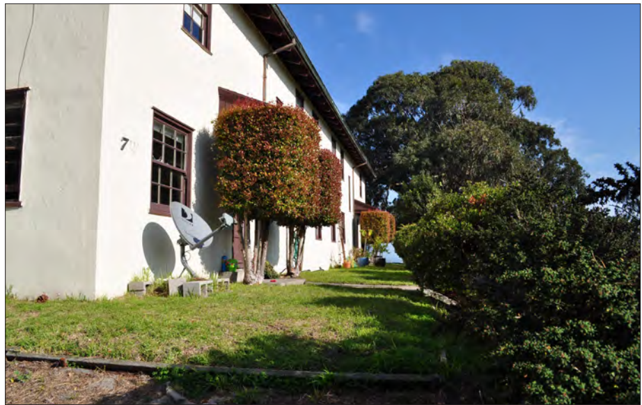
Figure 3.24. Foundation plantings along the south side of Quarters 7 to be rehabilitated. View looking east, 2012 (OCLP).
