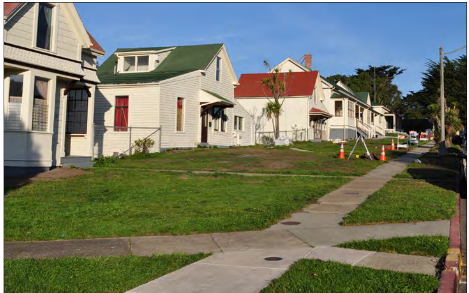
Figure 3.57. Historic walks to be retained or replaced in-kind where required to meet accessibility standards, shown here along Franklin Street. View looking north, 2011 (OCLP).
