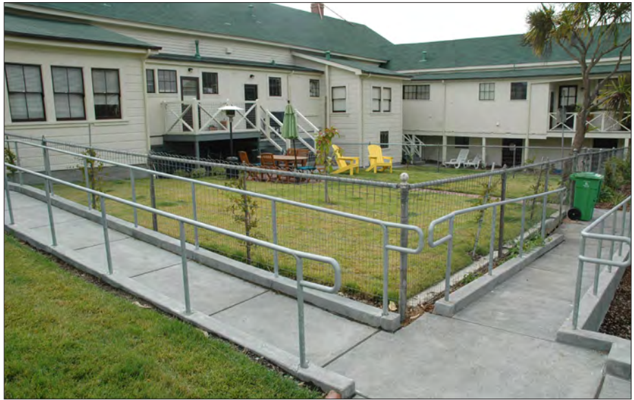
Figure 3.74. Rear of Building 235 shortly following installation of new walks and a new staircase at the building entrance. View looking southeast, 2012 (GGNRA).
