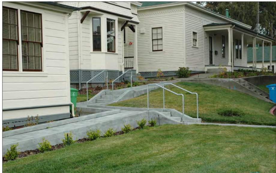
Figure 3.72. Accessible walks to the north and east of Building 235 now accommodate universal building access from Pope Road. View looking northwest, 2012 (GGNRA).
