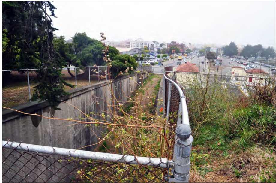
Figure 3.100. Chain-link fence above the railroad tunnel at the western edge of the Great Meadow to be raised to meet life-safety codes and replaced with vinyl coated black chain-link. View looking west, 2011 (OCLP).
