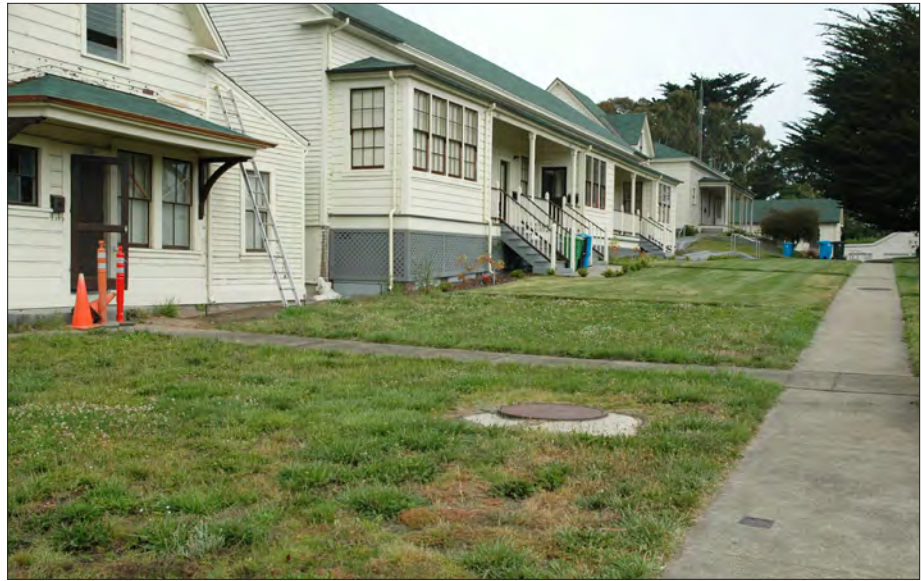
Figure 3.59. Missing foundation plantings to be reestablished along the east facades of all NCO Quarters, including Building 234, shown here at far left. View looking northwest, 2012 (GGNRA).
