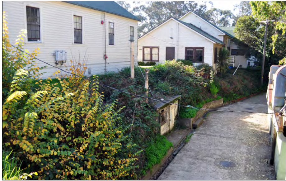
Figure 3.36. Existing view of the proposed location of the preferred alternative Civil War terreplein access ramp to the north of Building 241. Removal of invasive blackberries will reveal an embankment. View looking west, 2012 (OCLP).
