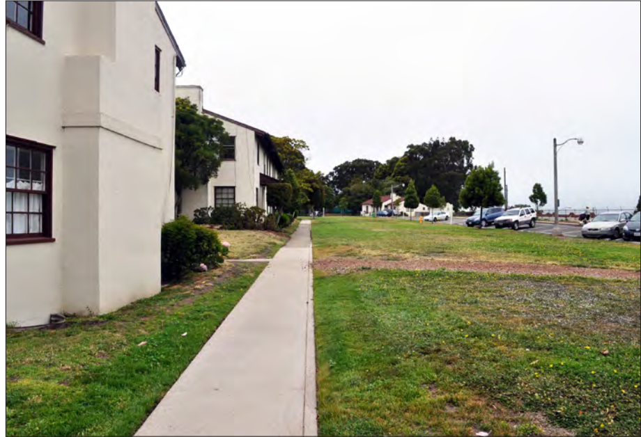
Figure 3.119. Missing street tree planting along MacArthur Avenue adjacent to the Quad buildings. View looking north, 2011 (OCLP).
