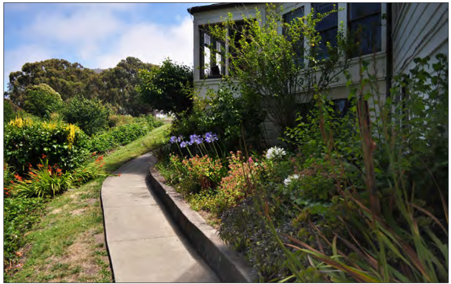
Figure 3.18. Foundation plantings along the east side of Quarters 3 to be retained and maintained. View looking south, 2011 (OCLP).
