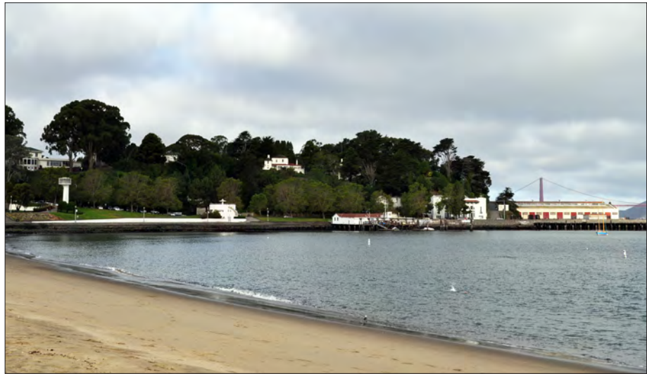
Figure 3.3. East Black Point slope from San Francisco Maritime National Historical Park showing mature trees that now block views to and from the Officers' Quarters. View looking west, 2011 (OCLP).
