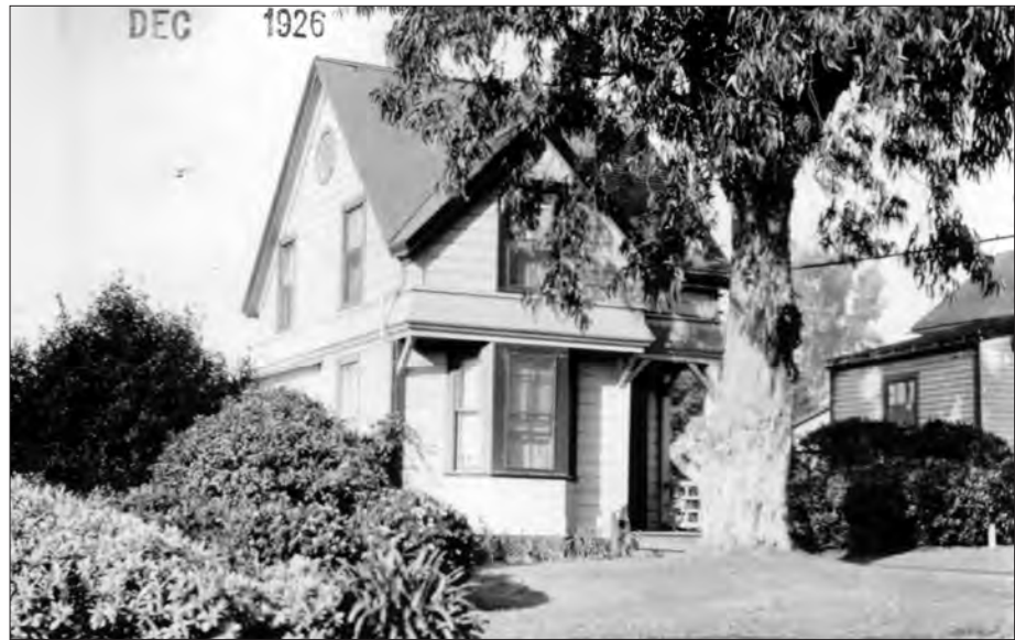
Figure 3.65. Historic blue gum to the east of Building 231 to be replaced in-kind. View looking west, 1926 (National Archives, RG 77, Records of the Construction Division - Annual Construction, Maintenance, and Repair Reports, 1924-1938, Box 135NM).
