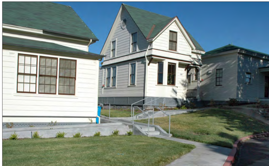
Figure 3.45. Recently reestablished foundation plantings on the grounds of Building 238, shown here shortly following architectural rehabilitation. View looking west, 2012 (GGRNA).
