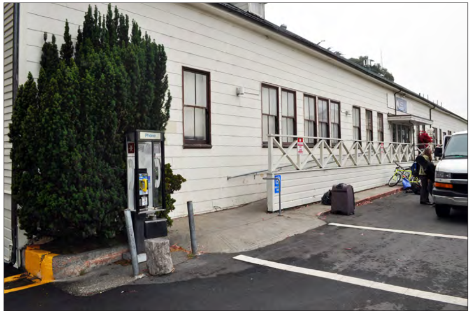
Figure 3.50. The entrance to Building 240 showing the existing narrow sidewalk and steep curb cut to be widened to accommodate universal access. View looking northeast, 2011 (OCLP).
