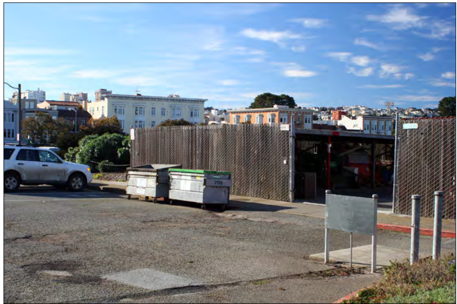
Figure 3.108. The entrance to the maintenance yard opposite Buildings 101 and 102 to be reconfigured to minimize its visibility and accommodate two landscape debris dumpsters. View looking southwest, 2011 (OCLP).
