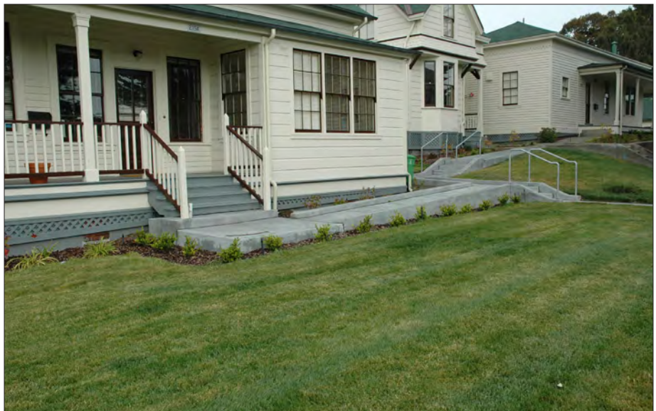
Figure 3.76. Foundation plantings recently reestablished along the east side of Building 235. View looking northeast, 2012 (GGNRA).
