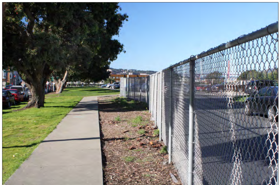
Figure 3.123. Bay Street sidewalk showing the galvanized chain-link fence between Officers' Park and Bay Street to be removed. View looking west, 2011 (OCLP).
