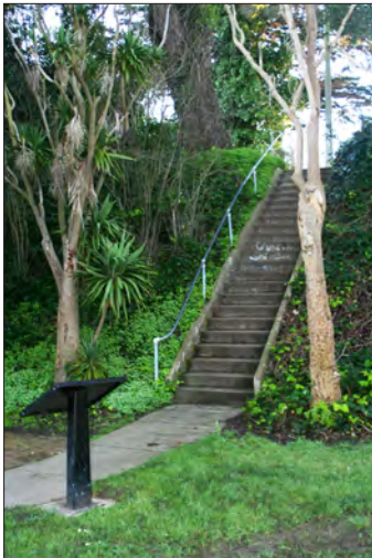
Figure 3.33. Steep staircase leading from Battery Burnham to the Civil War era fortifications to be reconfigured to meet life-safety codes. Note the mature twin cordylines flanking the staircase. View looking south, 2011 (OCLP).
