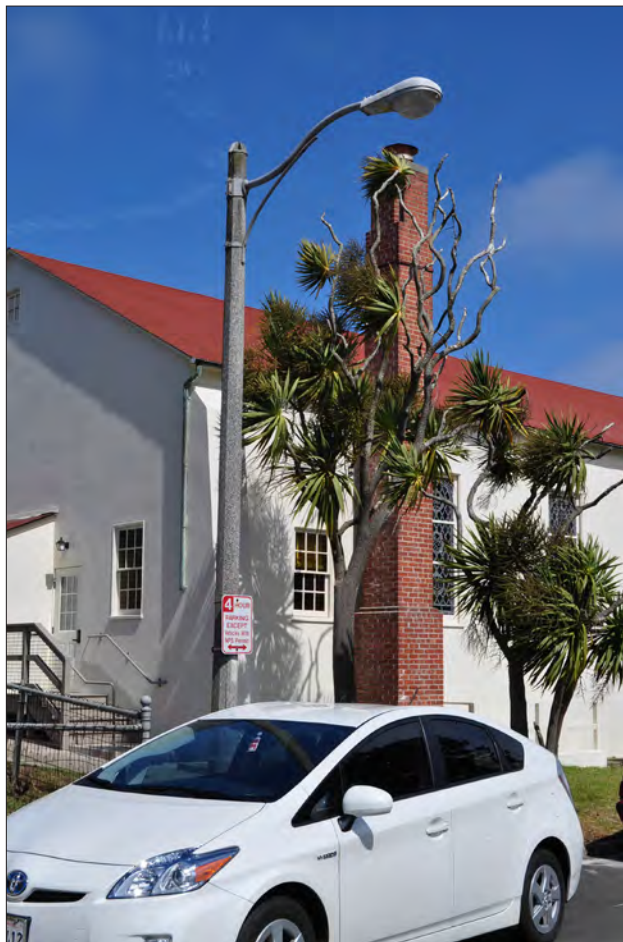
Figure 3.62. Cast-concrete pole light to the west of the Chapel along Pope Road to be retained. View looking southeast, 2011 (OCLP).
