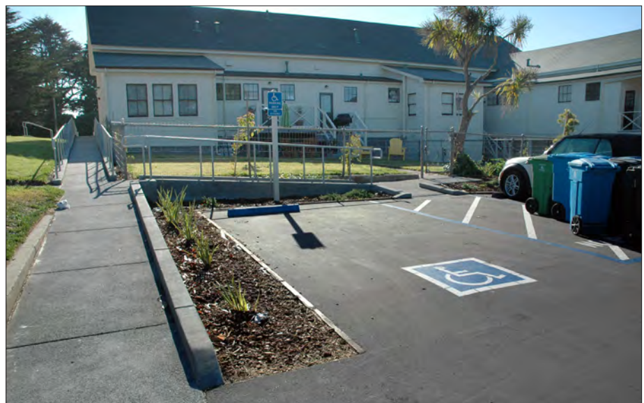
Figure 3.58. Parking area to the west of Building 235 shortly following reconfiguration to accommodate universal access. View looking east, 2012 (GGNRA).
