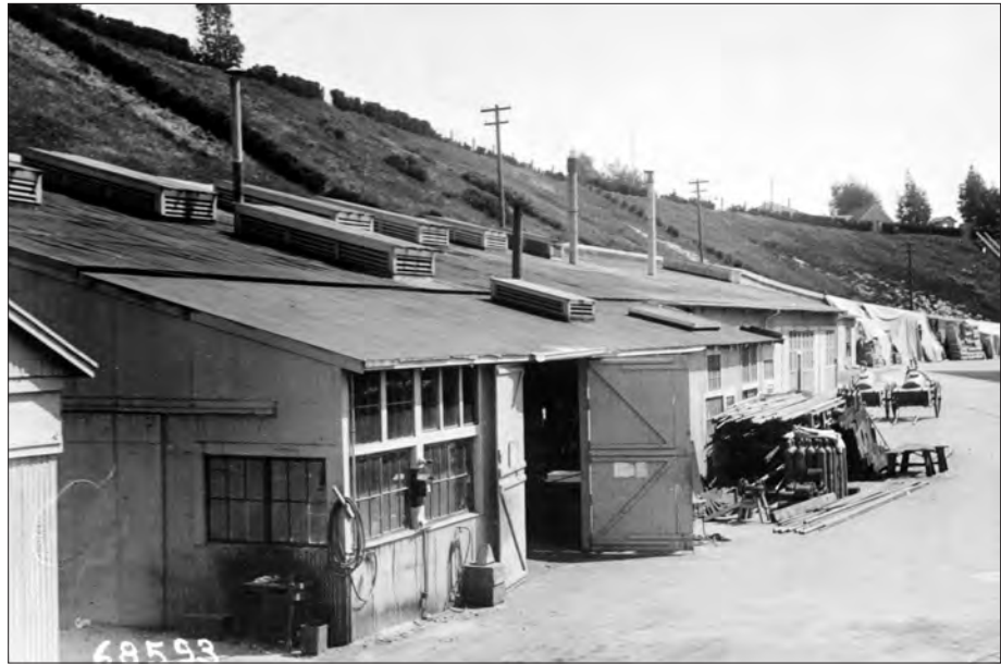
Figure 3.86. The Northwest Embankment from Lower Fort Mason showing the young Monterey cypress windbreak that characterized the slope during the period of significance. View looking south, 1922 (National Archives RG 77, Office of the Chief of Engineers, Construction Completion Reports E 393, Box 139, April 19, 1922).
