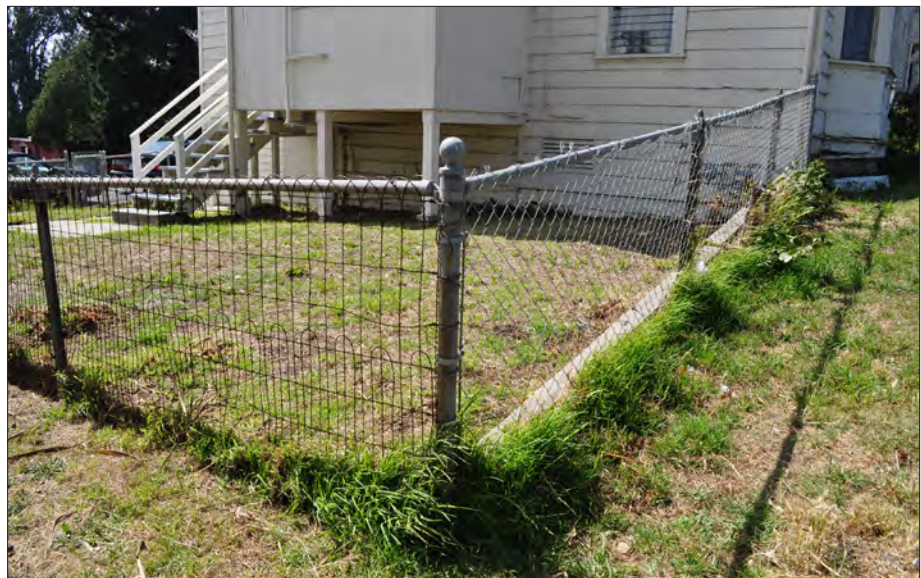
Figure 3.61. Historic woven wire fence to be retained to the south of Building 231 and non-historic chain-link fence to be replaced with historic fence material. View looking northwest, 2011 (OCLP).
