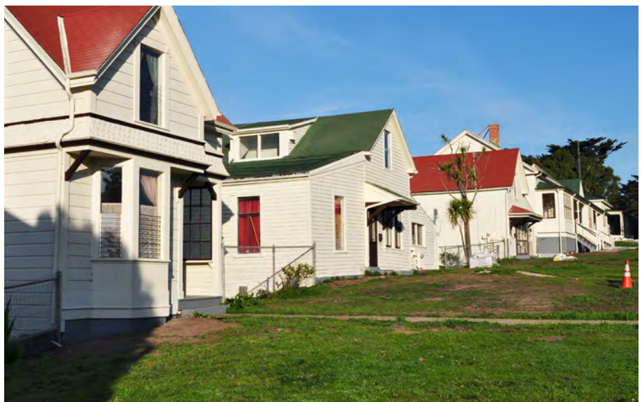
Figure 3.70. Missing foundation plantings to the east of Building 232 (green roof at center) to be reestablished to reflect their historic appearance. View looking northwest, 2012 (OCLP).
