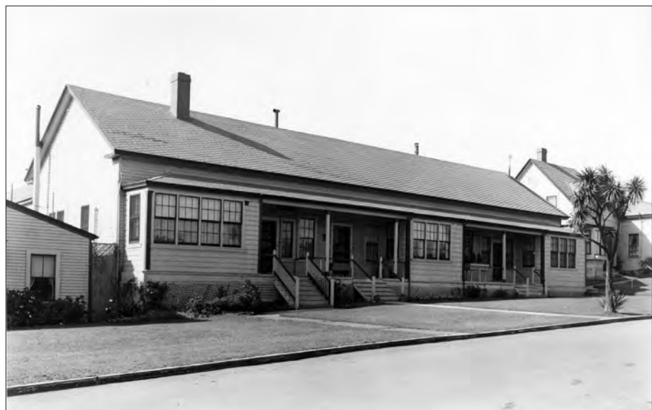
Figure 3.73. Historic view of Building 235 showing the distinctive jog in the south entry walk (left side of photo) to be replaced. View looking northwest, circa 1940 (NPS, GGNRA Archives).
