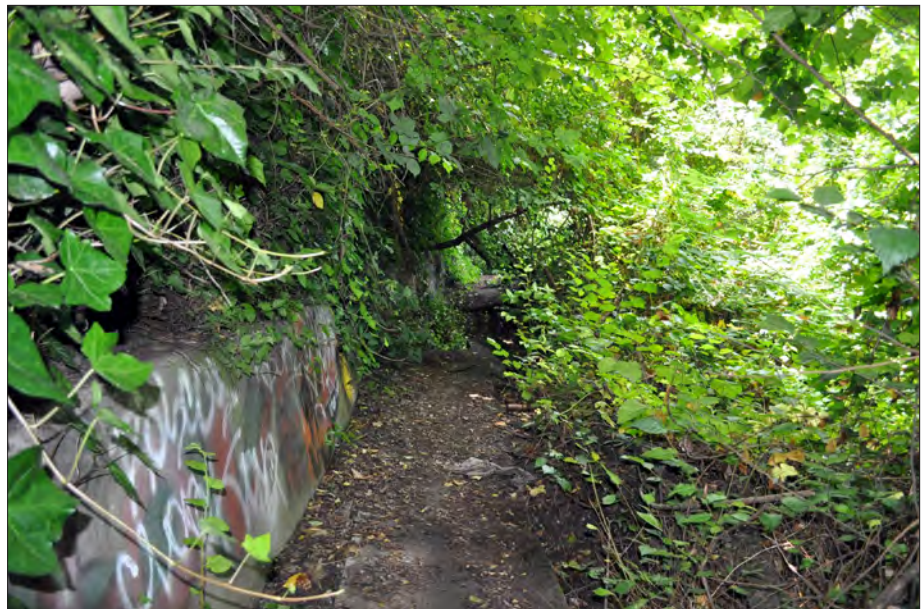
Figure 3.25. Black Point walk adjacent to a graffiti-covered retaining wall showing dark mid-day conditions to be remedied through vegetation management and the installation of security lighting. View looking north, 2011 (OCLP).
