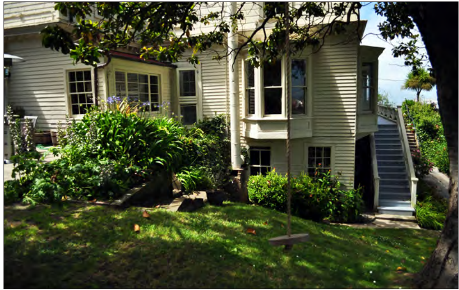
Figure 3.21. Foundation plantings to the south of Quarters 4 to be retained and maintained. View looking north, 2011 (OCLP).
