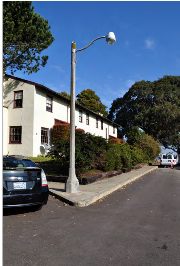
Figure 2.8. Cast-concrete pole light to the south of Quarters 7. View looking east, 2012 (OCLP).
