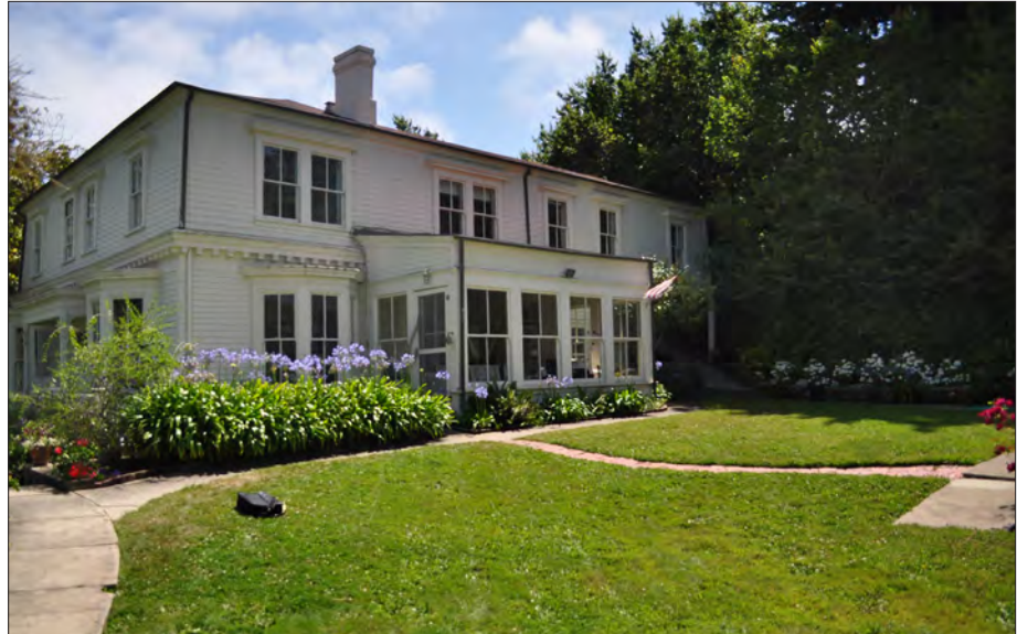
Figure 3.22. Foundation plantings to the north of Quarters 4 to be rehabilitated consistent with access improvements. View looking south, 2011 (OCLP).
