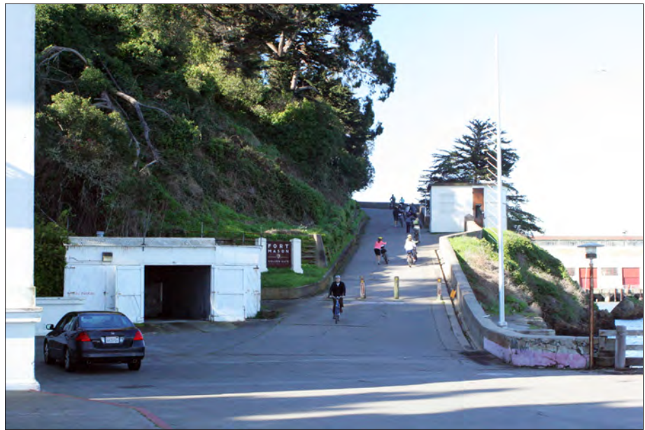
Figure 3.84. Entrance to Upper Fort Mason from the base of McDowell Avenue showing the City Pumping Station garage to be rehabilitated to project a more welcoming appearance. View looking west, 2011 (OCLP).
