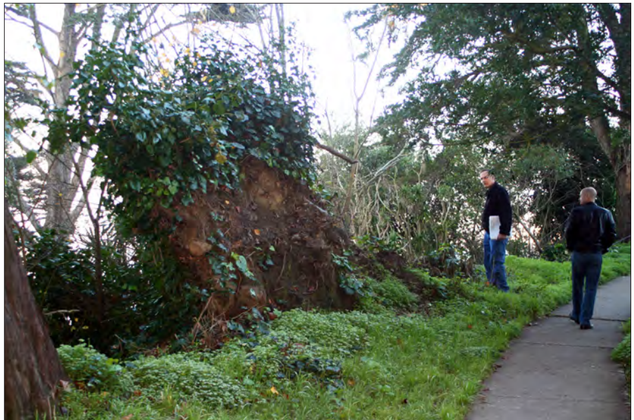
Figure 3.31. An uprooted, wind-fallen tree below Battery Burnham illustrates the potential damage to resources if mature trees are not removed from the earthen terraces. View looking east, 2011 (OCLP).
