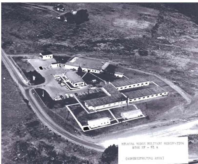
Fig. 6.4: Photograph of the headquarters area at Milagra Ridge.
