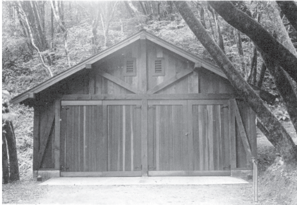
Figure 4.28: The new (lower) garage, completed in May 1931, illustrating exposed timber framing detail. The garage was built on the site of a smaller garage built in 1923. J. Barton Herschler, Muir Woods May 1931 monthly report. National Archives II, College Park, Maryland, RG 79, PI 166, E7, Central Classified Files, 1933-1949, Muir Woods, box 601.
