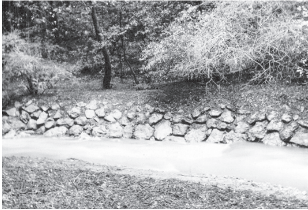
Figure 4.41: Revetment at junction with Fern Creek completed by the spring of 1937, view looking west from main trail. J. Barton Herschler, Muir Woods April 1937 monthly report. National Archives II, College Park, Maryland, RG 79, PI 166, E7, Central Classified Files, 1933-1949, Muir Woods, box 2293.
