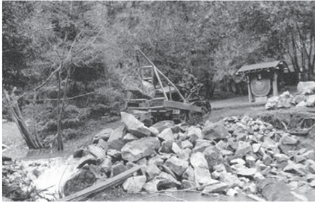
Figure 4.36 (left): View looking northeast across Redwood Creek at stone check dam being built by CWA crews opposite the log cross section, March 1937. J. Barton Herschler, ECW-CWA report, 1934. National Archives II, College Park, Maryland, RG 79, PI 166, E7, Central Classified Files, 1933-1949, Muir Woods, box 2292.
