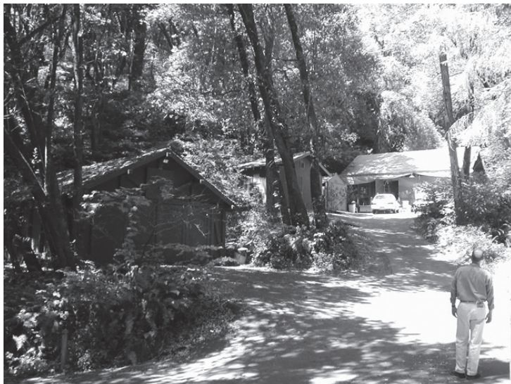
Figure 6.5: View looking northeast in the utility area, showing the 1931 Garage at left, 1934 Equipment Shed (main shop) built by the CCC in the right distance under repair, and newer sheds in middle ground, July 2003. SUNY ESF.
