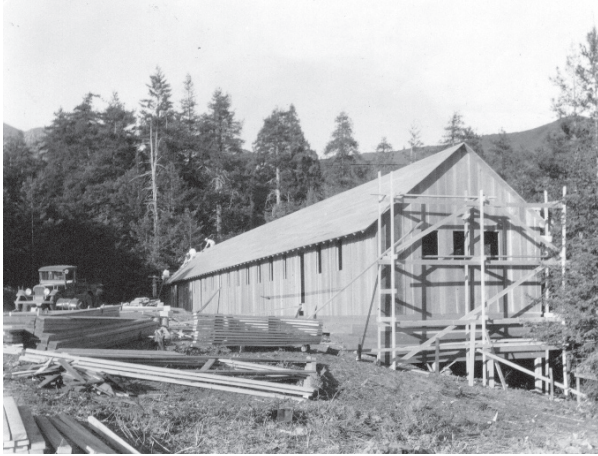
Figure 4.9: The mess hall at the CCC Muir Woods Camp under construction, October 26, 1933, west of site of first Muir Inn. J. Barton Herschler, Emergency Conservation Work (ECW) Monthly Report for October 1933. National Archives II, College Park, Maryland, RG 79, PI 166, E7, Central Classified Files, 1933-1949, Muir Woods, box 2297.
