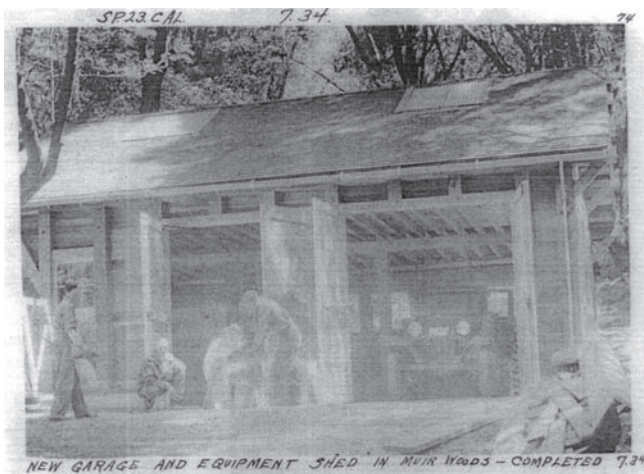
Figure 4.50: The Equipment Shed nearing completion by CCC crews, July 1934. Courtesy Golden Gate National Recreation Area, Park Archives, box 36/6, Muir Woods Collection.
