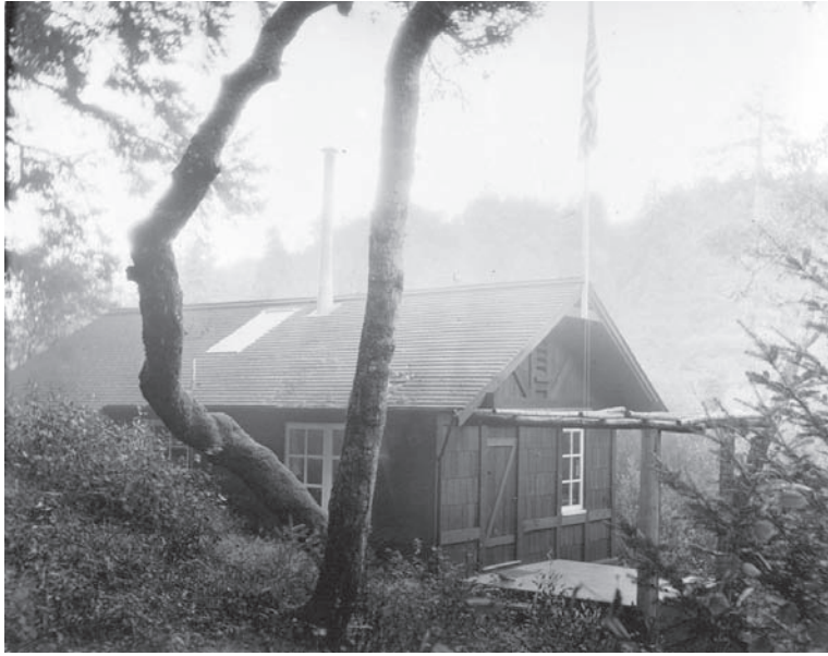
Figure 3.40: The Custodian's Cottage showing original section built in 1922, view looking southwest across lower canyon, October 1934. Courtesy Golden Gate National Recreation Area, Park Archives, GOGA 32470 B36, Muir Woods Collection.
