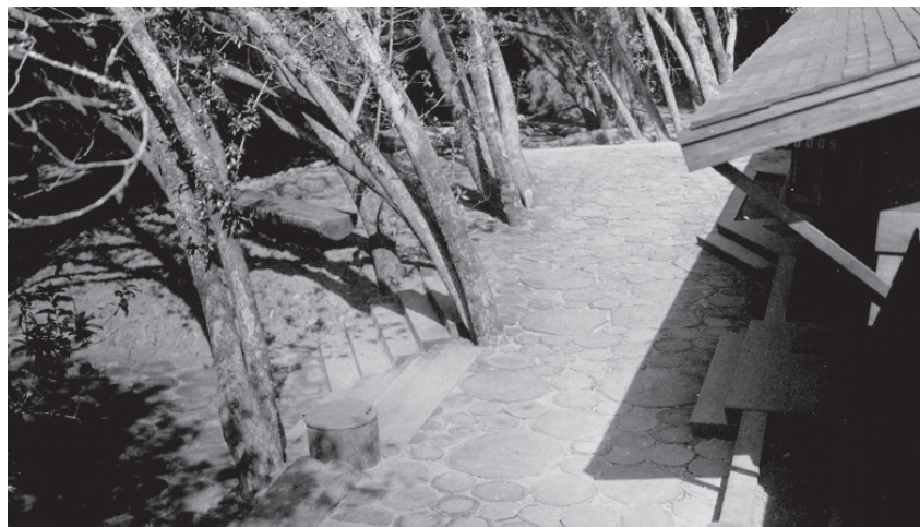
Figure 4.64: The terrace illustrating redwood rounds paving built by CCC Camp Alpine Lake along the south front of the operator wing, April 1941. Walter Finn, April 1941 monthly report. National Archives II, College Park, Maryland, RG 79, PI 166, E7, Central Classified Files, 1933-1949, Muir Woods, box 2293.
