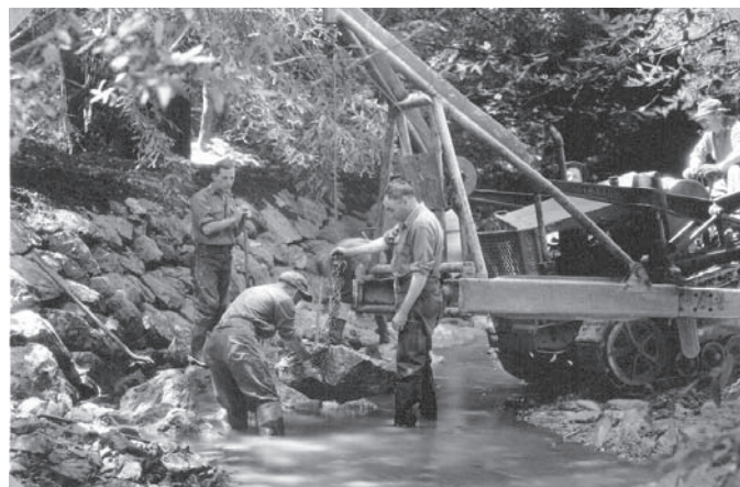
Figure 4.40: CCC crews at work building stone revetments in Redwood Creek, June 1936. Mt. Tamalpais State Park Camp SP-23, June 1936 report. National Archives II, College Park, Maryland, RG 35, Records of the Civilian Conservation Corps, Division of Investigations, Camp Inspection Reports, 1933-42, California, box 10.
