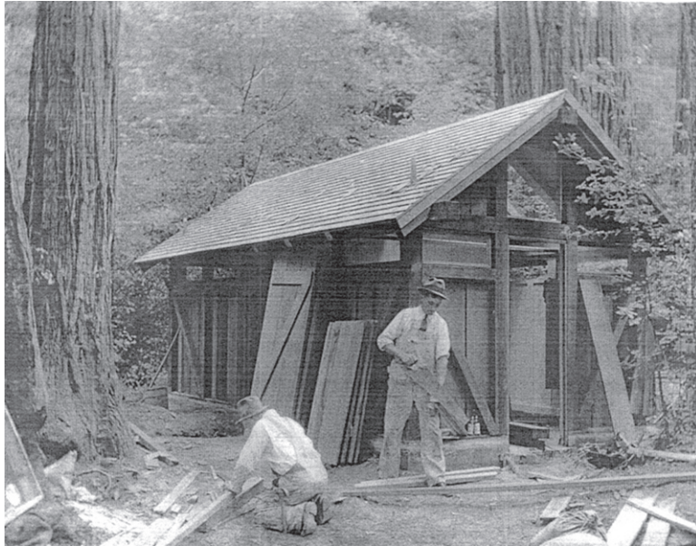
Figure 4.46: The Cathedral Grove comfort station under construction, August 25, 1934. Courtesy Golden Gate National Recreation Area, Park Archives, box 36/6, Muir Woods Collection.
